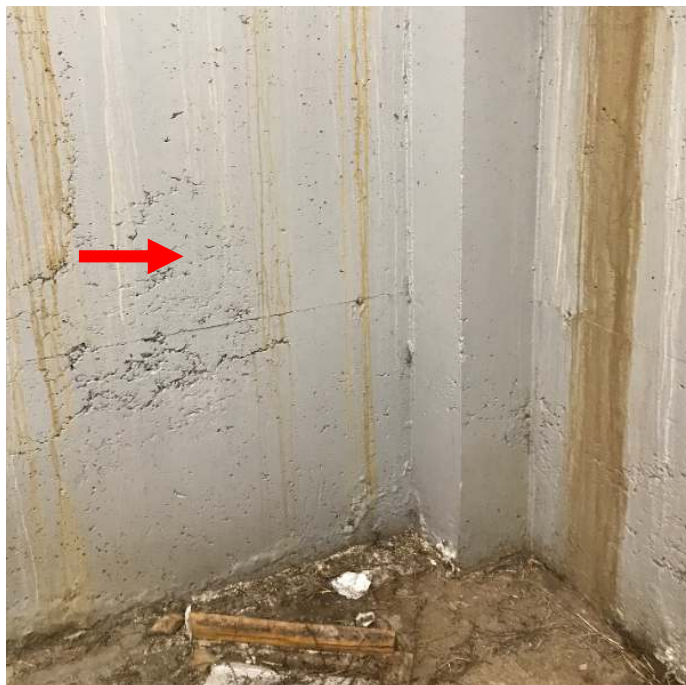
Photo 1. Interior, Mechanical Room Wall: Grey paint was confirmed to contain 20 ppm lead (DST Sample ID 2759-LP01).
