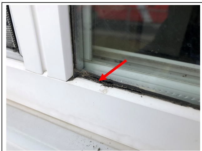
Photo 4: House – Asbestos-containing exterior window glazing compound – back on the exterior laundry room and kitchen windows.
