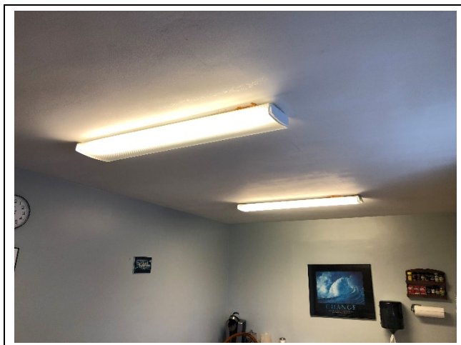
Photo 10: House – Fluorescent light tubes containing mercury vapour in kitchen.
