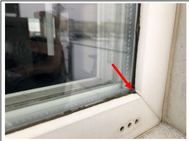
Photo 13: Office Building – Asbestos-containing exterior window glazing – black on exterior windows.
