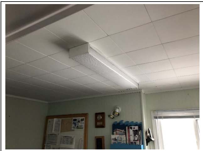
Photo 17: Office Building – Fluorescent light tubes containing mercury vapour in office 1.
