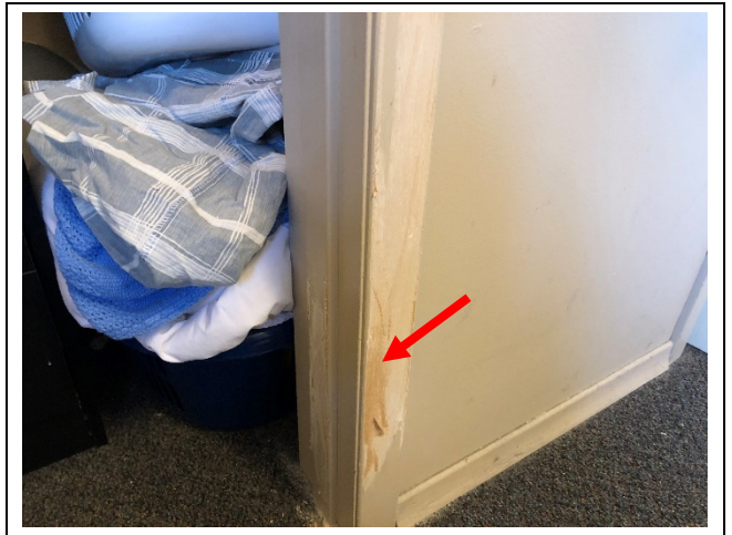
Photo 6: House – Lead-containing white coloured paint on interior wood finishes.
