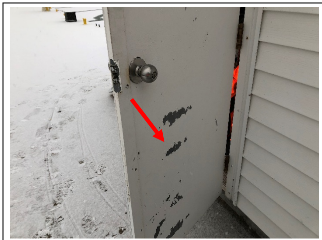
Photo 20: Pier Building – Damaged lead-containing white coloured paint on exterior doors.
