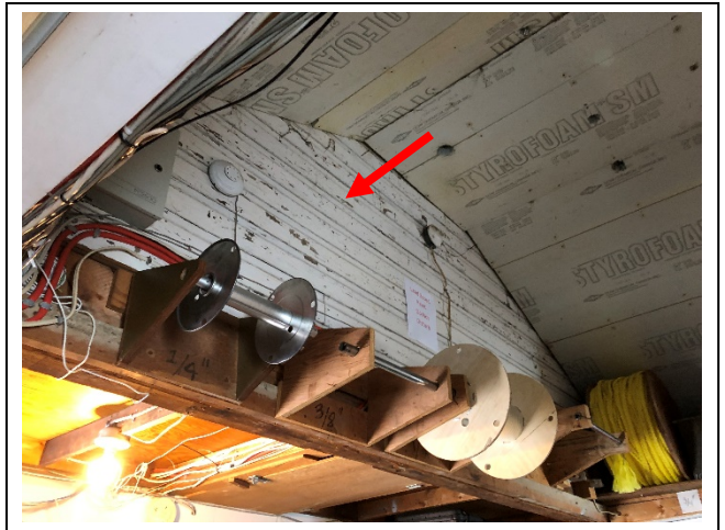
Photo 14: Office Building – Damaged lead-containing white coloured paint on wood siding in the locker room.
