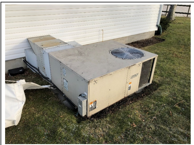
Photo 9: House – Lennox HVAC unit containing R-22 ozone depleting substances on exterior.
