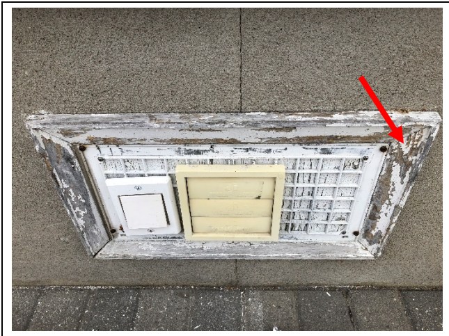
Photo 5: House – Damaged lead-containing white coloured paint on exterior wood finishes.
