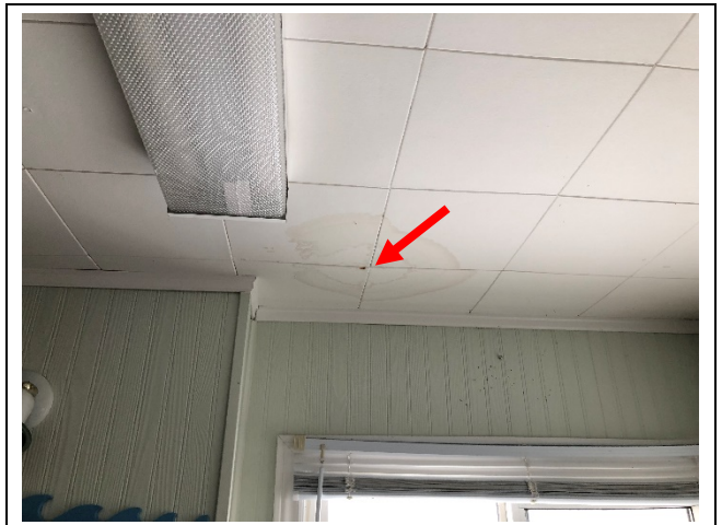
Photo 16: Office Building – Water stained ceiling tiles on office 1 ceiling.
