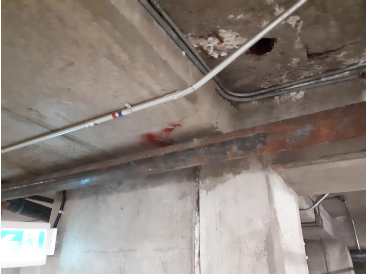
Photo 1. Non-asbestos containing cement parging near former drain pipe.
