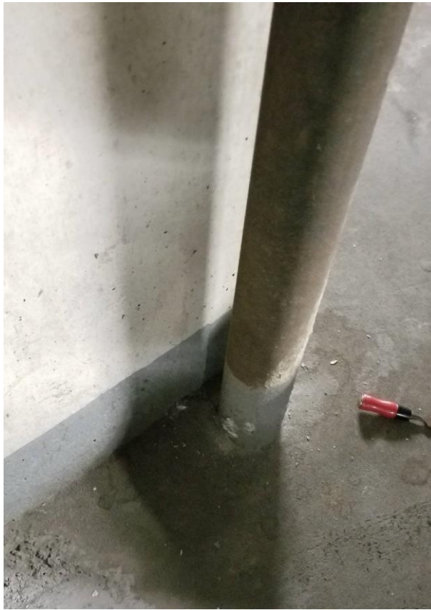
Photo 2. Non-asbestos containing cement compound near a column. Cement compound is troweled on to bottom of pipe.
