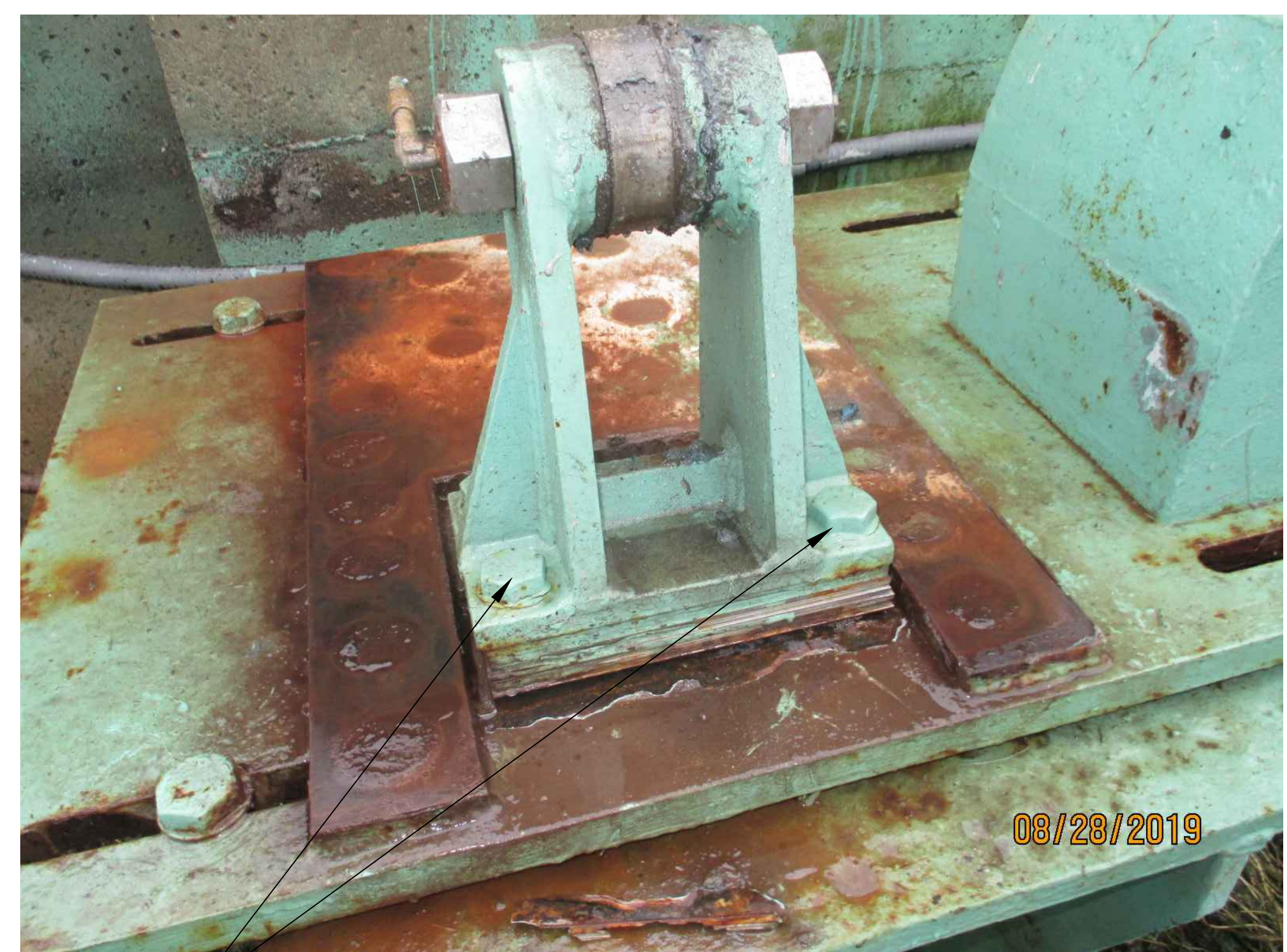
PHOTO OF SOUTH SPAN LOCK RECEIVER
