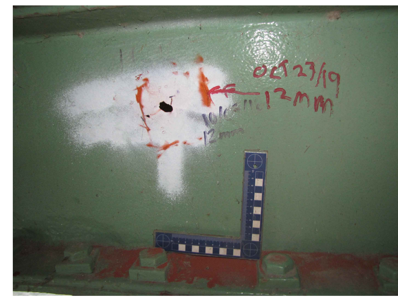
14S-16S NORTH CHANNEL EXISTING CONDITION
