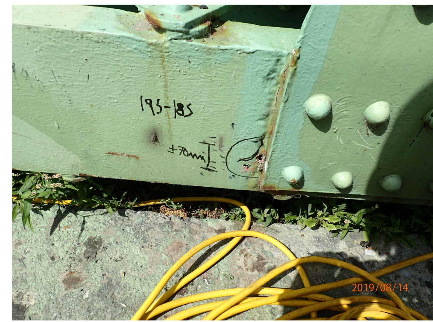
18S-19S - TOWER TRUSS EXISTING CONDITION
