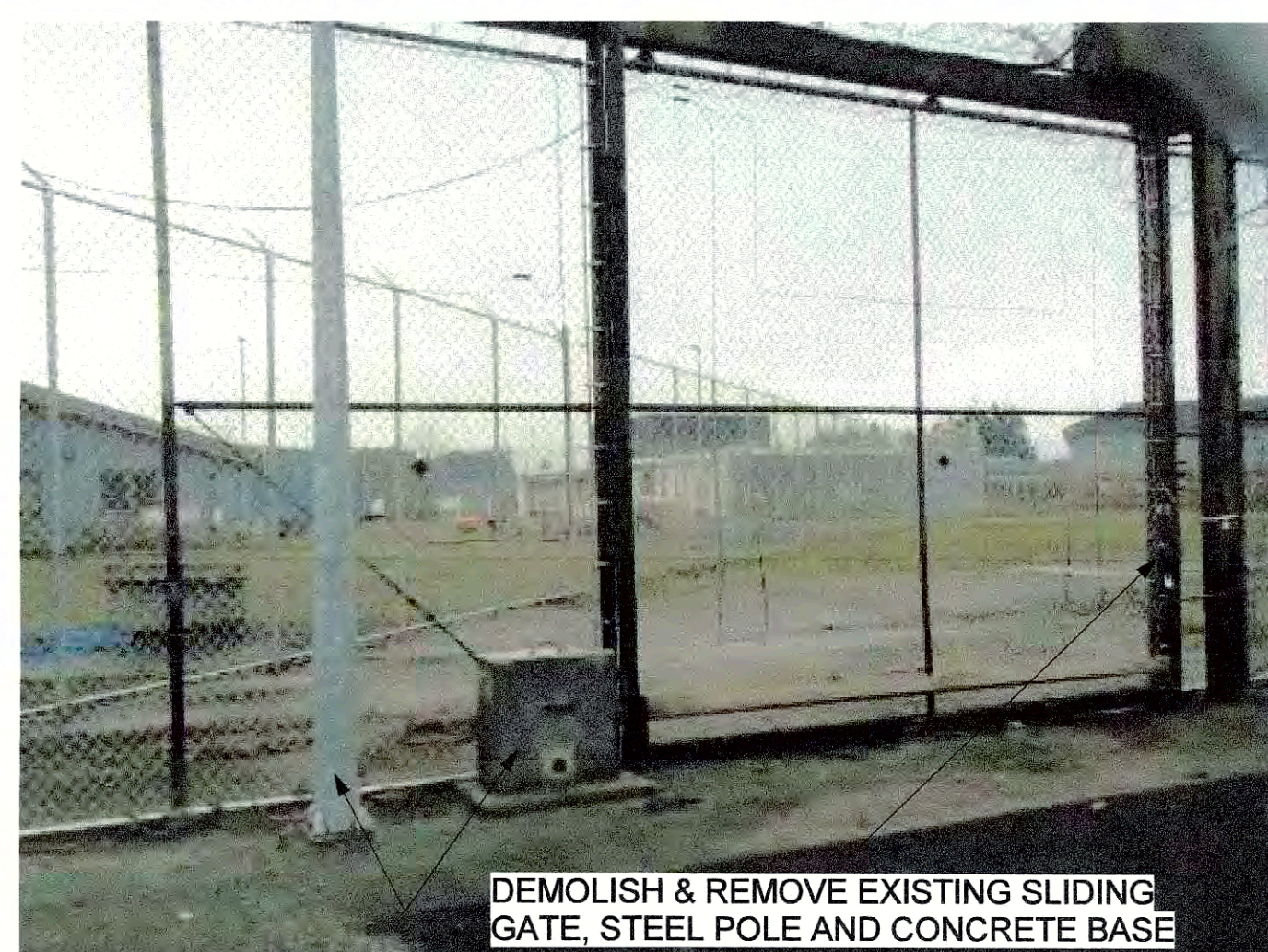
PHOTO F DEMOLISH EXISTING SLIDING GATE 17
