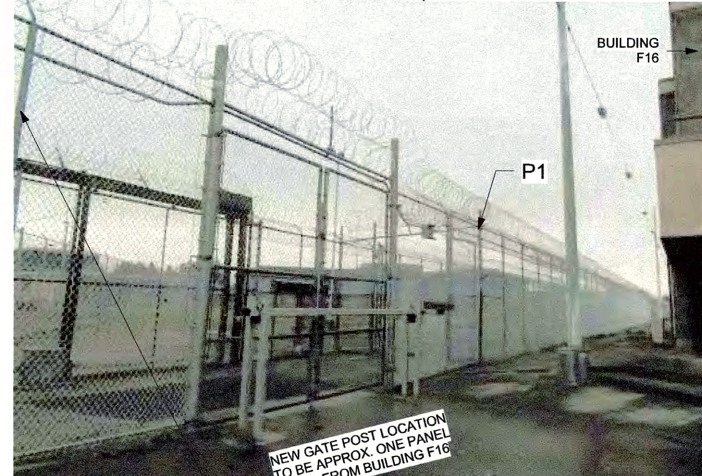
PHOTO C OF EXISTING GATE 18 & CRASH BEAM (OUTER PERIMETER FENCE)
