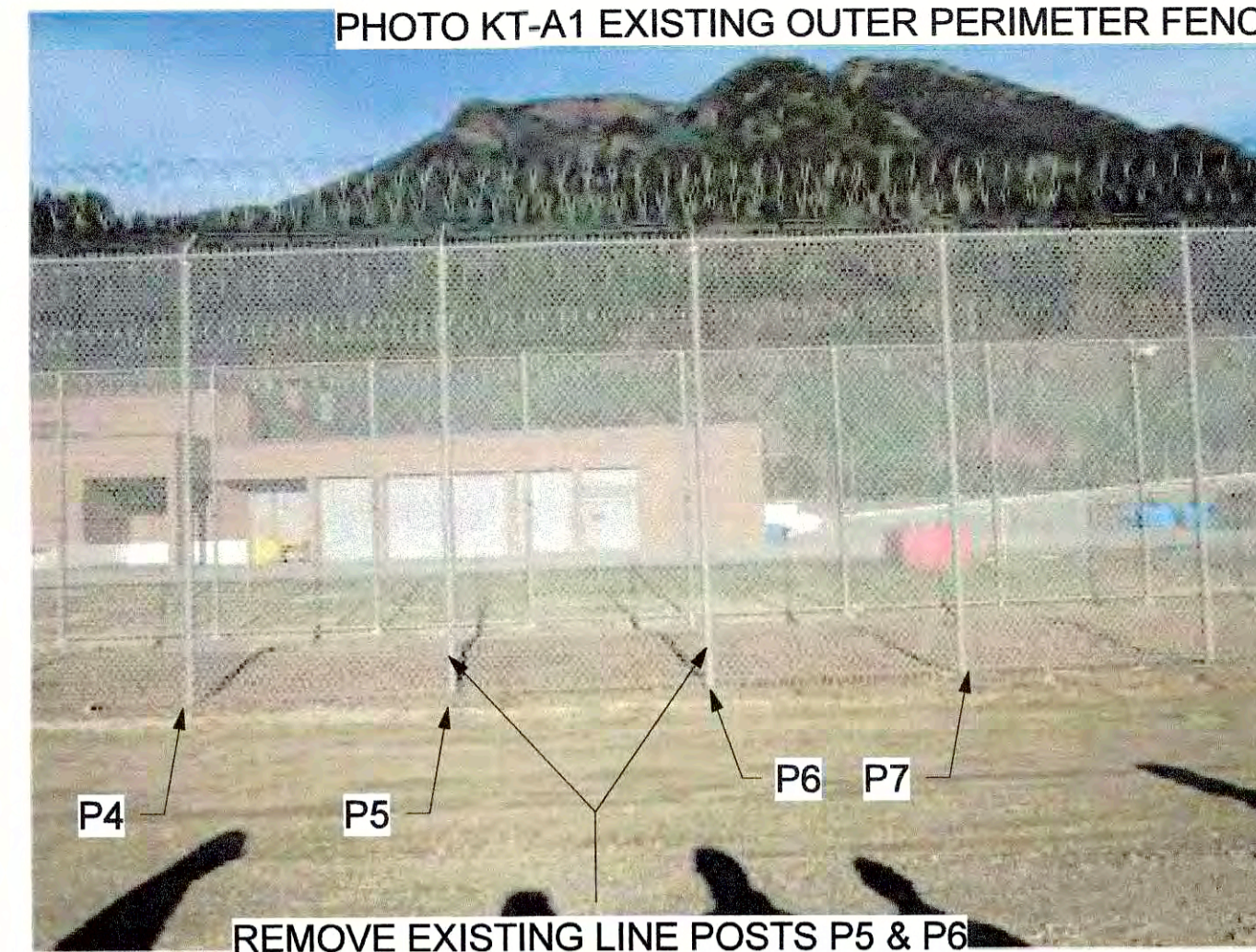
PHOTO KT-A1 EXISTING OUTER PERIMETER FENCE
