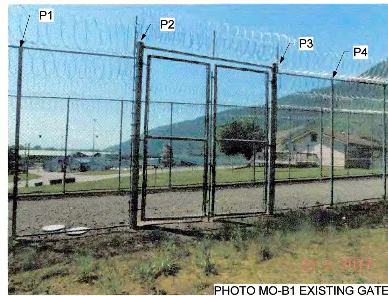
PHOTO MO-B1 EXISTING GATE 8
