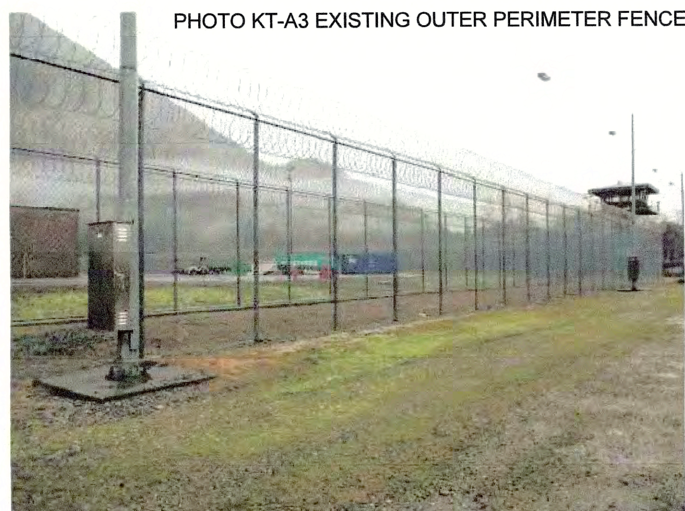
PHOTO KT-A3 EXISTING OUTER PERIMETER FENCE
