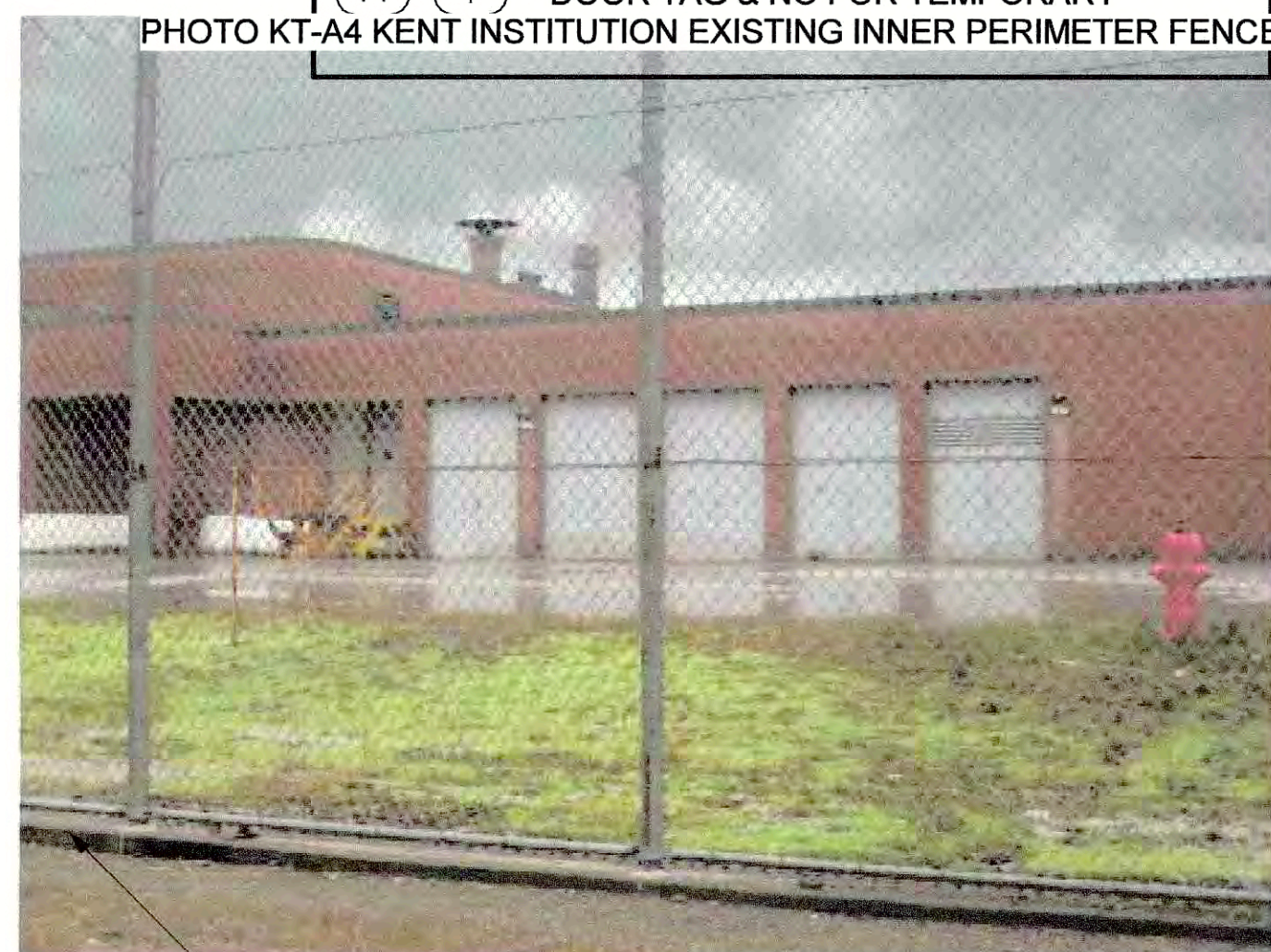
EXISTING ANTI-TUNNELING WALL WITH MIN 900 MM DEPTH AT INNER PERIMETER FENCE (TYP)
