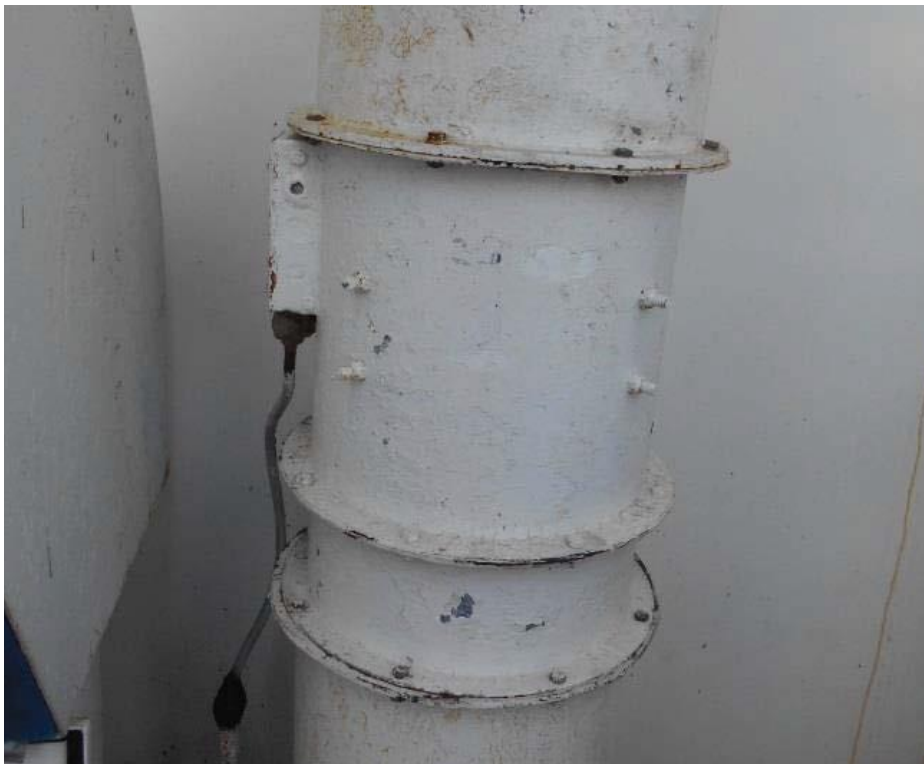
Figure 16.3-8: Photograph of in-situ Galley exhaust axial fan (EF-2), installed on open deck
