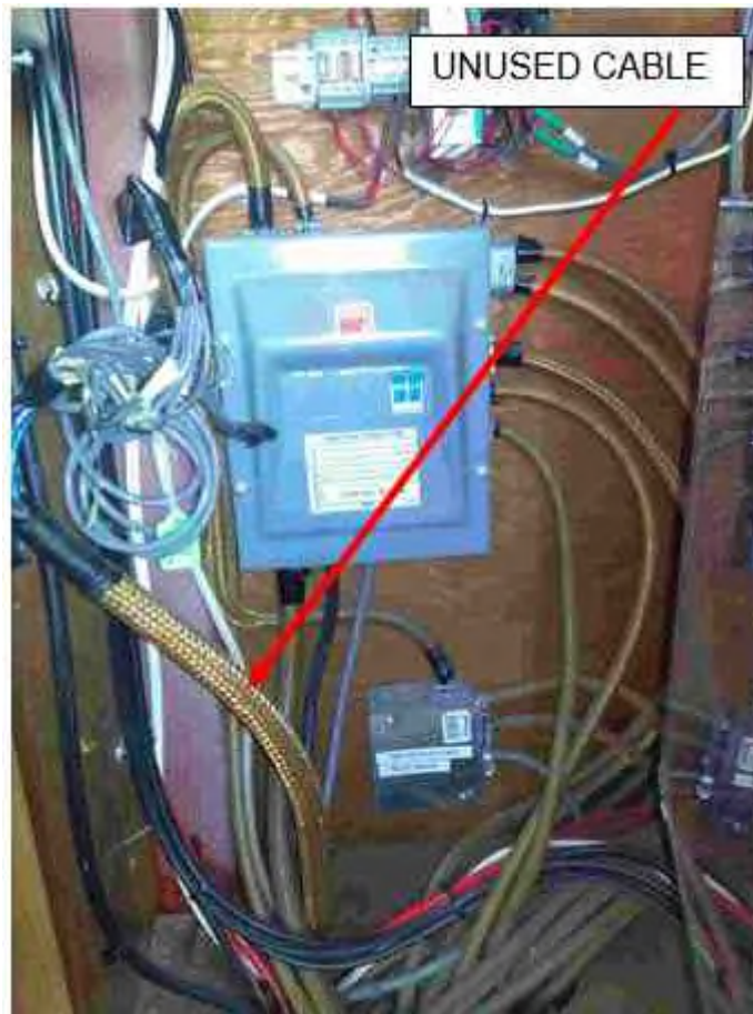
Figure 17.4-18: Cable to remove
