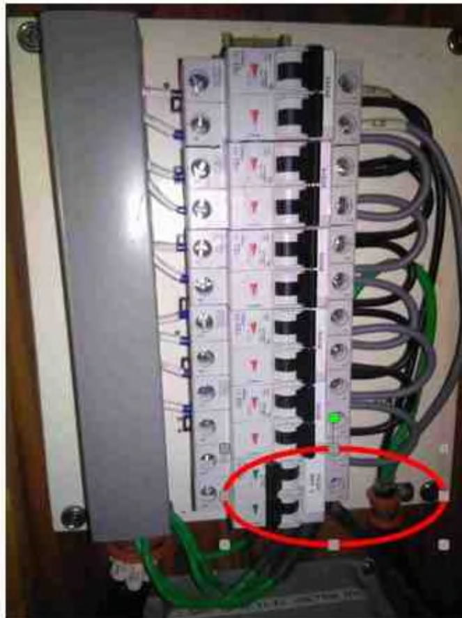
Figure 17.4-26: Radar UPS Breaker
