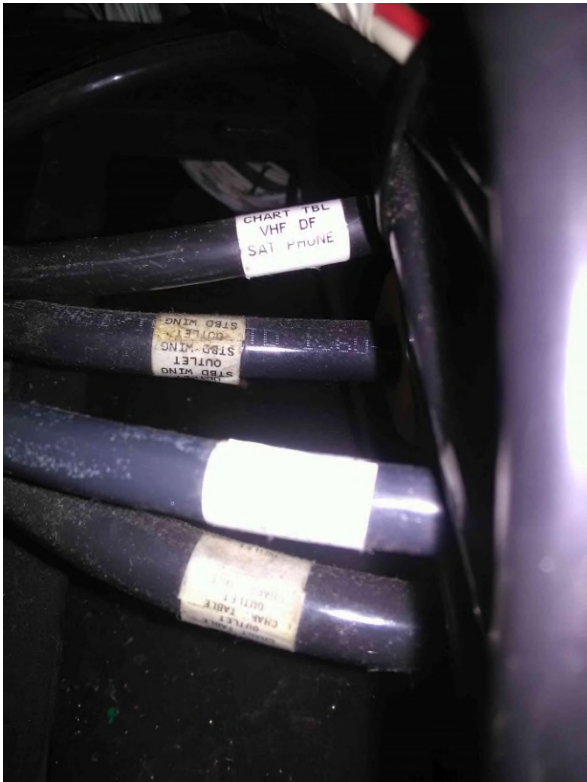
Figure 17.4-13: UPS output cables
