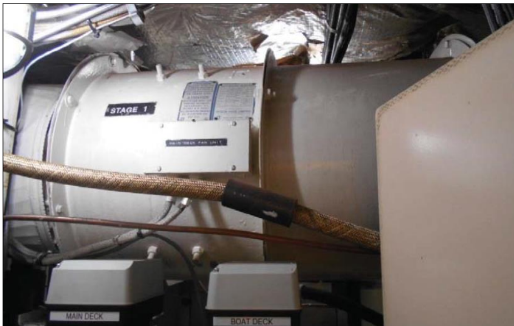
Figure 16.3-4: Photograph of in-situ main deck supply axial fan (SF-3)
