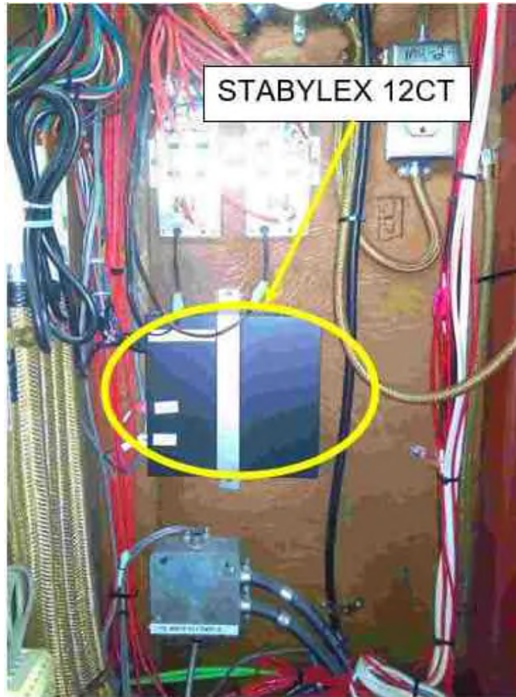
Figure 17.4-1: Stabylex Power Supply Location
