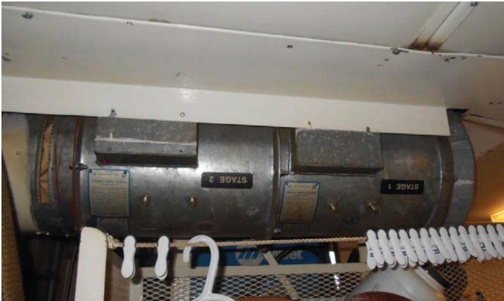
Figure 16.3-9: Photograph of in-situ Deck Workshop supply axial fans (SF-6.1 & SF-6.2)
