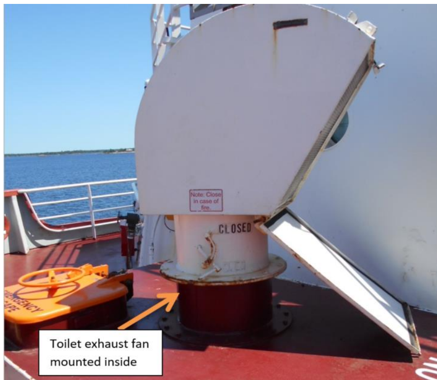
Figure 16.3-11: Photograph of in-situ toilet Exhaust axial fans (EF-4)
