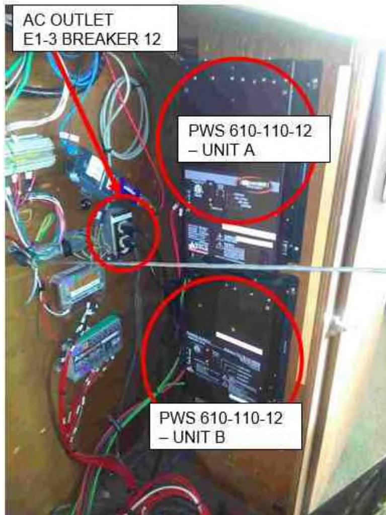
Figure 17.4-16: Current 12V Power supplies location
