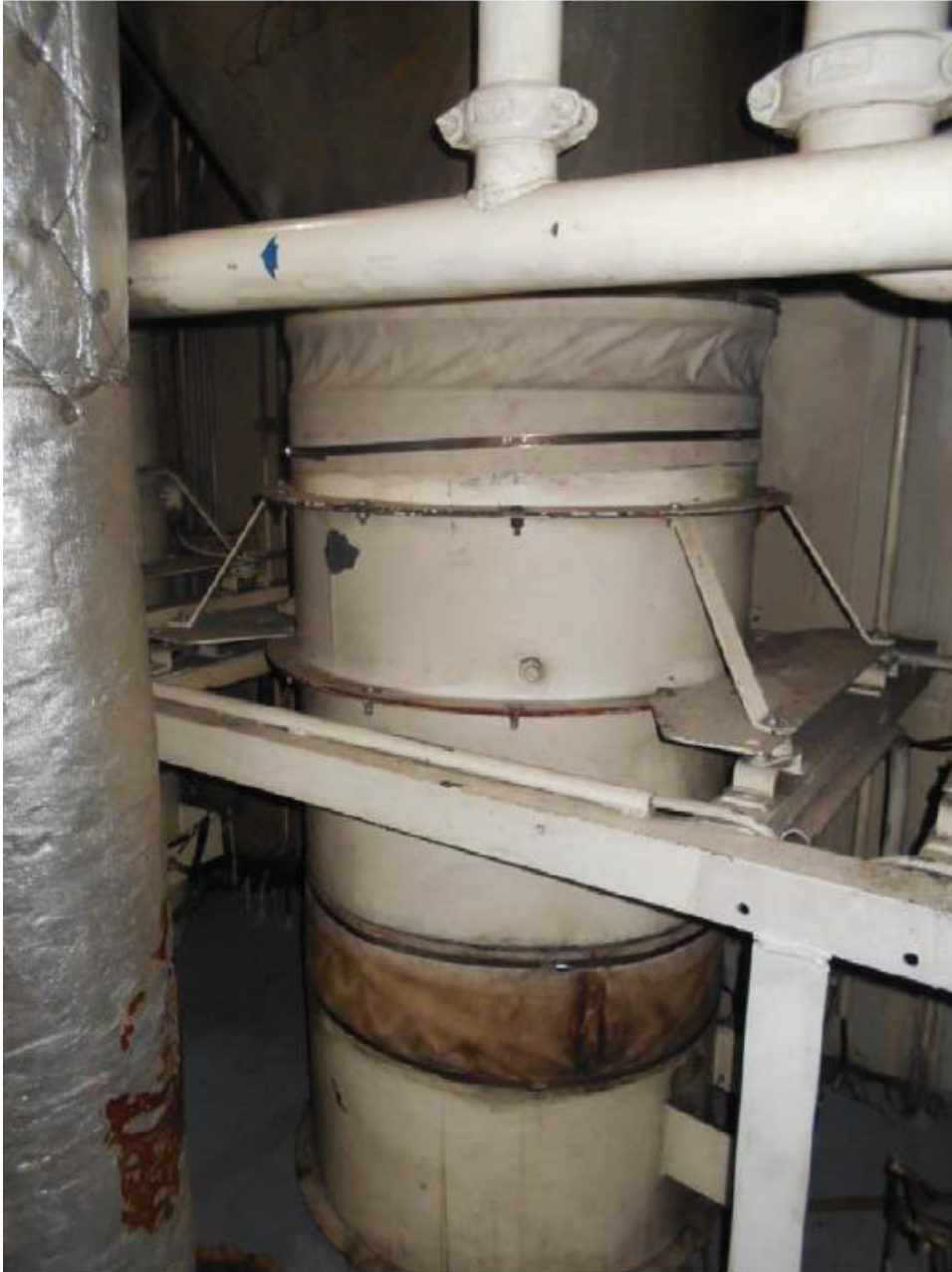
Figure 16.3-1: Photograph of in-situ engine room Supply Fan (SF-7 or SF-8)
