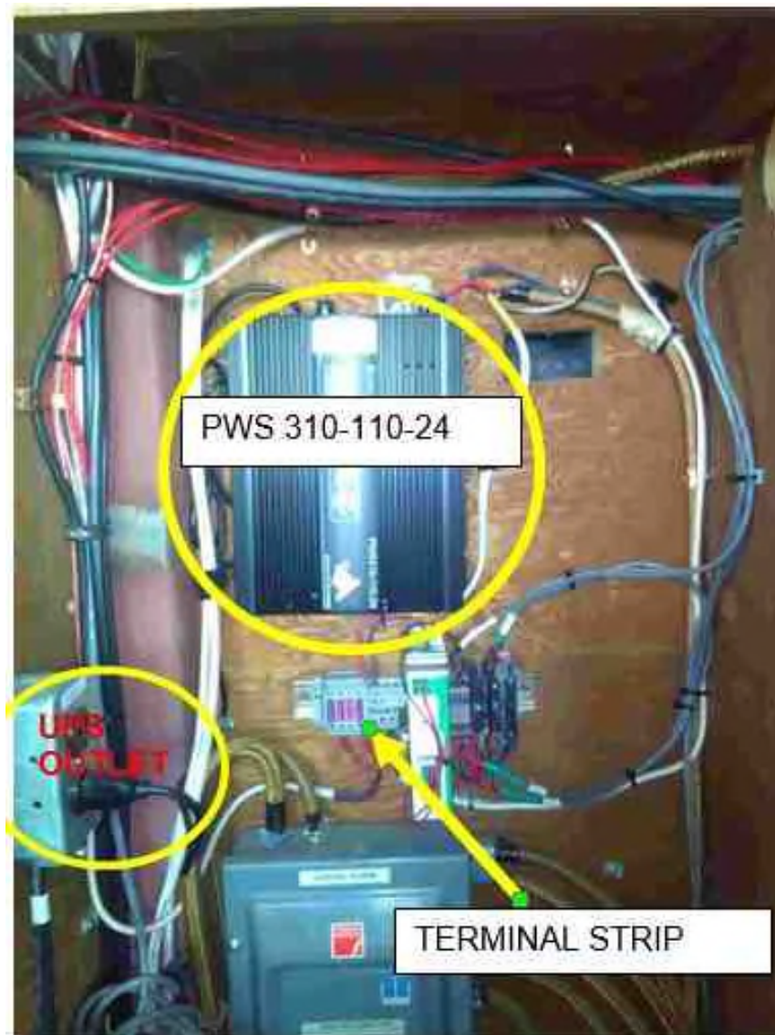
Figure 17.4-4: 24v Power Supply – Chart table
