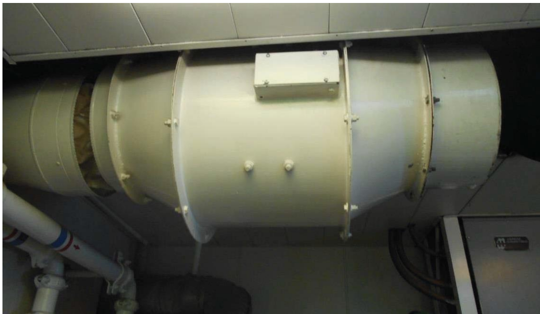
Figure 16.3-6: Photograph of in-situ Emergency Generator supply axial fan (SF-9)
