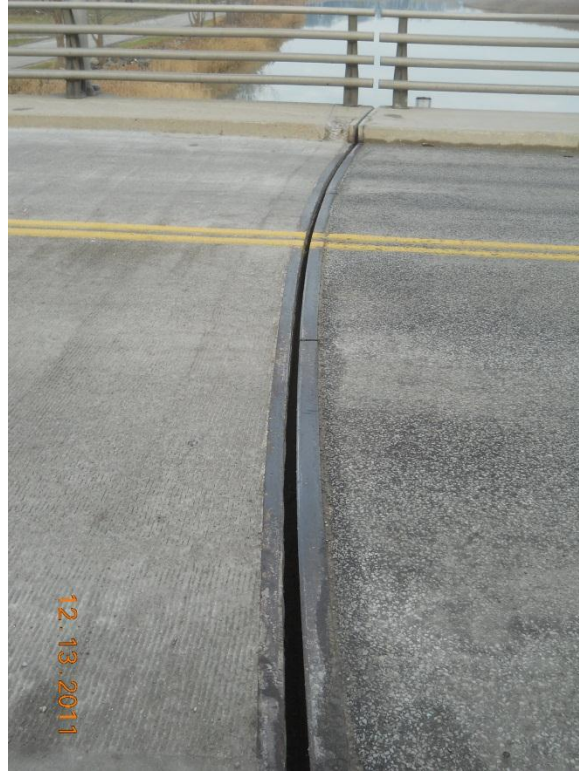
Photograph 33 - West rest pier joint looking north
