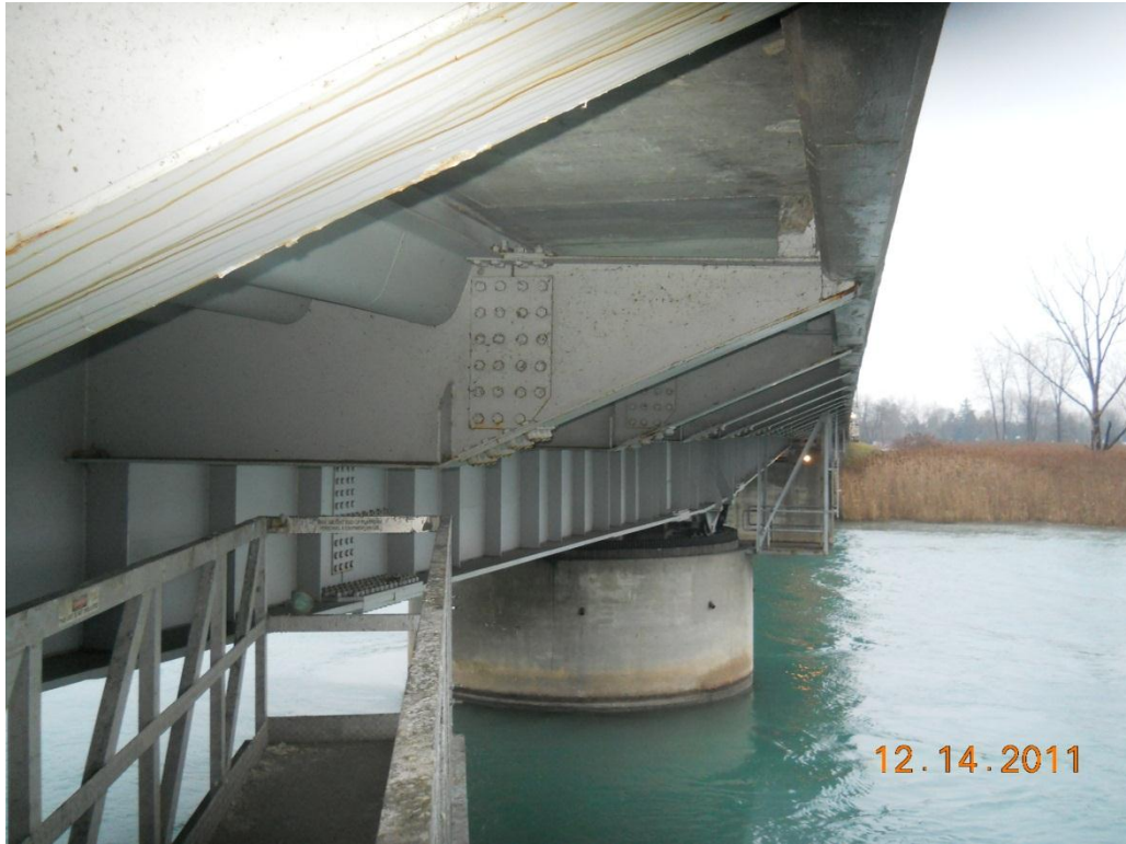
Photograph 111 - Span 3, south exterior soffit looking east
