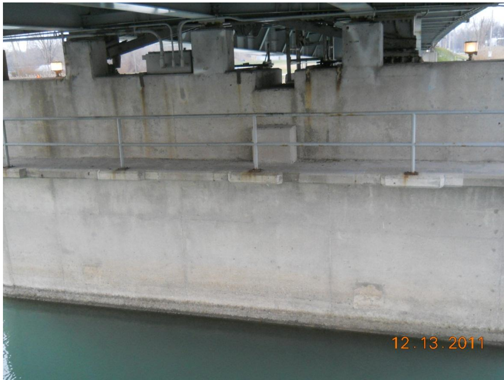
Photograph 54 - East face of east rest pier
