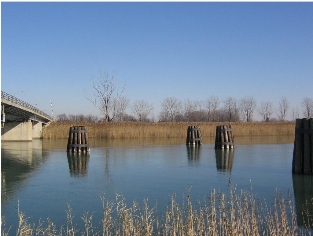
Photograph 138 - Downstream protective dolphins
