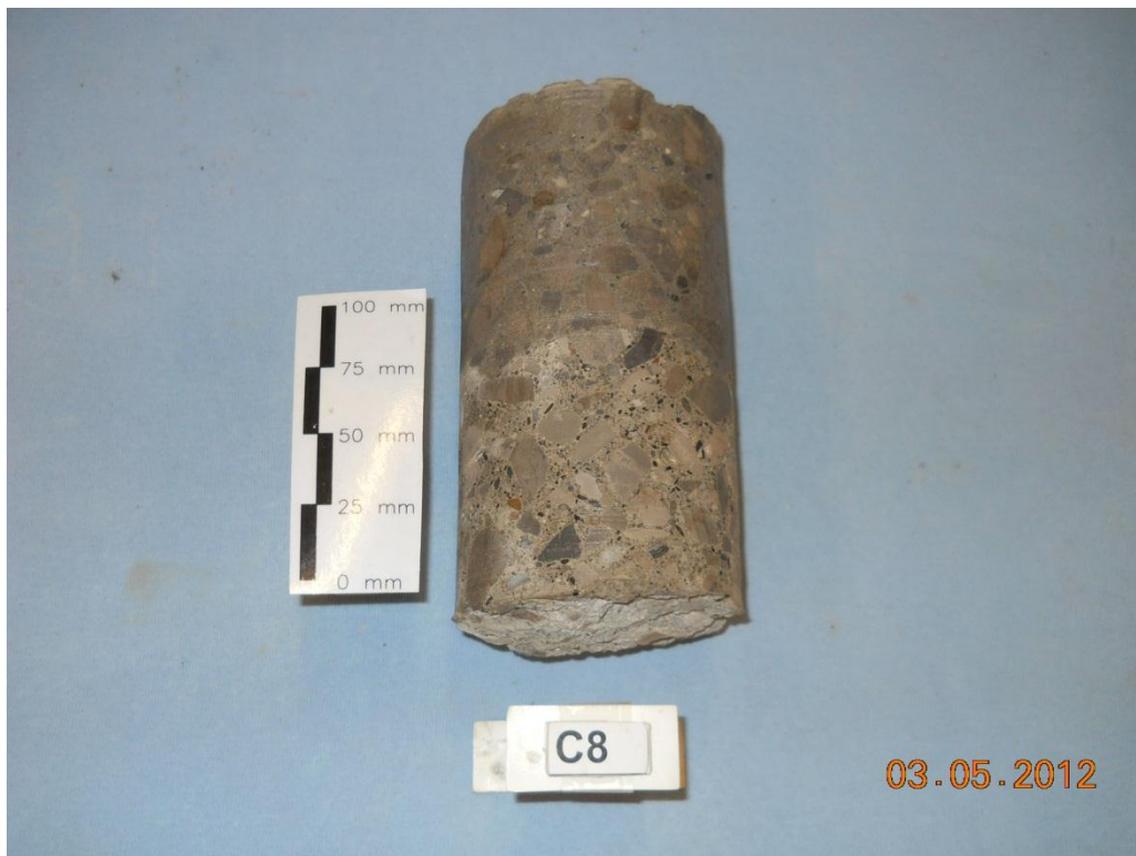
Core C8 - Note core removed from area of deck patching
