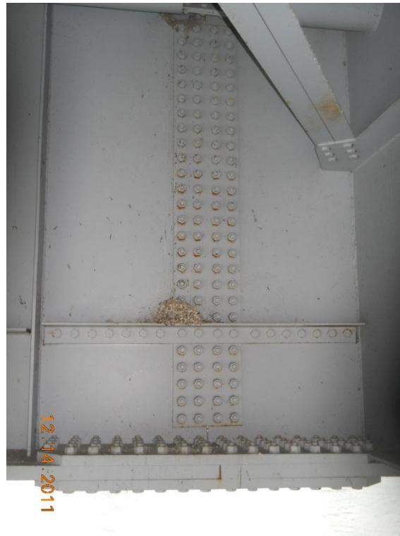
Photograph 97 - Transverse splice, span 4, typical
