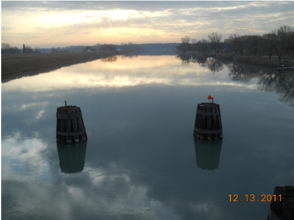
Photograph 39 - Looking south (downstream), note three of four protective dolphins
