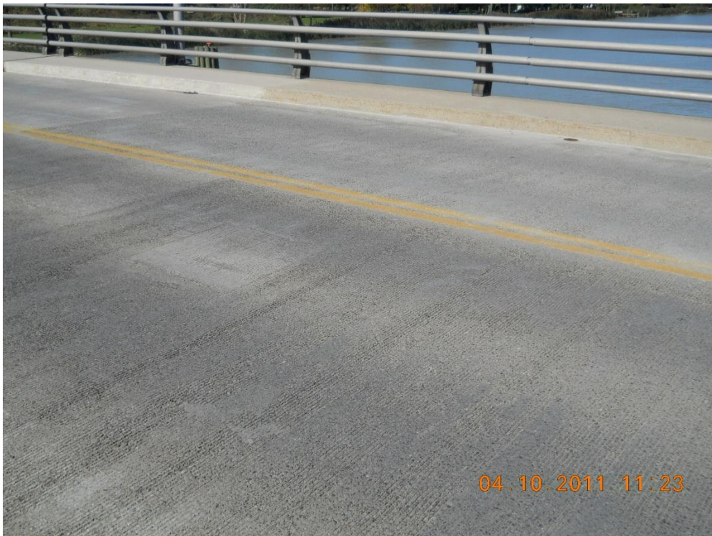
Photograph 14 - Span 5 wearing surface looking west
