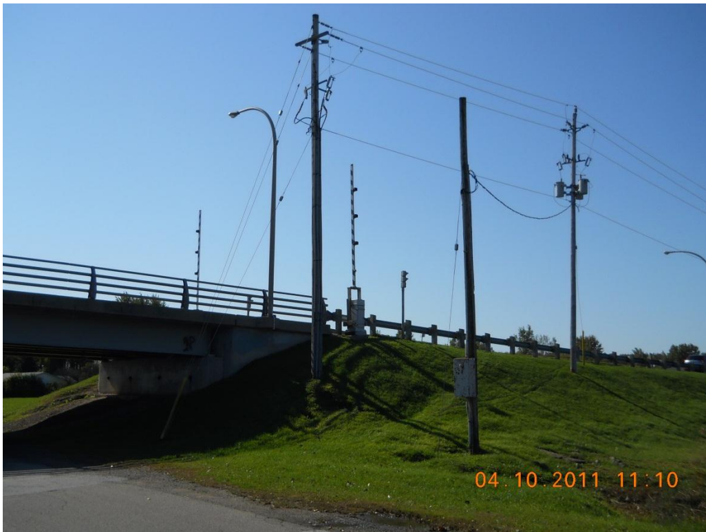
Photograph 136 - Note utilities at the northwest corner
