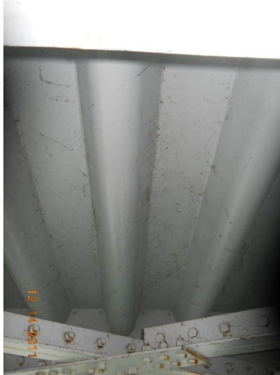
Photograph 107 - Soffit, span 4, typical steel orthotropic deck
