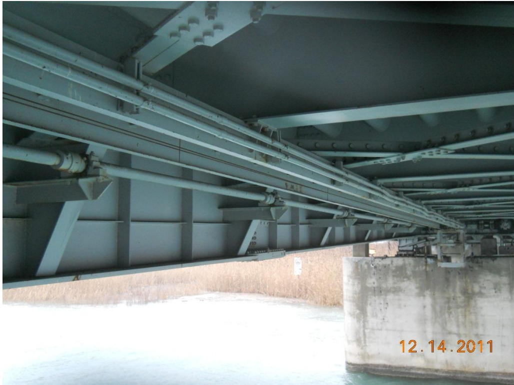
Photograph 101 - Span 4, girder 1 looking east, typical condition
