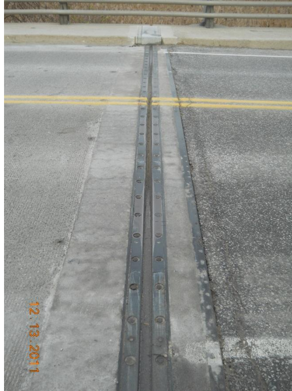
Photograph 37 - East abutment expansion joint looking north, note some debris accumulation
