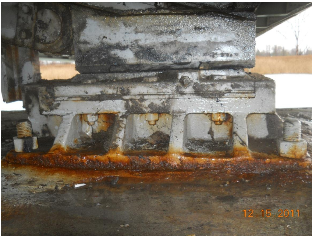
Photograph 78 - Span 3 west rest pier, south bearing, typical to other
