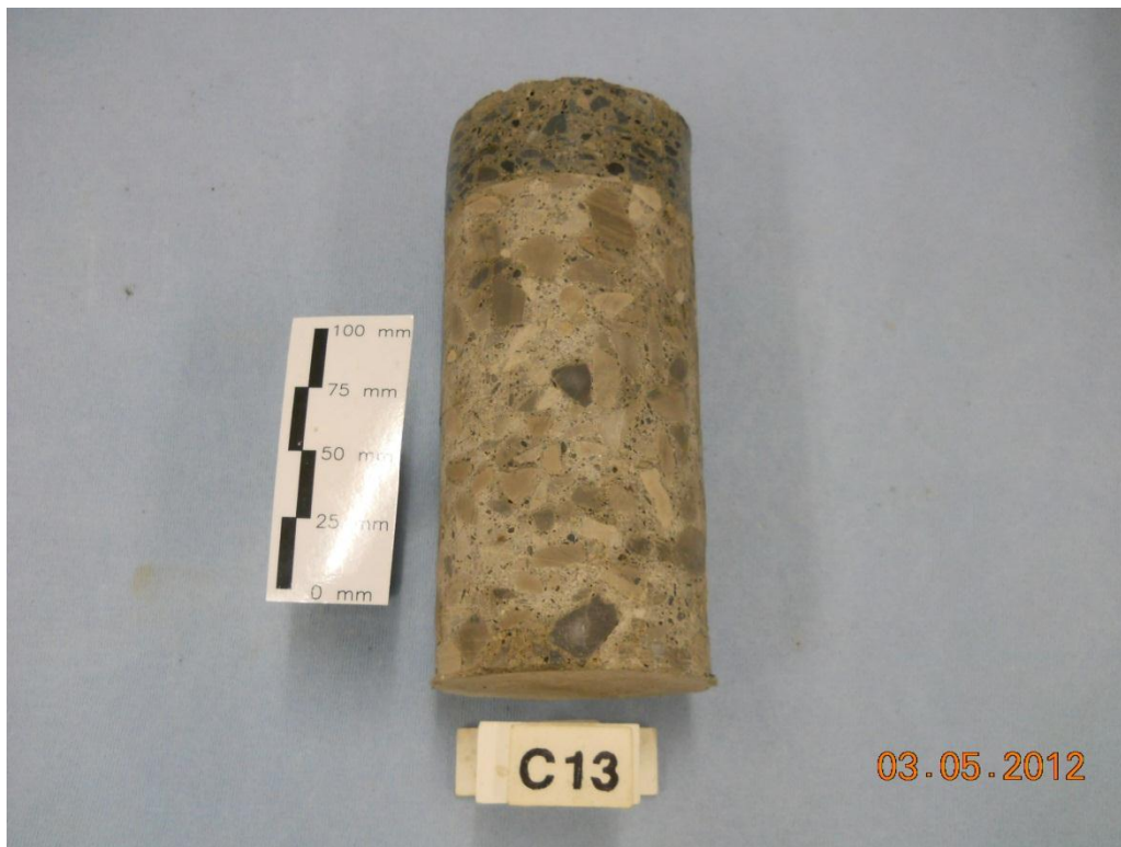
Core C13 - Note narrow horizontal crack at overlay/deck interface
