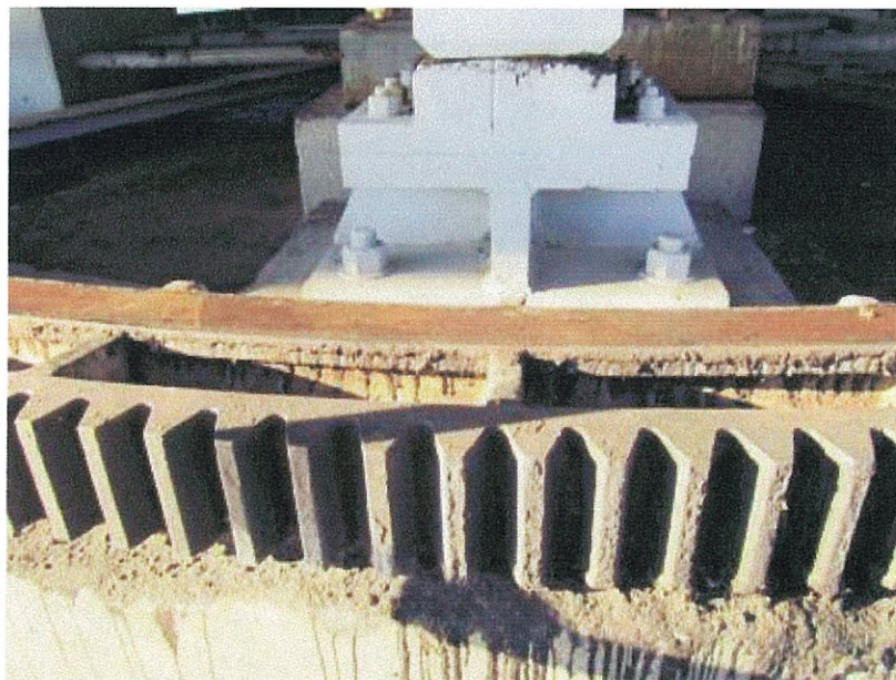
PHOTOGRAPH 14: SOUTH SIDE CENTRE PIER LIVE LOAD RELIEF WEDGE AND CIRCULAR RACK
