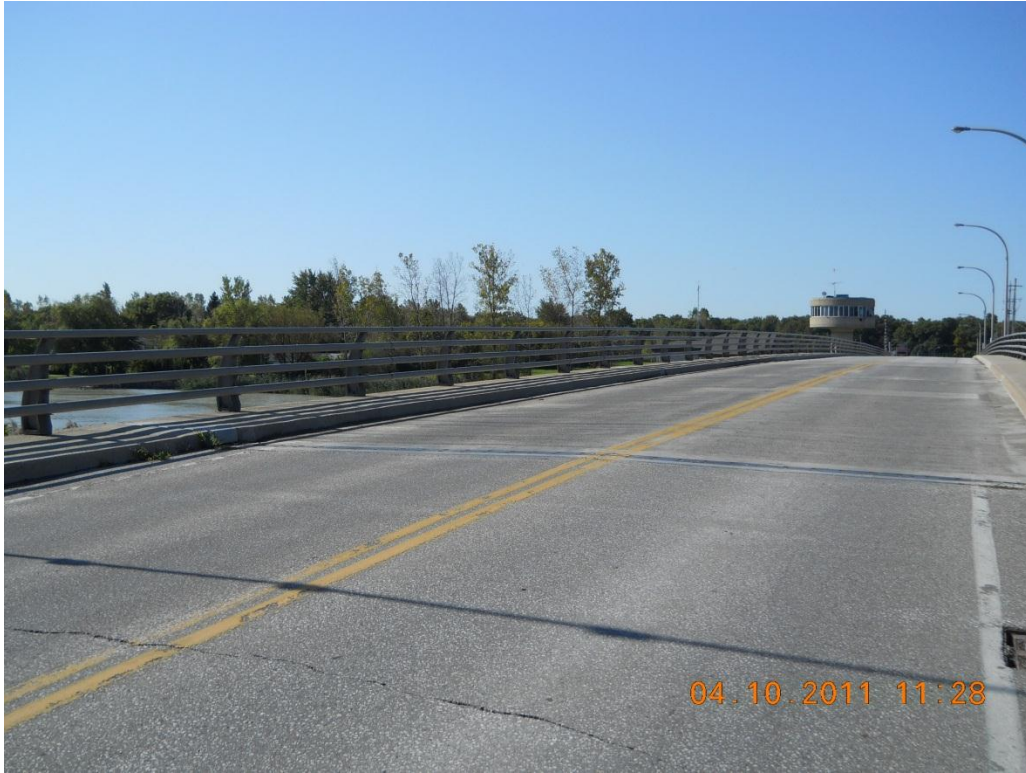
Photograph 27 - South railing looking west
