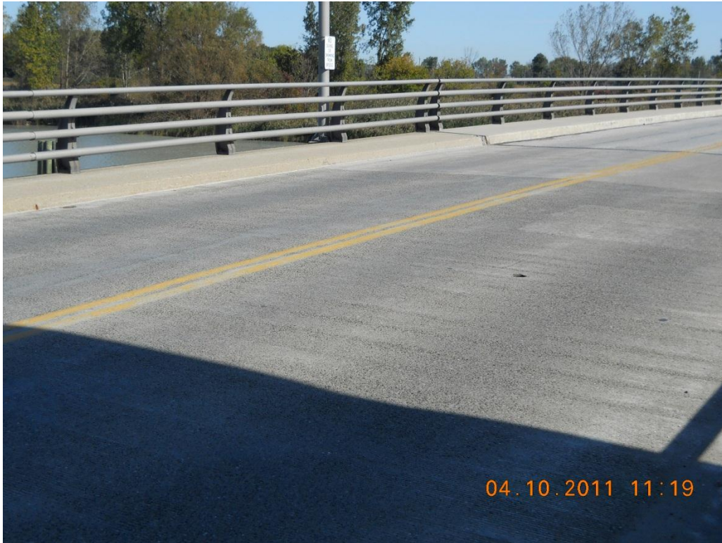
Photograph 19 - Span 2 wearing surface looking east
