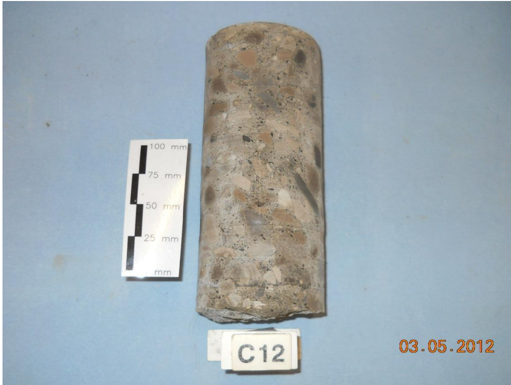
Core C12 - Note core removed from sidewalk, note air voids
