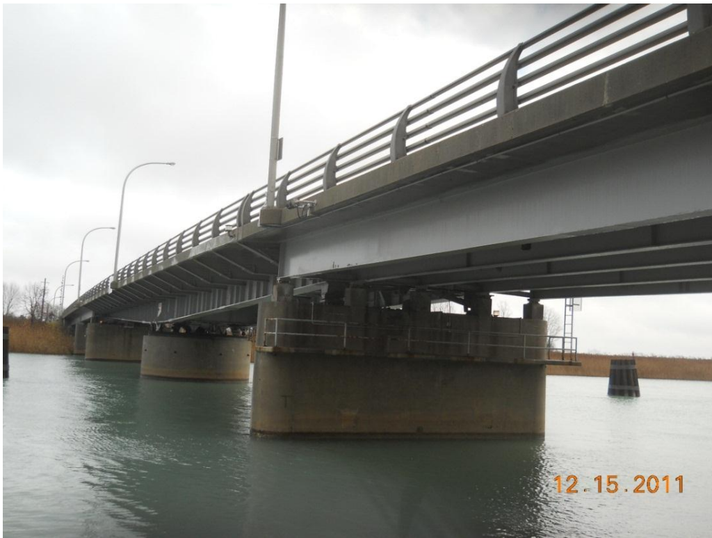
Photograph 1 - North elevation showing spans 2, 3, 4, 5 and 6 from the west
