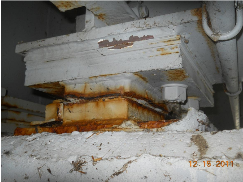
Photograph 75 - Span 5 east rest pier bearing, second from north, typical to others
