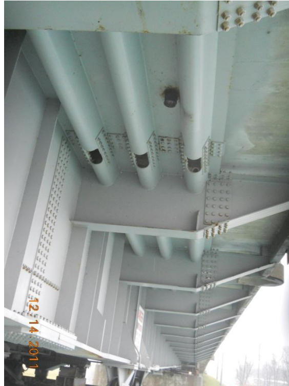
Photograph 105 - Span 4, north exterior soffit looking west
