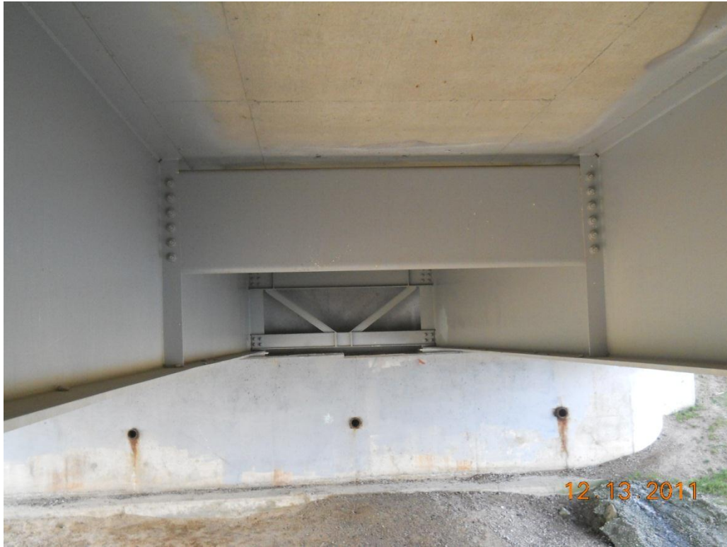
Photograph 121 - Diaphragm, span 1 looking west, typical condition
