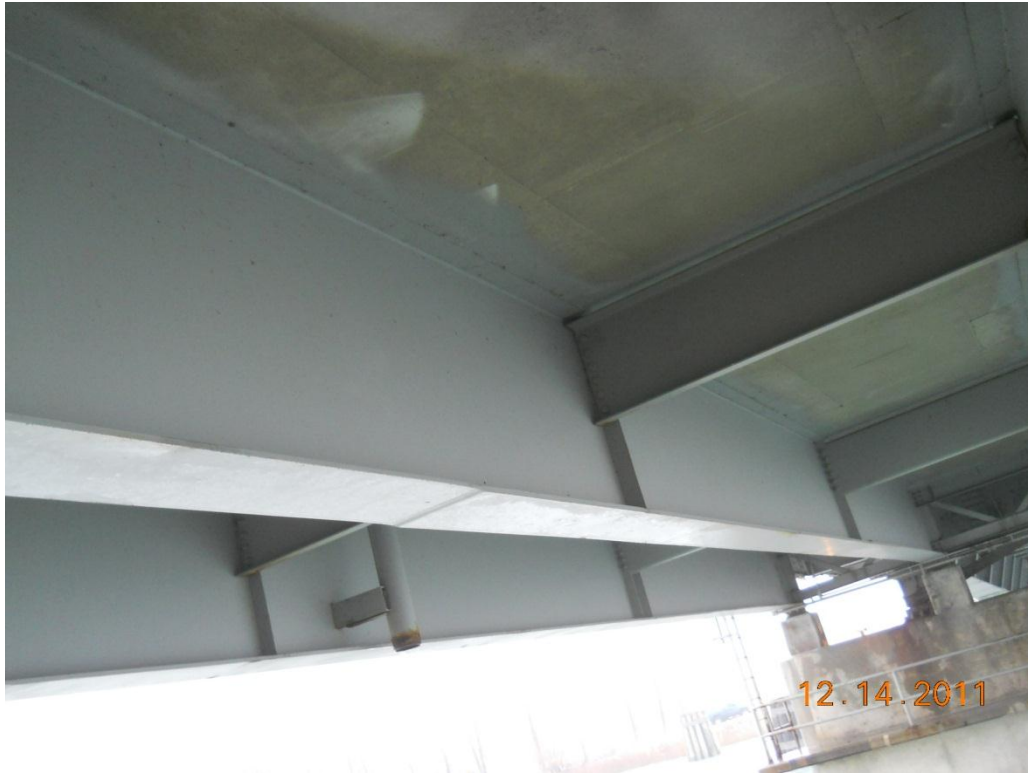
Photograph 95 - Soffit and girders 4, 5, span 5 looking west
