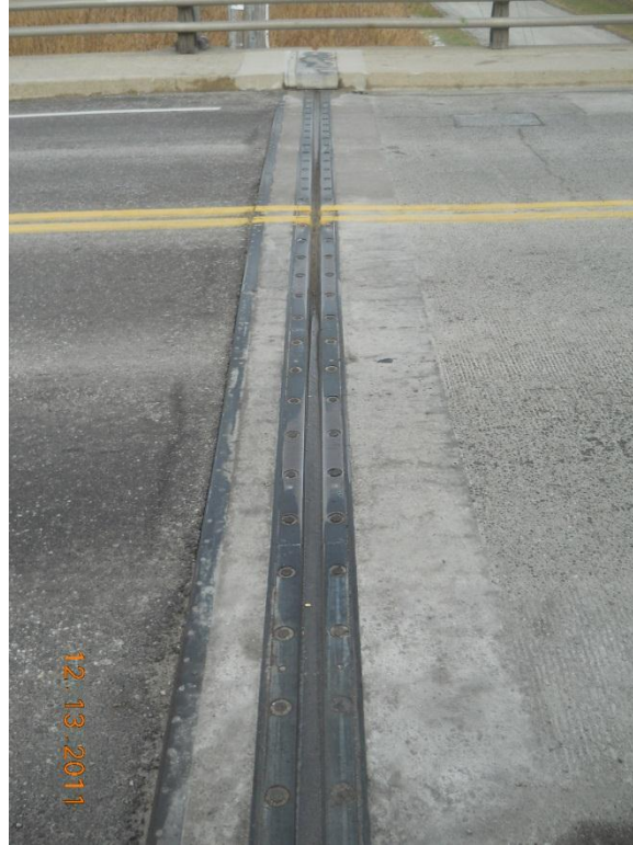
Photograph 31 - West abutment expansion joint looking north, note some debris accumulation
