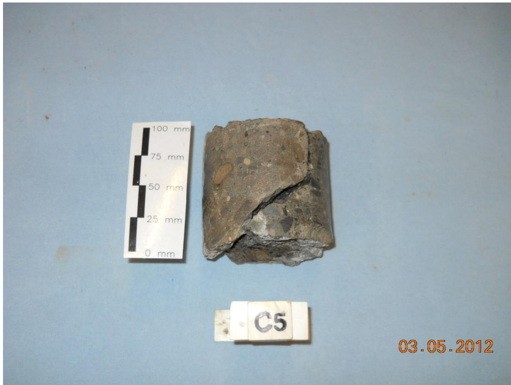
Core C5 - Note split due to coring operation
