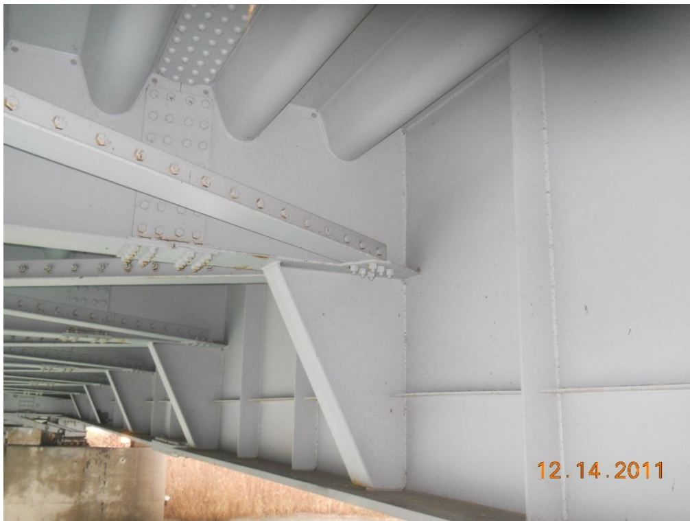
Photograph 100 - Span 4, girder 2 looking east, typical condition
