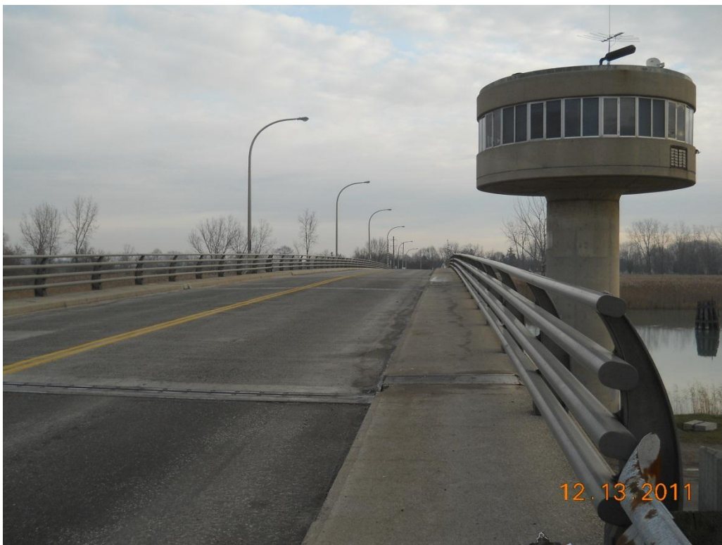
Photograph 10 - Looking east from west approach slab
