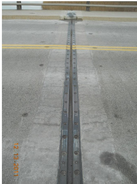
Photograph 36 - East shore pier expansion joint looking north, note some debris accumulation
