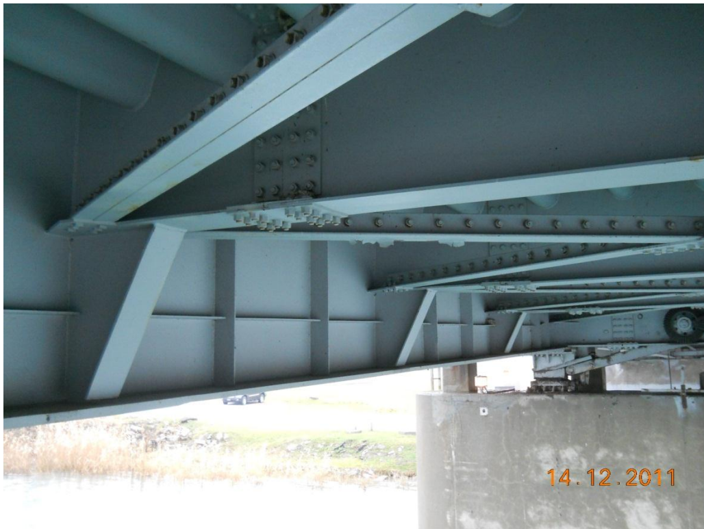
Photograph 114 - Span 3, girder 2 looking west
