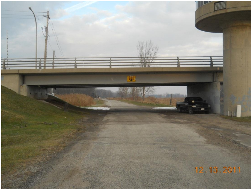
Photograph 3 - South elevation of span 1
