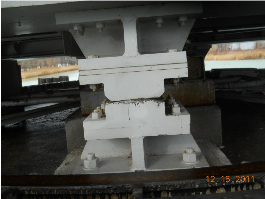
Photograph 77 - Pivot pier, south live load relief bearing
