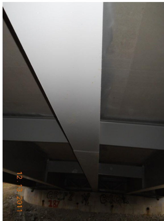
Photograph 82 - Soffit and girder 4, span 1 looking east
