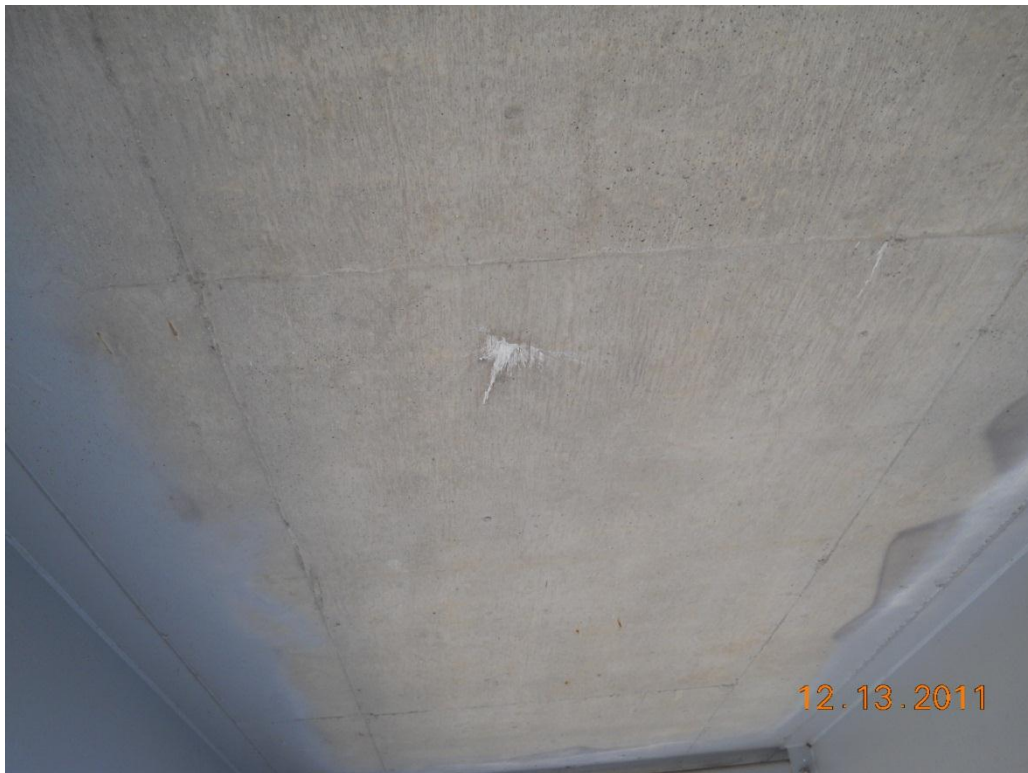
Photograph 88 - Soffit, span 1, typical condition
