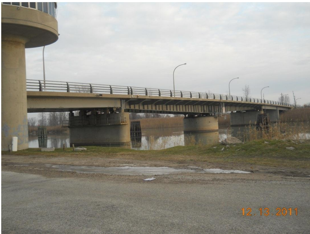
Photograph 2 - South elevation showing spans 2, 3, 4, 5 and 6 from the west
