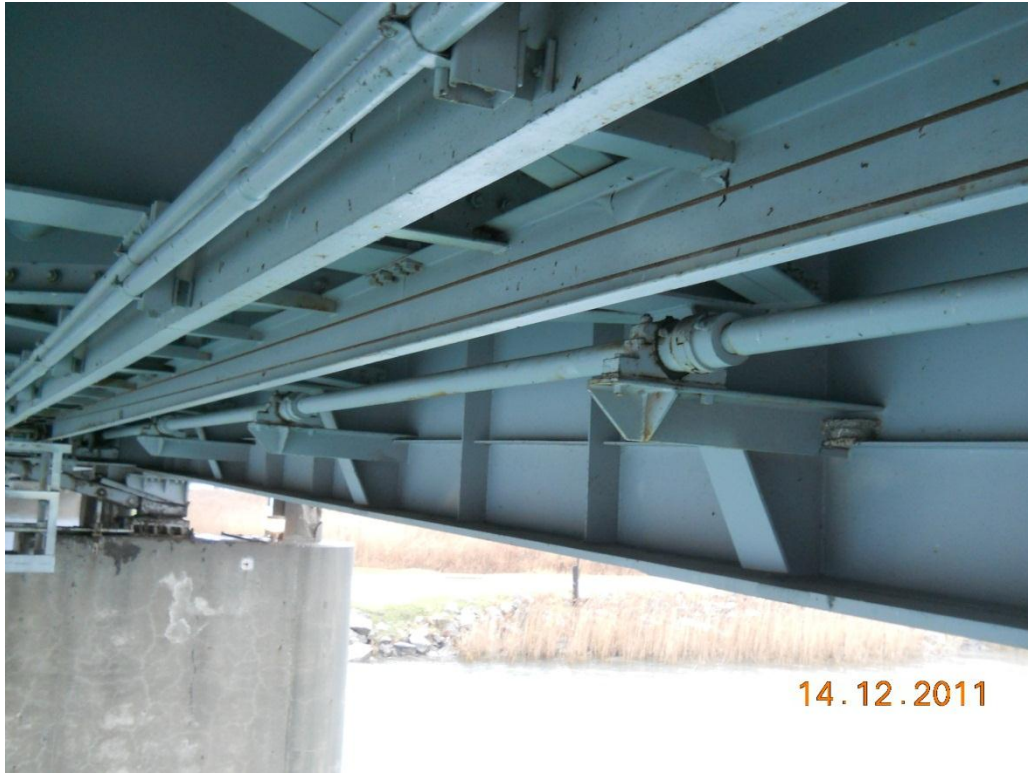
Photograph 113- Span 3, girder 1 looking west
