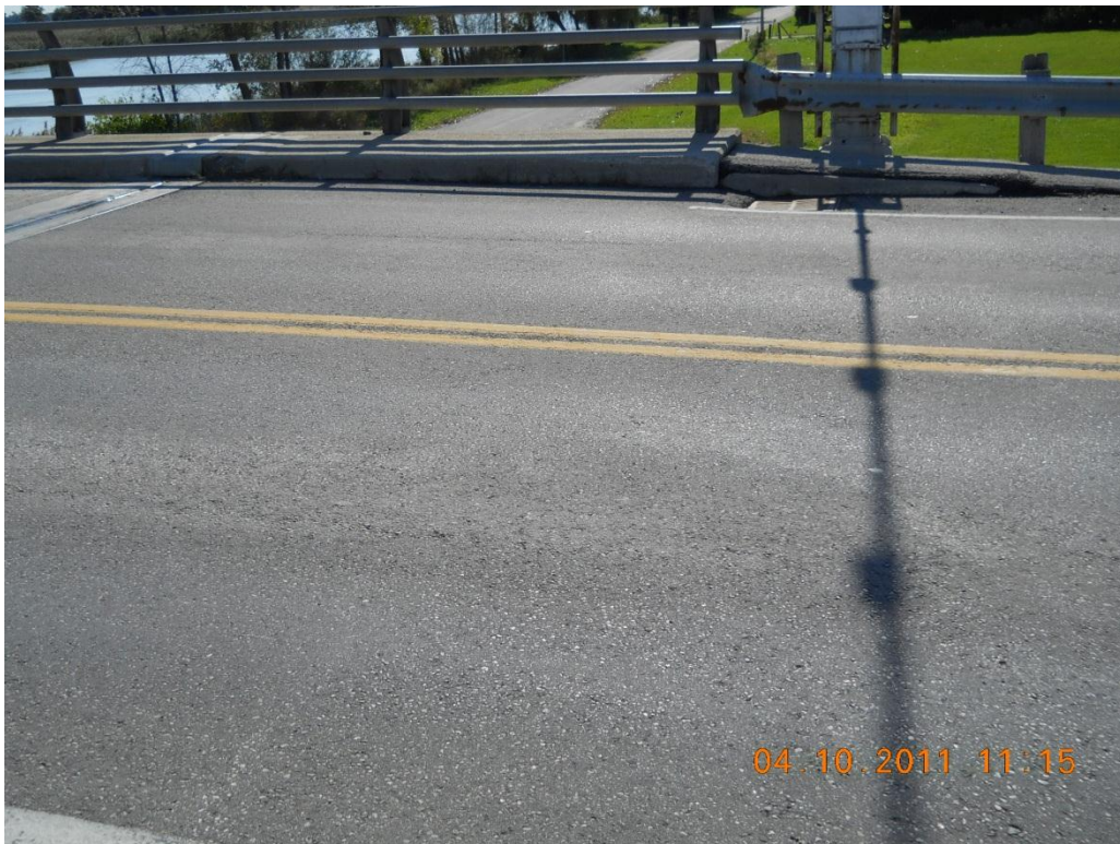
Photograph 12 - West approach slab wearing surface
