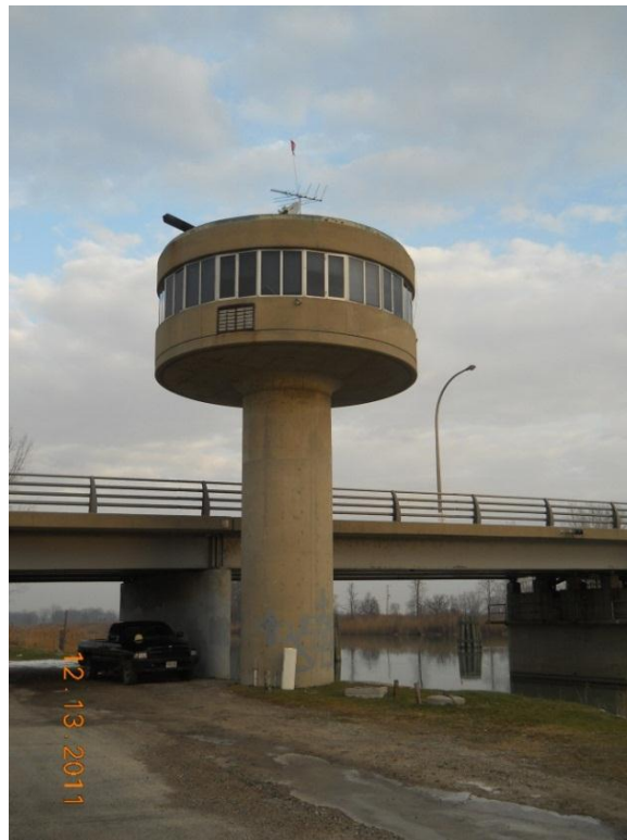
Photograph 4 - South elevation of the control tower
