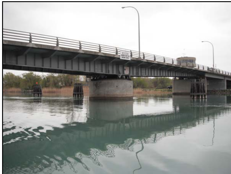
Figure 5: Pivot Pier, North Face
