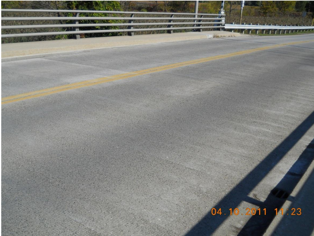
Photograph 13 - Span 6 wearing surface looking east
