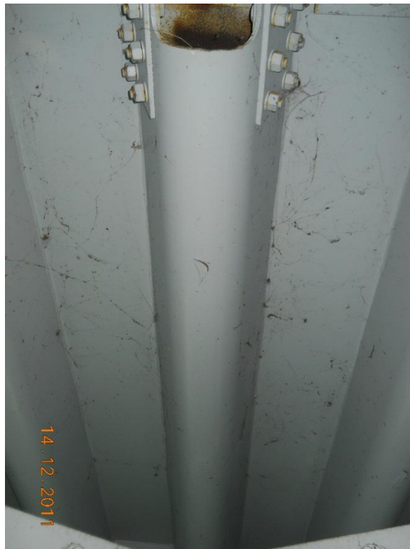
Photograph 112 - Soffit, span 3, typical condition
