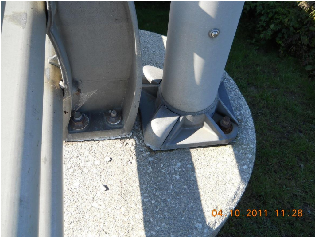
Photograph 29 - Typical railing and lamp post anchorages
