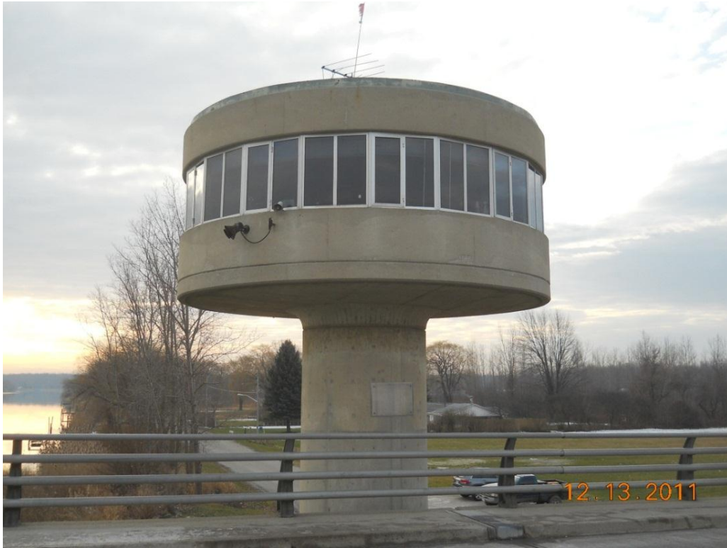
Photograph 5 - North elevation of the control tower
