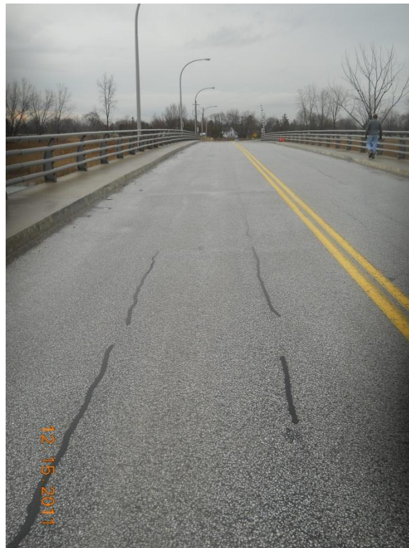
Photograph 18 - Span 3 asphalt wearing surface looking east, westbound lane, note sealed crack
