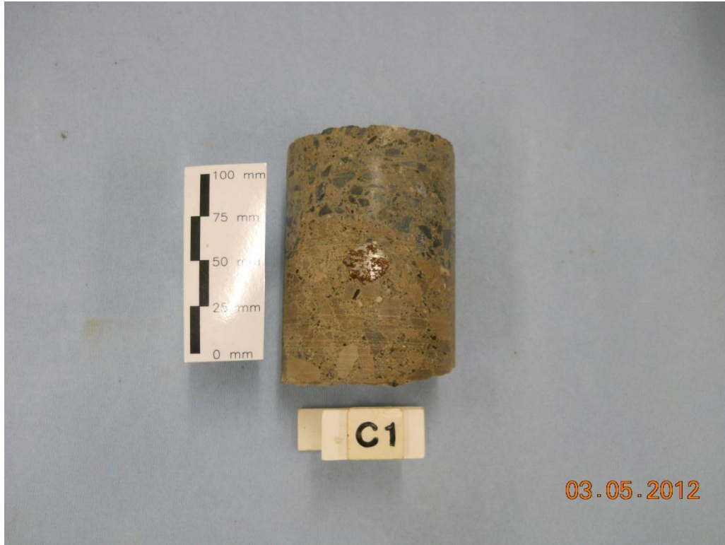
Core C1 - Note light surface rusting on reinforcing steel bar
