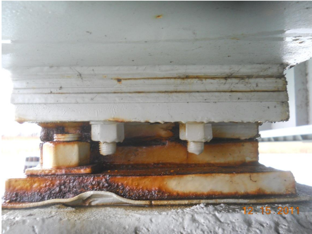
Photograph 79 - Span 2 west rest pier bearing, first from north, typical to others
