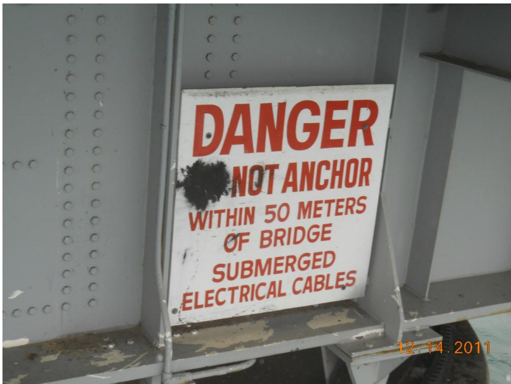
Photograph 134 - Danger sign over pivot pier north side. Typical on south side
