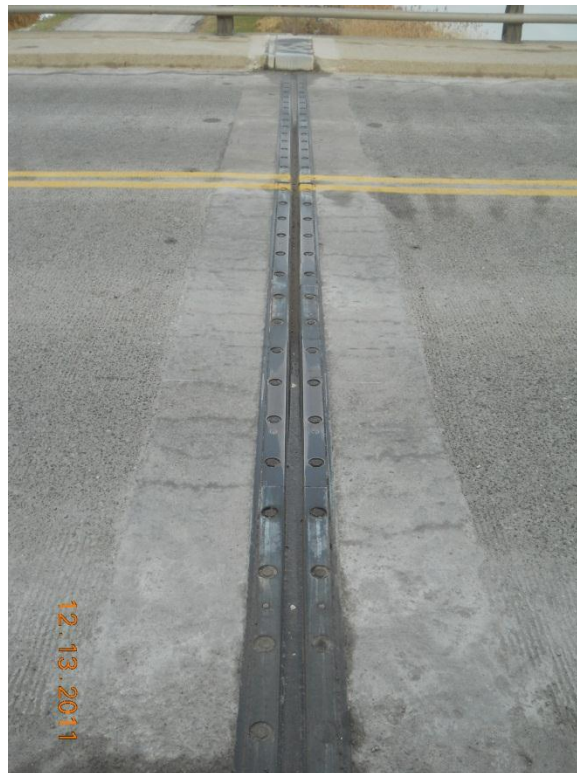
Photograph 32 - West shore pier expansion joint looking north, note some debris accumulation
