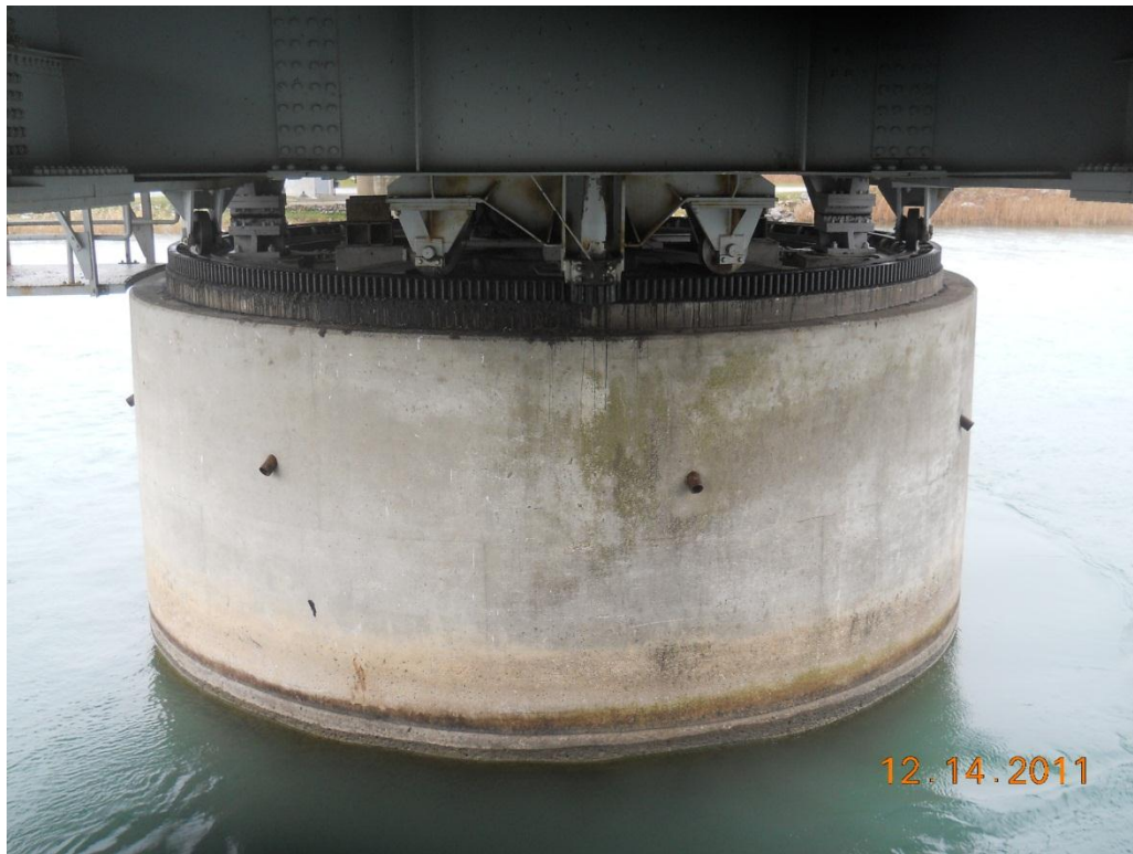
Photograph 60 - East face of pivot pier
