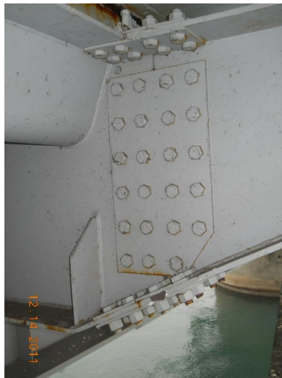
Photograph 102 - Span 4, typical connection of exterior cross beams
