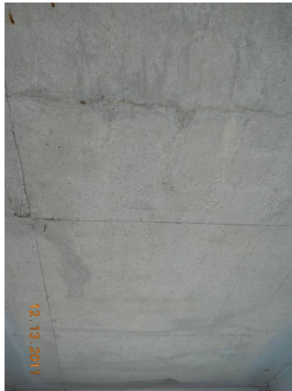
Photograph 86 - Soffit, span 2, typical condition
