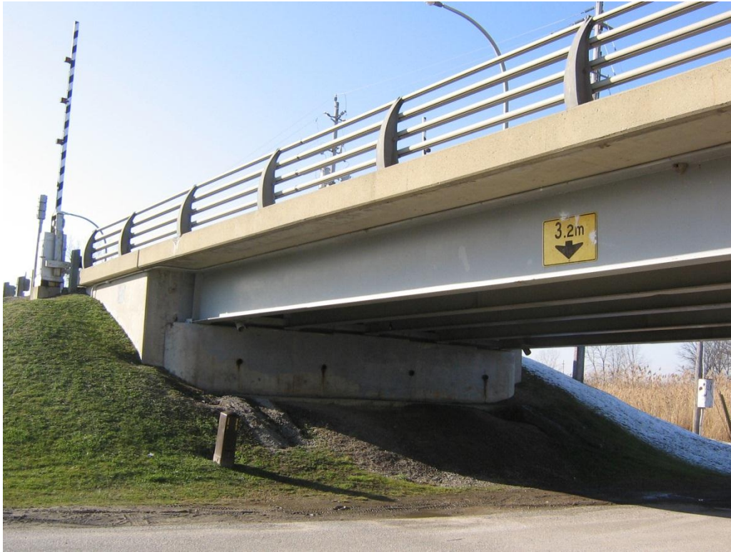
Photograph 137 - Note utility box at southwest corner
