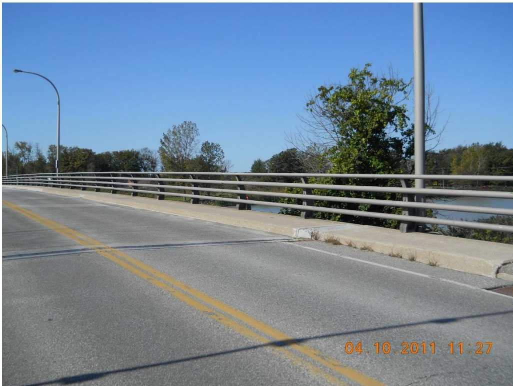
Photograph 26 - North railing looking west
