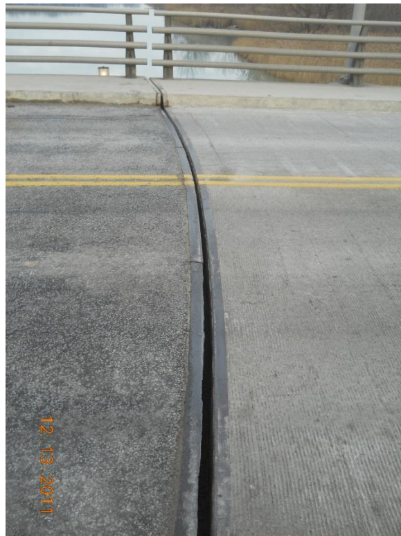
Photograph 34 - East rest pier joint looking north
