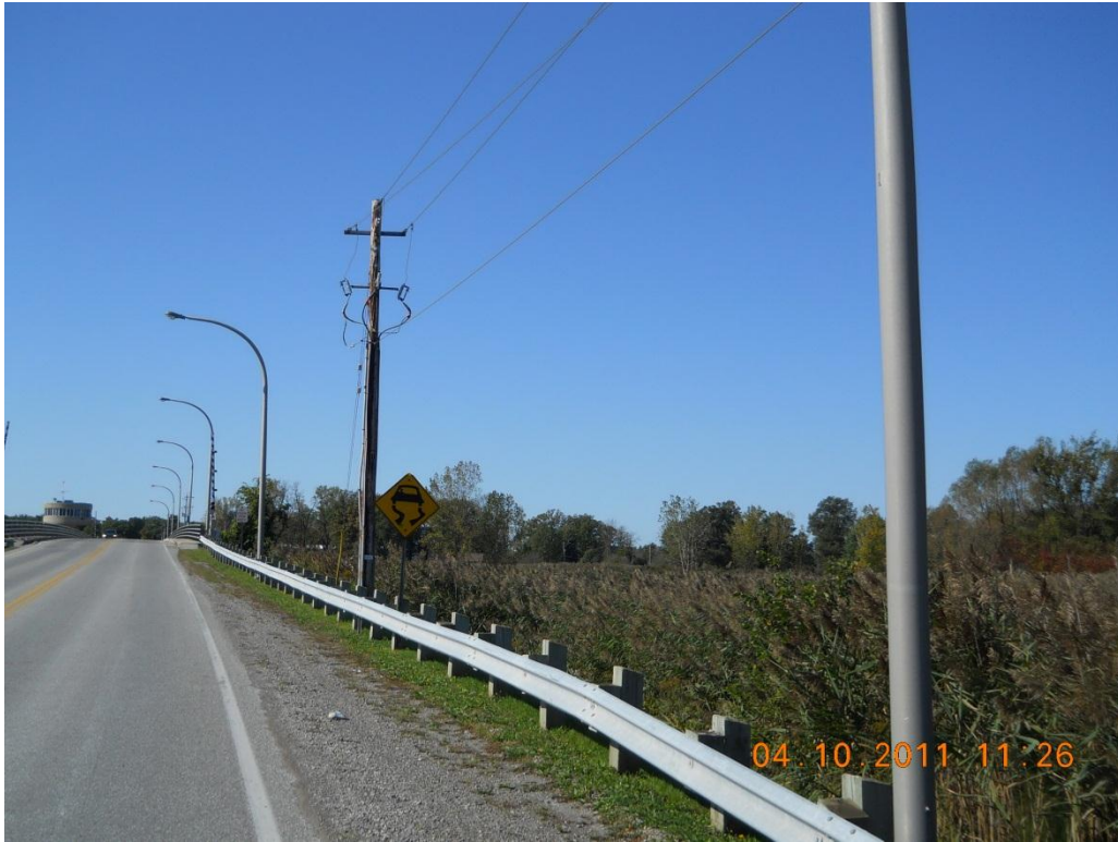
Photograph 135 - Note utilities at the northeast corner
