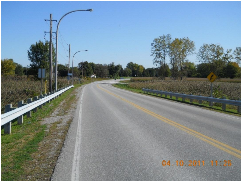
Photograph 6 - East approach looking east
