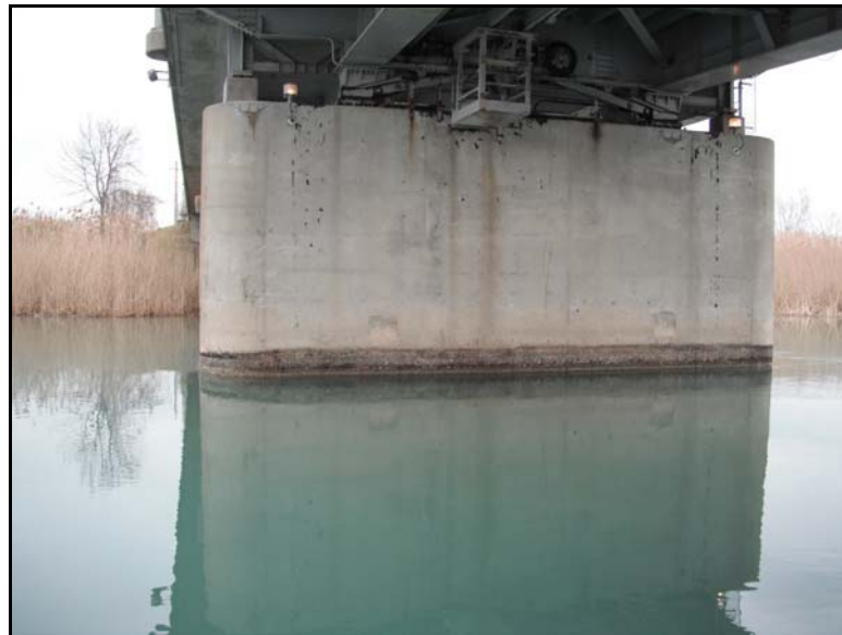
Figure 6: East Rest Pier, West Face
