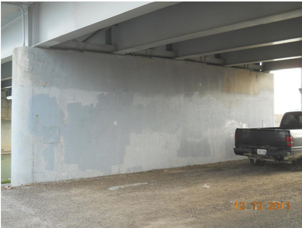
Photograph 72 - West face of west shore pier
