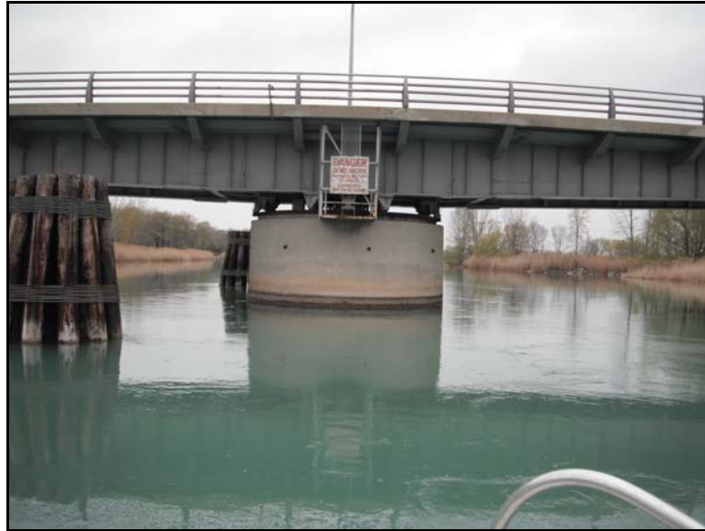
Figure 4: Pivot Pier, South Face
