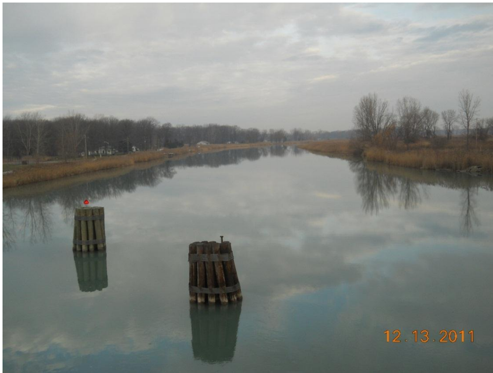
Photograph 38 - Looking north (upstream), note two of four protective dolphins. Note that the right dolphin is leaning towards structure.
