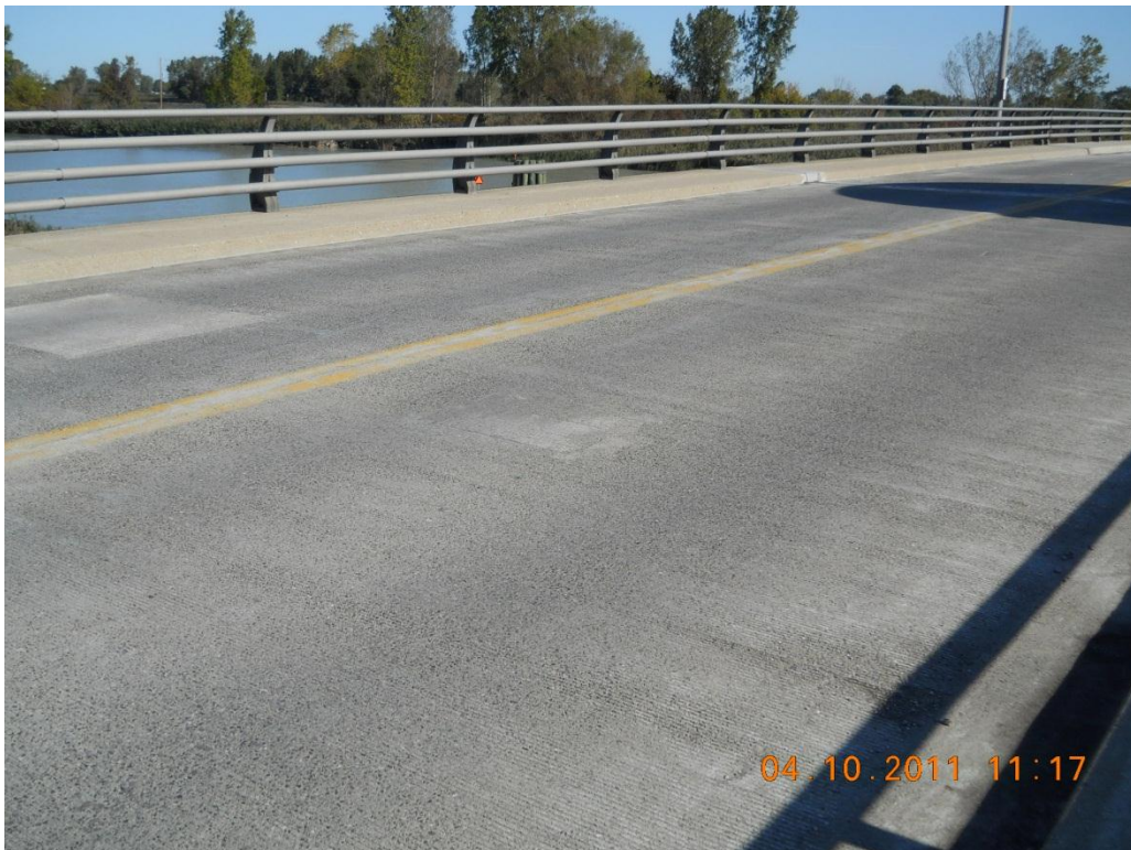
Photograph 20 - Span 1 wearing surface looking east
