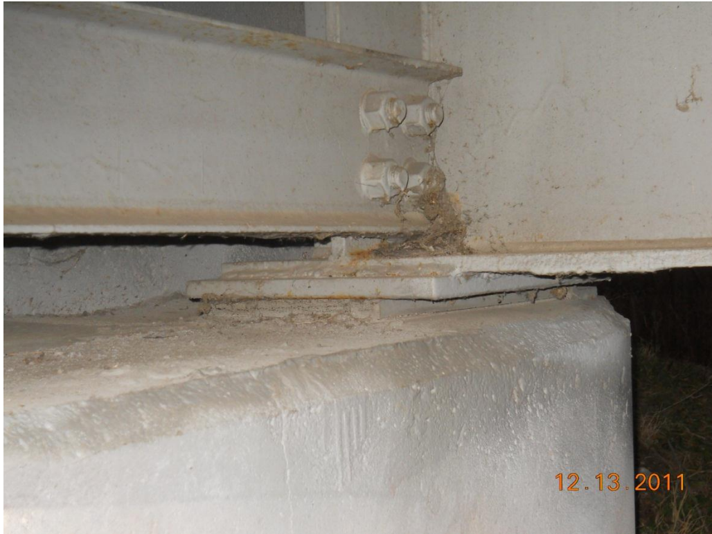
Photograph 73 - East abutment bearing, fifth from north end, typical to others
