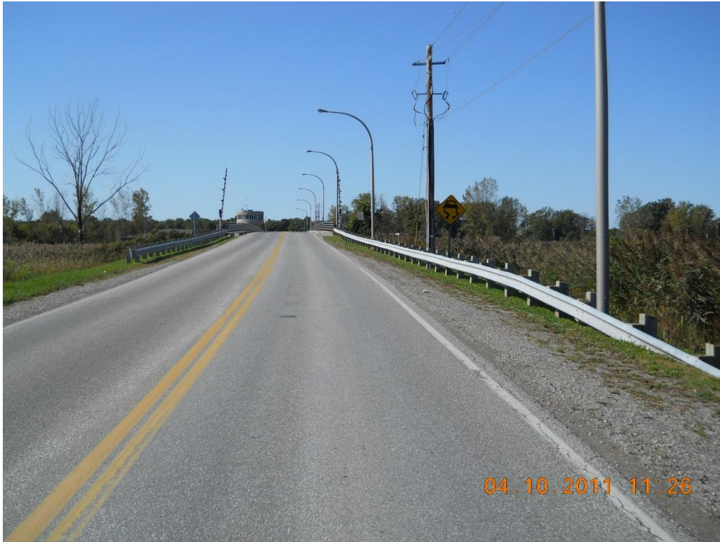
Photograph 7 - East approach looking west
