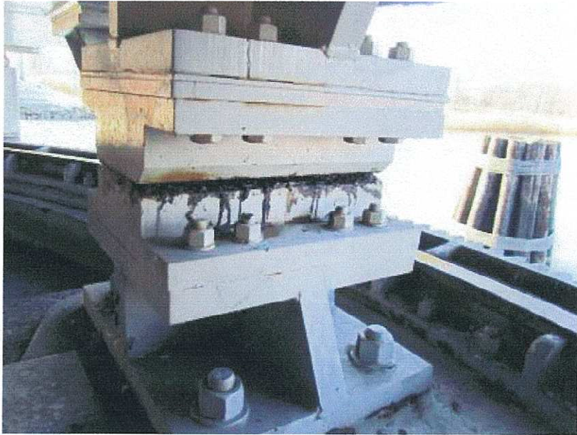
PHOTOGRAPH 27: NORTH SIDE CENTRE PIER LIVE LOAD RELIEF WEDGE
