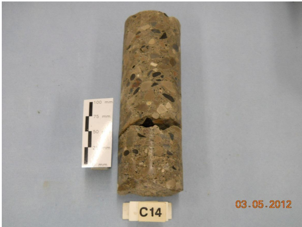
Core C14 - Note, core split during coring operation. Note narrow horizontal crack along sidewalk/deck interface below split
