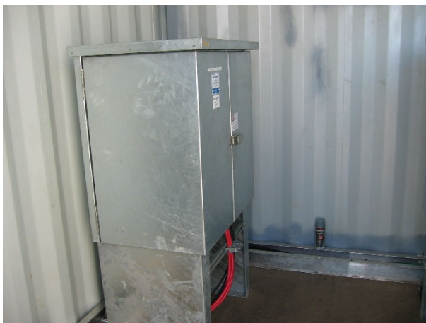
Rectifiers R2, R4 and R5-7 installed in the electrical container.
