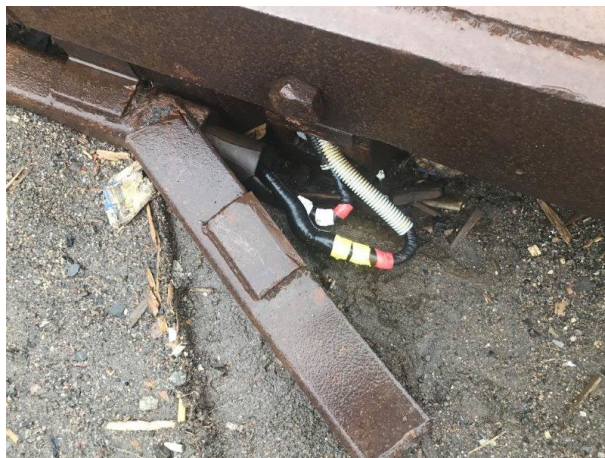
Examples of main anodes cables and HSS repairs.
