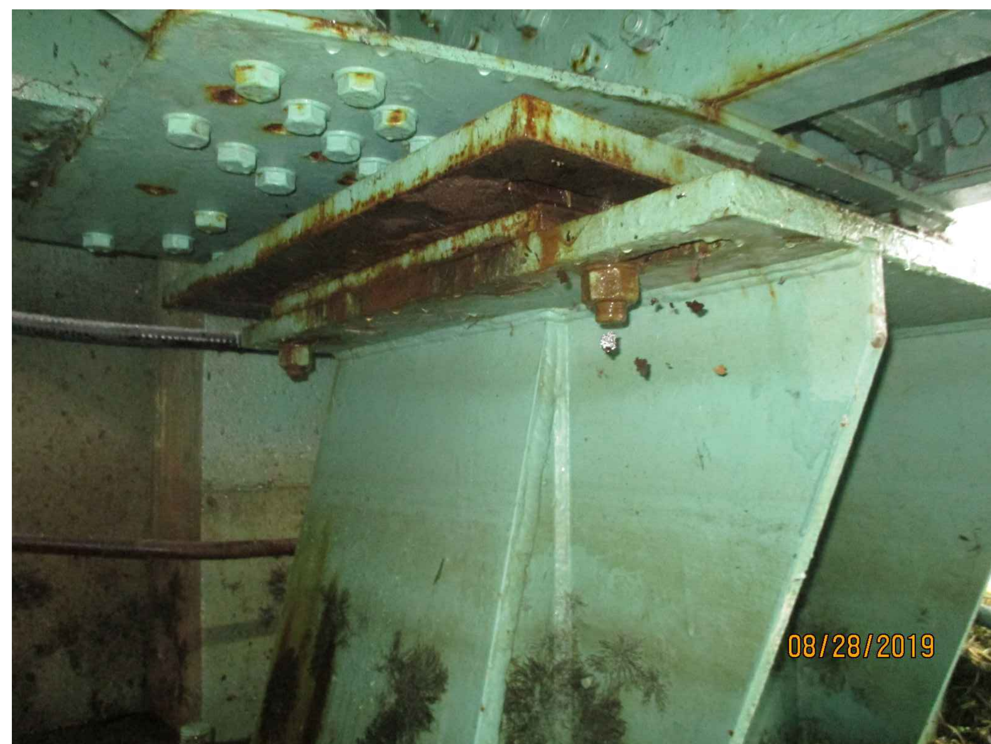
PHOTO OF LIVE LOAD SUPPORT UNDER SIDE
