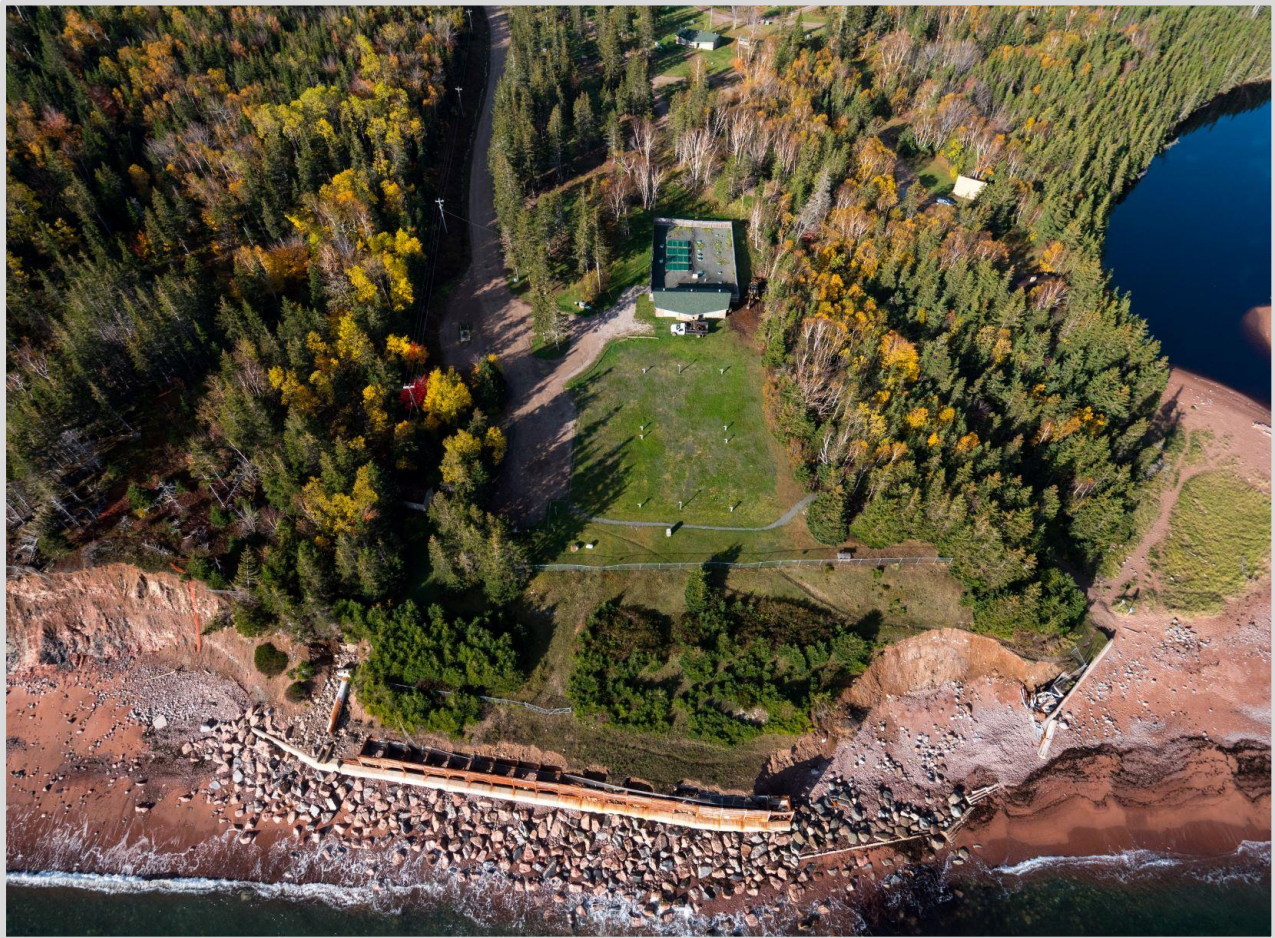
Figure 1. Broad Cove Campground retaining wall site location, 2019 aerial photograph.
