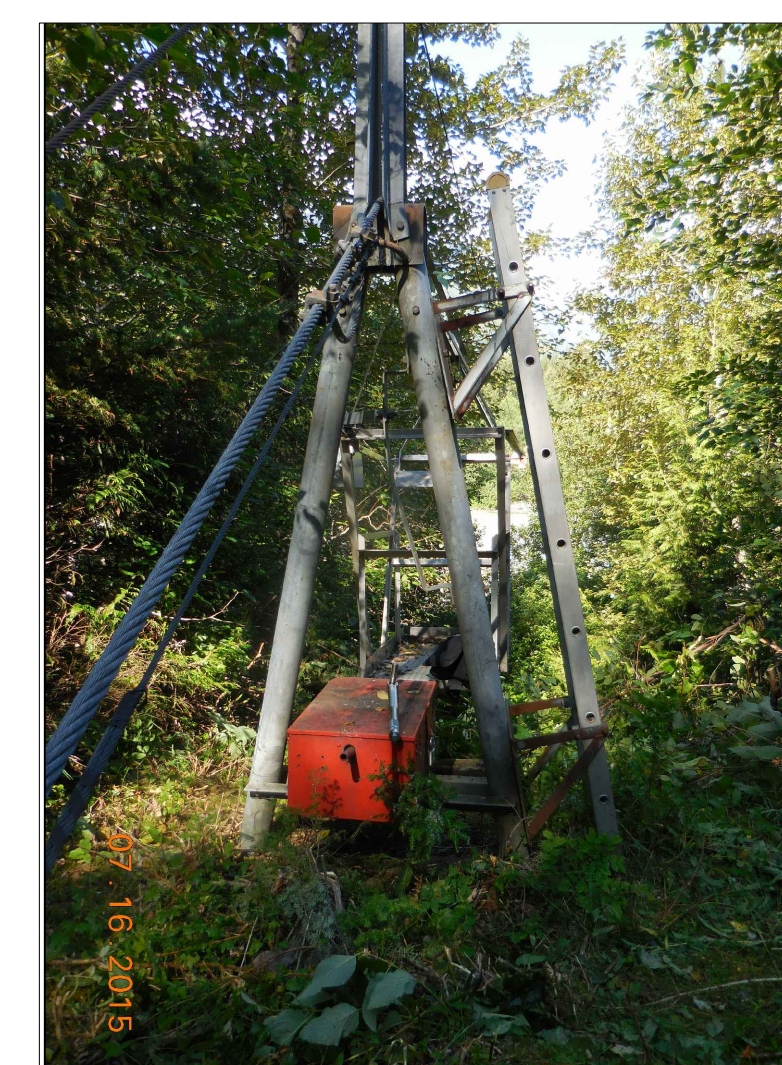
PHOTO 2: BACK VIEW OF EXISTING A-FRAME AND COMPONENTS
