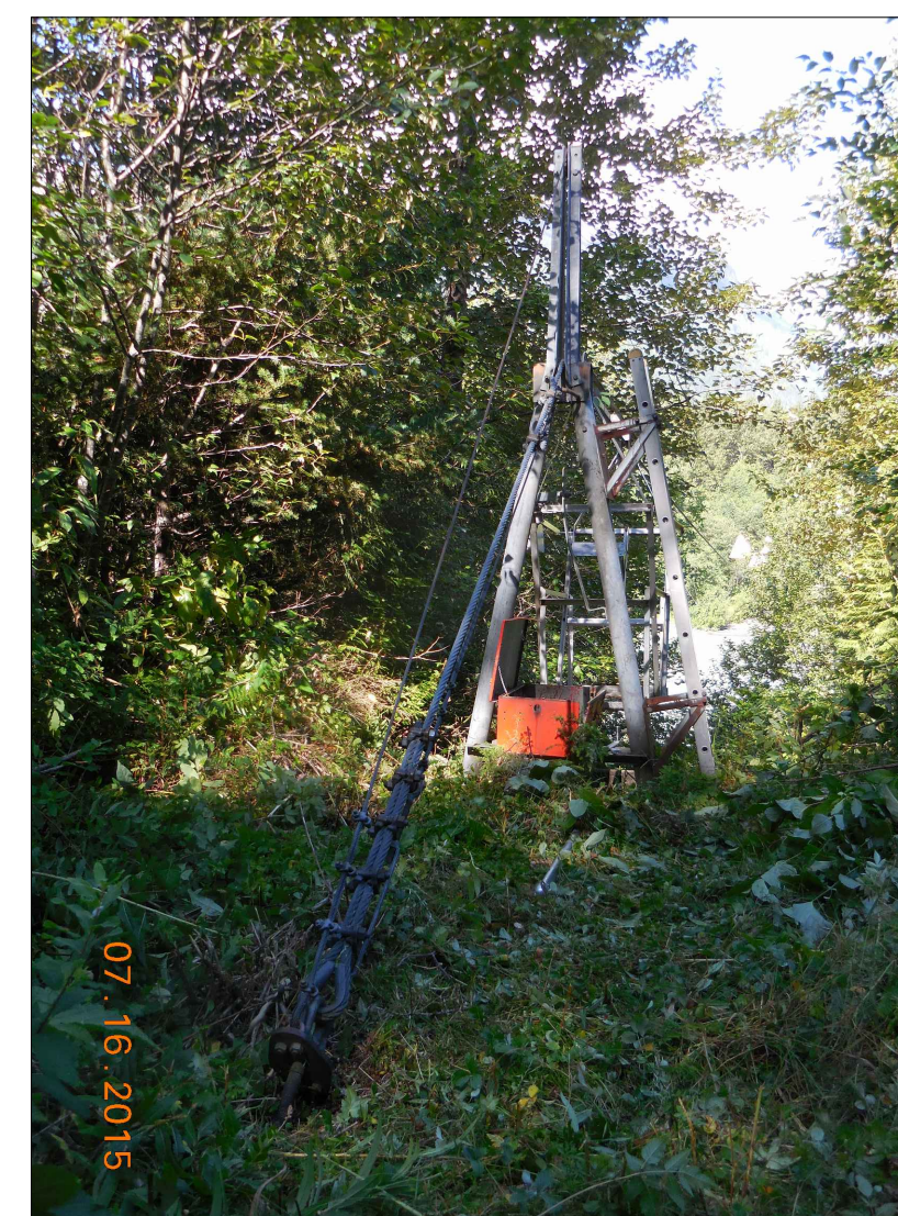
PHOTO 1: HOME-SIDE GENERAL VIEW
