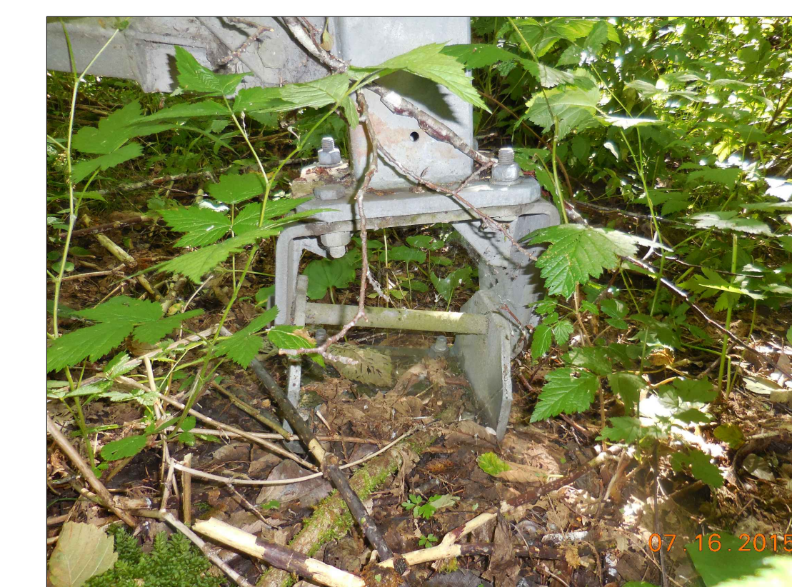
PHOTO 8: EXISTING CONNECTION OF A-FRAME TO FOOTING
