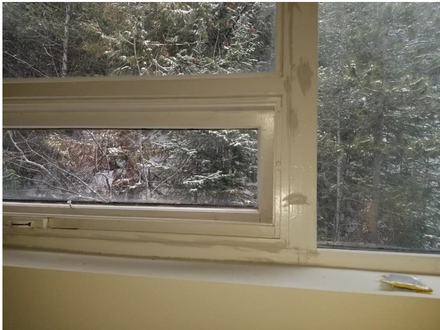
Photograph 6: Asbestos-Containing Window Caulking West Recreation Room
