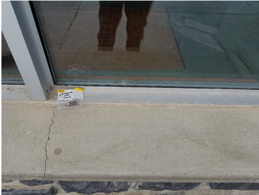
Photograph 1: Asbestos-Containing Glazing Putty Ground Floor East
