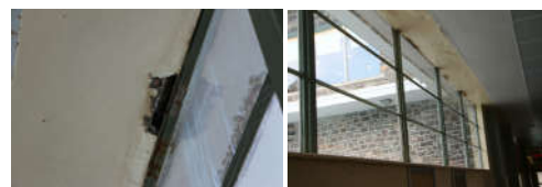
TYP. HEAD CONDITION @ MAIN FLOOR POOL COORIDOR. REMOVE EXISTING DAMAGED DRYWALL
