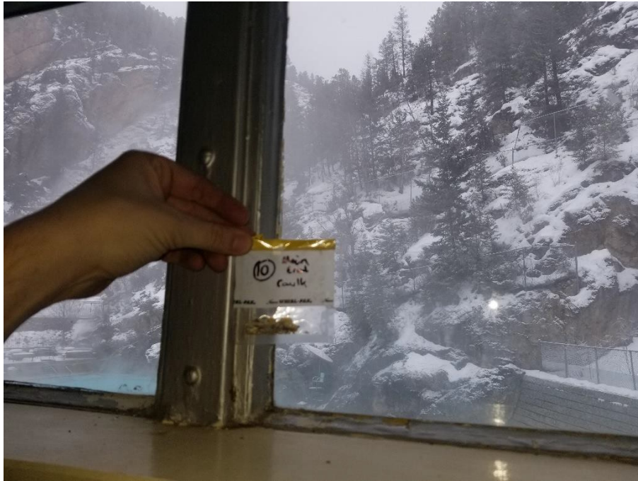
Photograph 5: Asbestos-Containing Window Caulking Main Floor East
