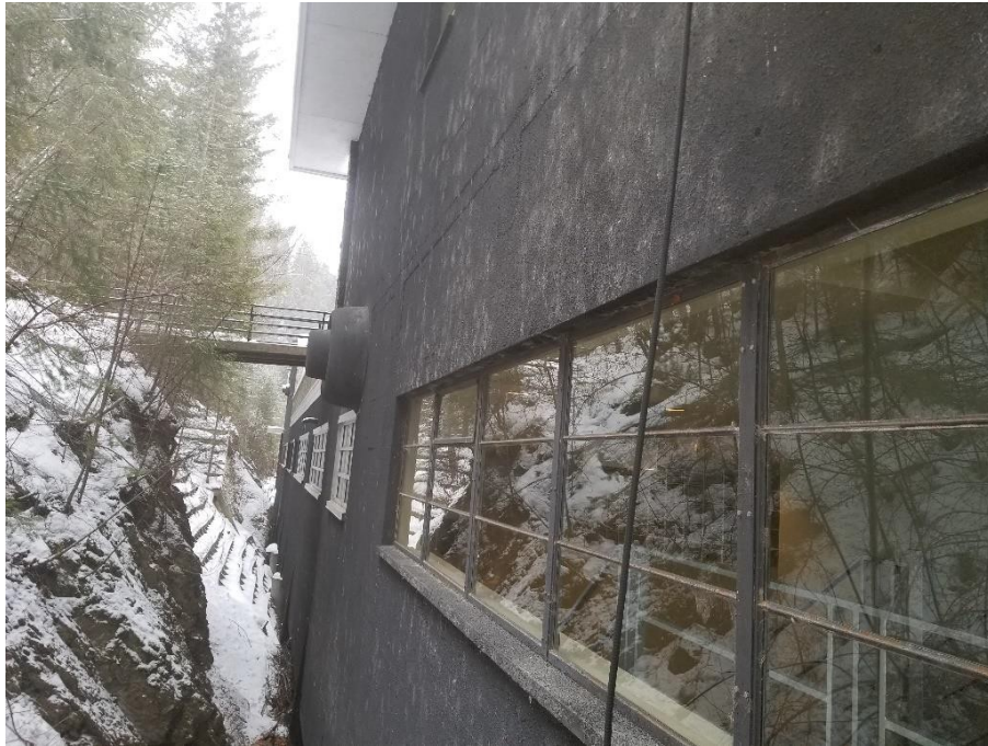
Photograph 7: Asbestos-Containing Stucco
