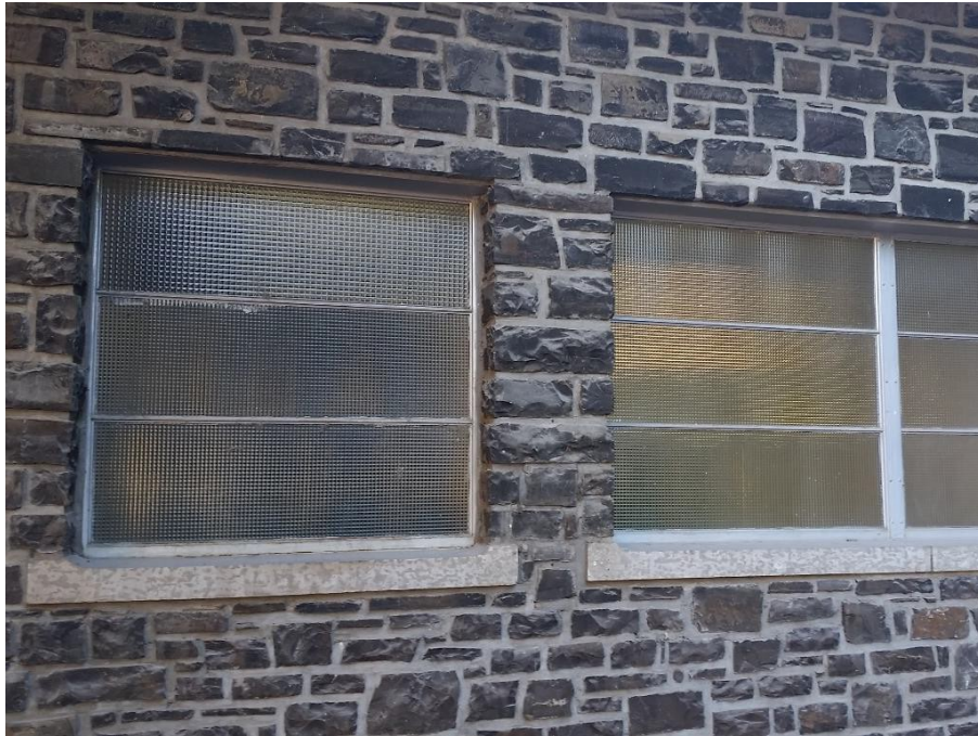
Photograph 9: Silver Lead-Based Paint on Exterior Bathroom Window Frames
