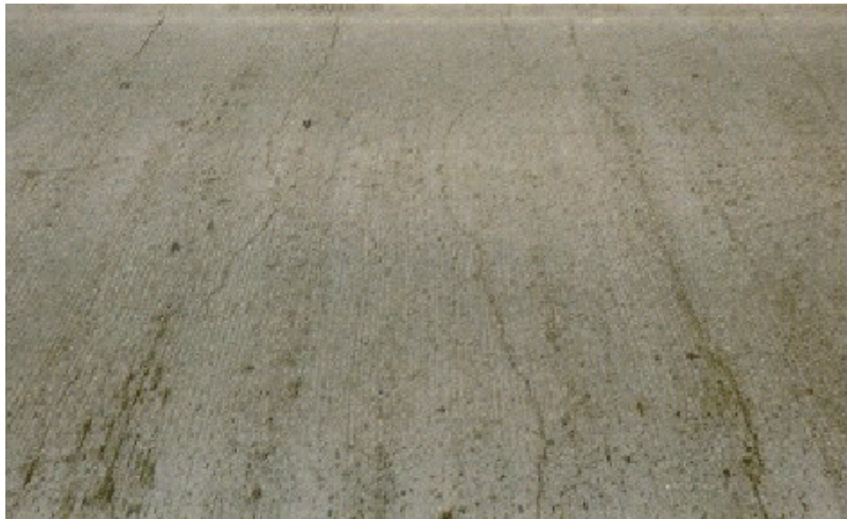
Figure A7.1.2(b) Exposed Concrete Deck
