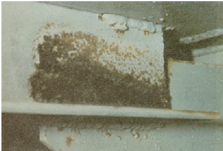
Figure 2.8.1(d) Chemical Attack
