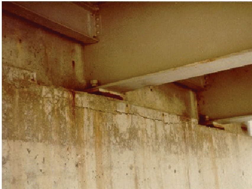
Figure A3.1.2(t) Concrete Bearing Seats
