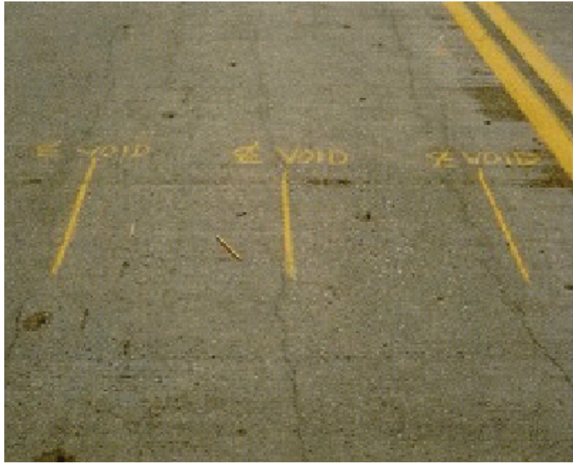
Figure A7.1.2(a) Exposed Concrete Deck of a Voided Slab
