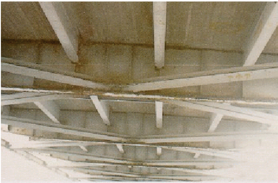
Figure A6.1.2(p) Bottom Lateral Bracing
