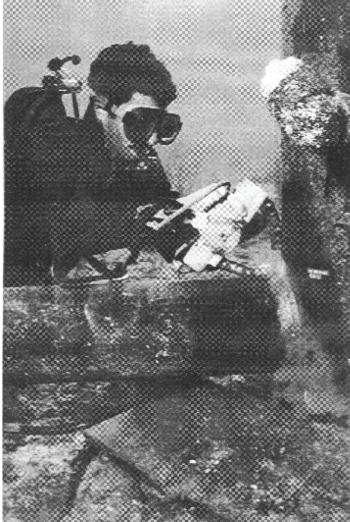
Figure E1.4.2 Underwater Magnetic Particle Inspection
