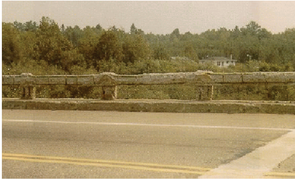
Figure A8.1.2(g) Concrete Guide Rail
