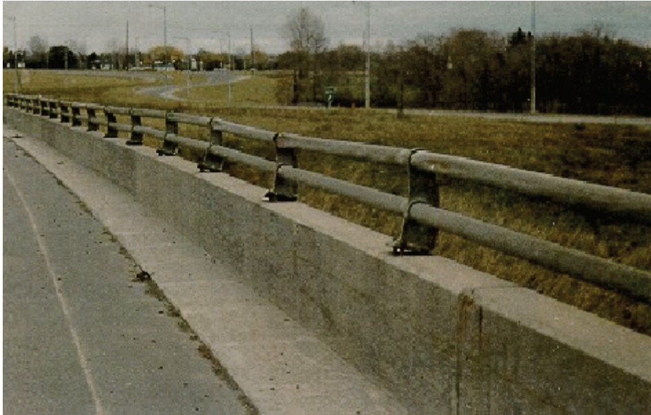
Figure A8.1.2(a) Parapet Wall
