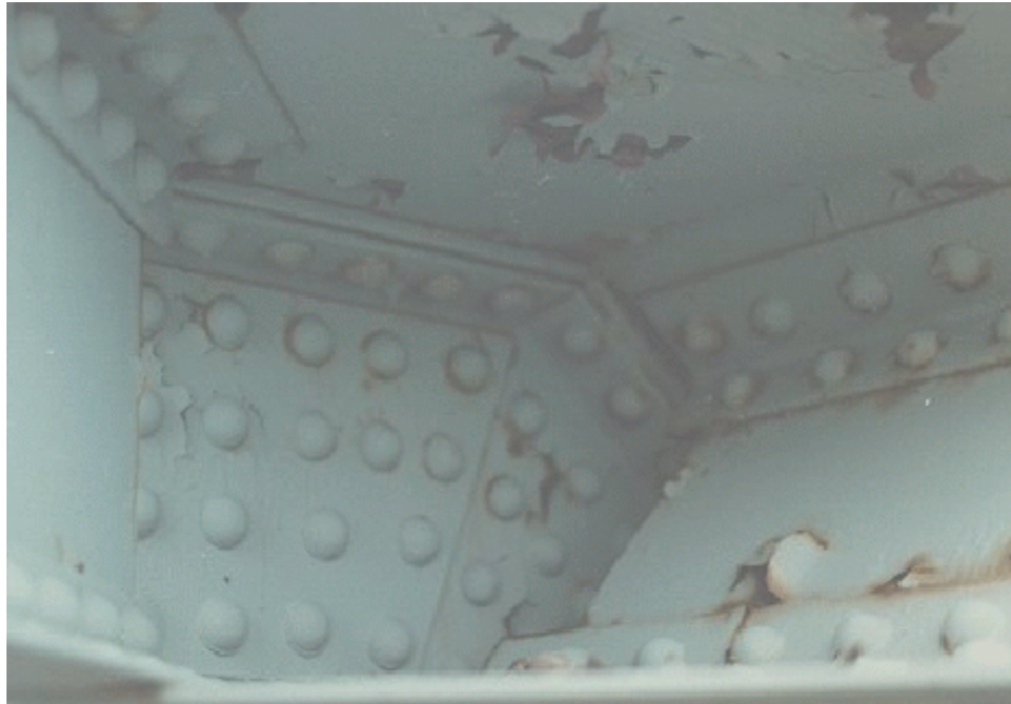
Figure A9.1.4(b) Connection of Primary Components
