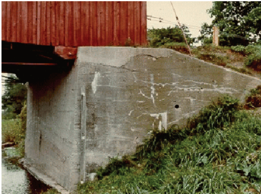
Figure A3.1.2(n) Concrete Wingwall
