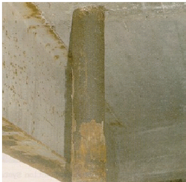
Figure A7.1.2(n) Steel Deck Drain
