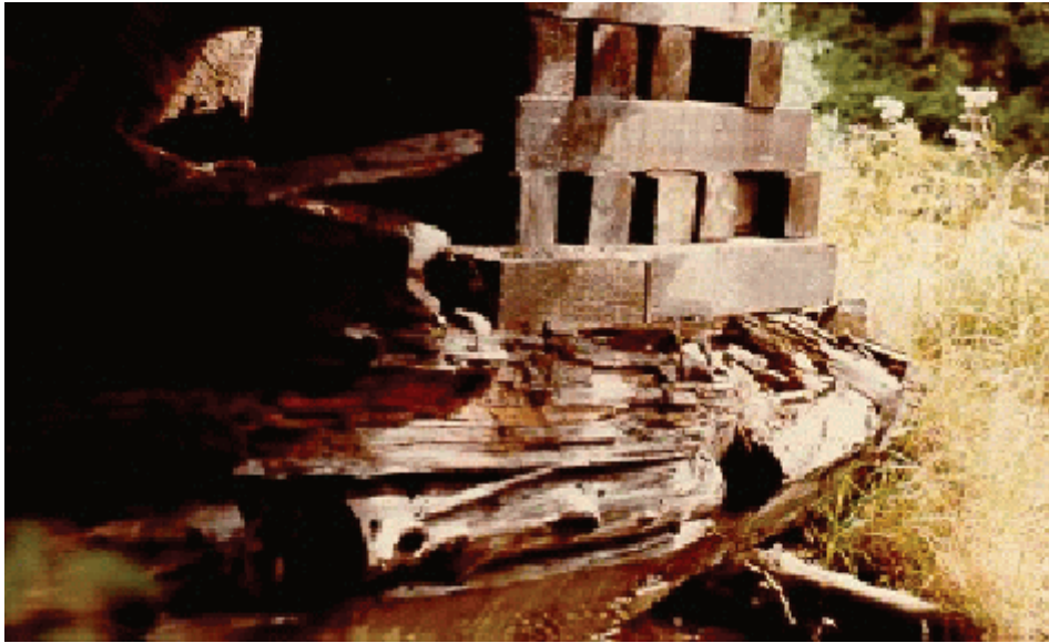
Figure A3.1.2(g) Wood Crib – Abutment Wall
