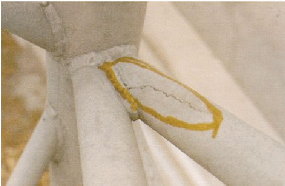
Figure 2.6.2 Wide Crack
