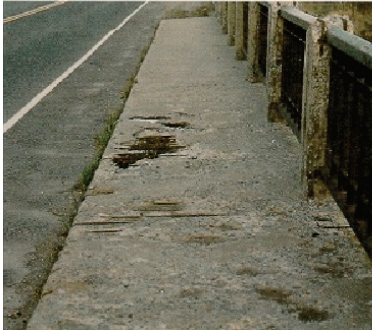
Figure A7.1.2(i) Concrete Sidewalk
