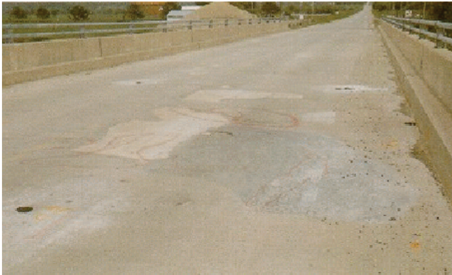
Figure A7.1.2(d) Concrete Deck
