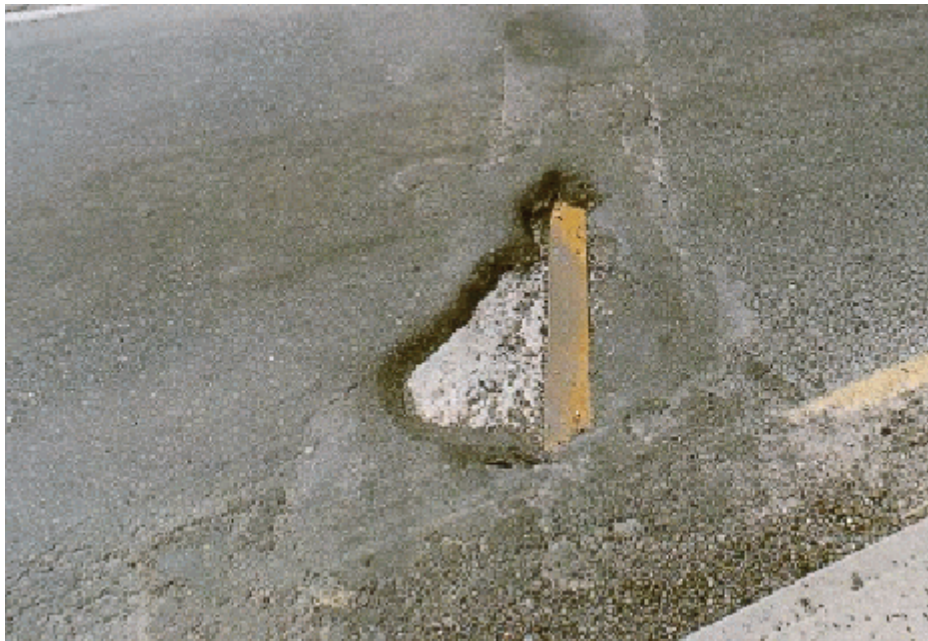
Figure 2.7.4 Severe Pothole
