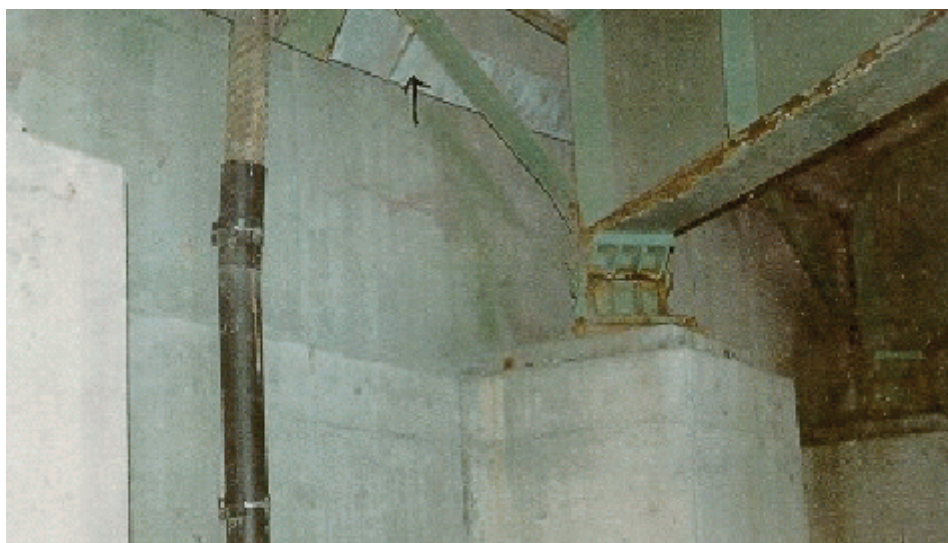
Figure A7.1.2(p) Drainage Collection System
