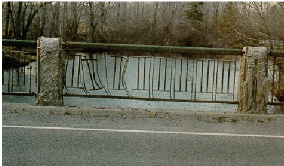
Figure A8.1.2(f) Steel Railing with Concrete Posts
