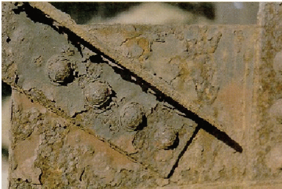
Figure A6.1.2(r) Sway Frame Connection
