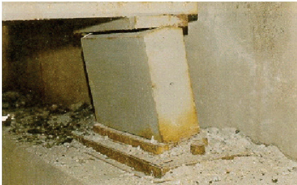
Figure A4.1.2(f) Steel Rocker Bearing
