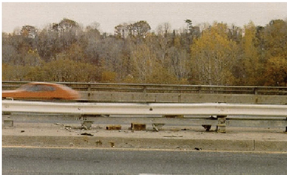
Figure A8.1.2(h) Steel Flex Beams
