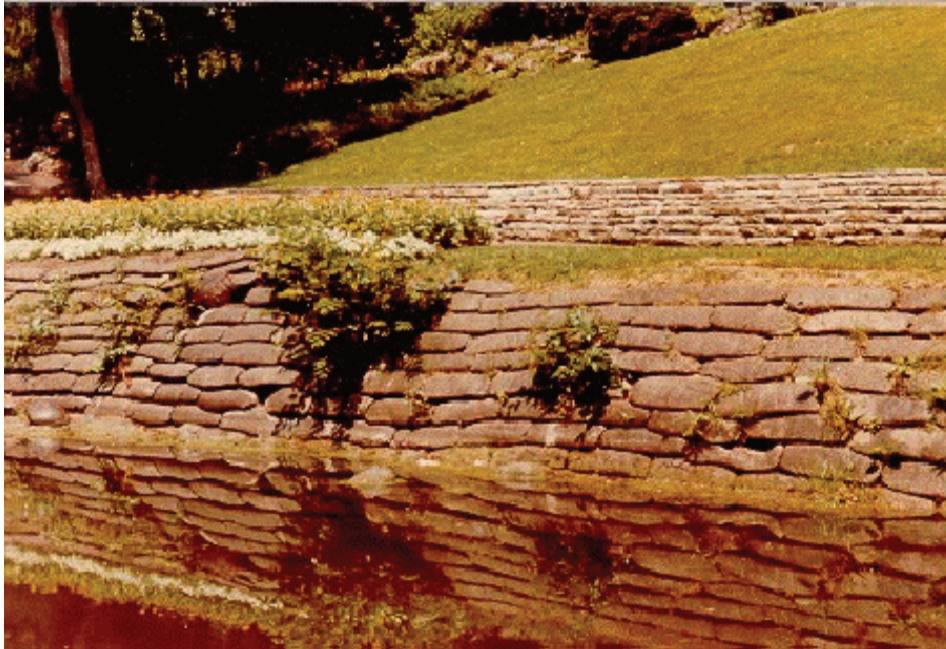
Figure A3.1.2(s) Bag Mortar Retaining Wall
