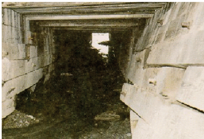
Figure A6.1.2(n) Wood Culvert
