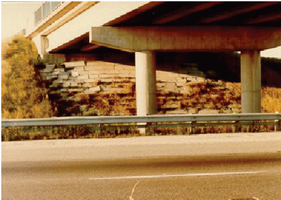
Figure A2.2.2(d) Precast Concrete Slope Protection
