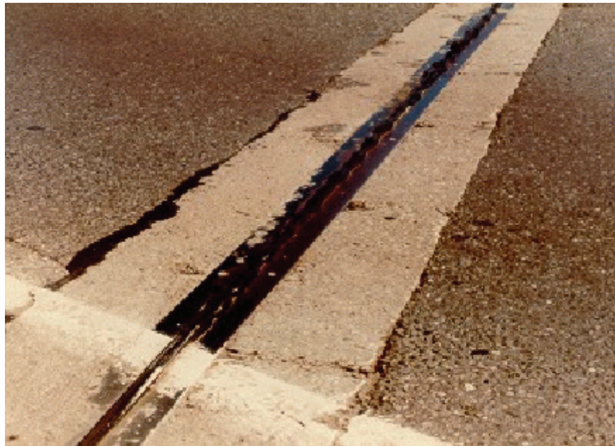
Figure A5.1.3(b) Compression Seal Joint
