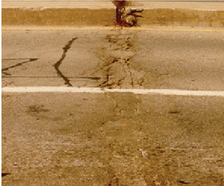
Figure A5.1.3(c) Paved-Over Joint
