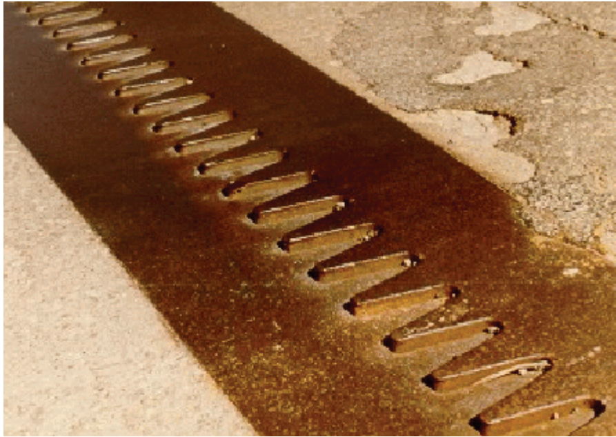
Figure A5.1.3(a) Finger Plate Expansion Joint
