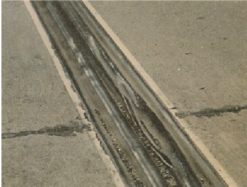
Figure A5.1.3(e) Multiple Seal Joint
