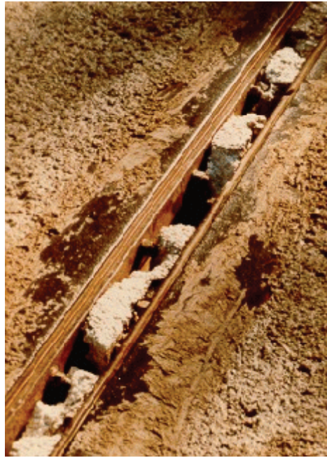
Figure A5.1.3(g) Horizontally Bolted Seal
