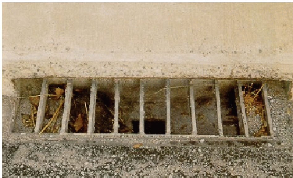
Figure A7.1.2(o) Deck Drain With Basin
