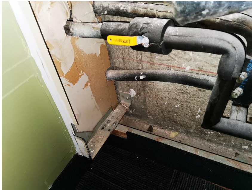
Photo 3: Drywall, sealed with asbestos containing joint compound located inside the heater units. No fungal contamination was observed.
