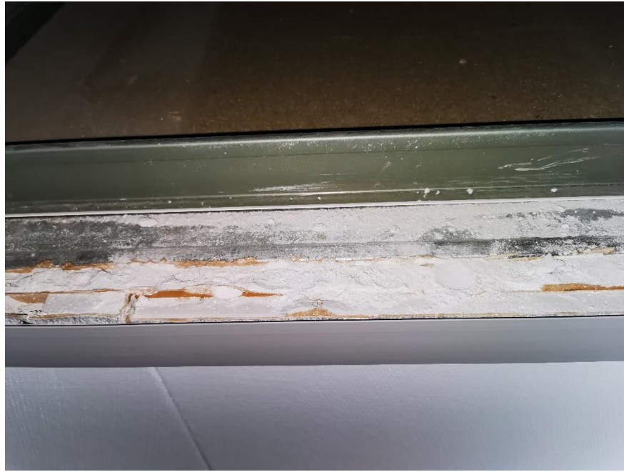
Photo 5: Wall panels were installed overtop of asbestos containing drywall materials.
