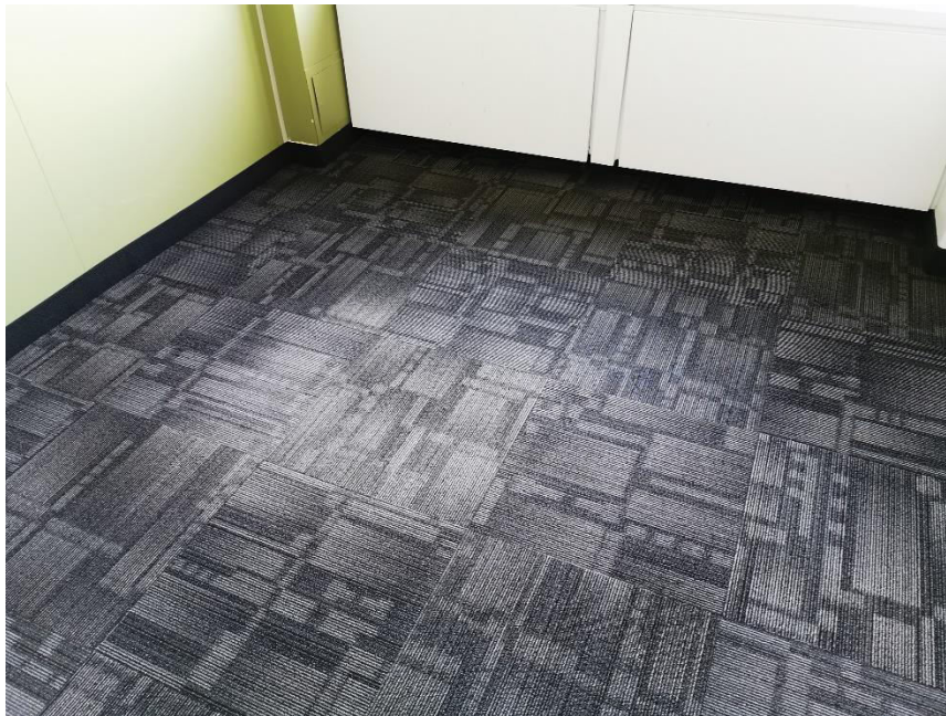
Photo 6: Flooring throughout was observed to be non-suspect carpet applied ontop of concrete subfloor.
