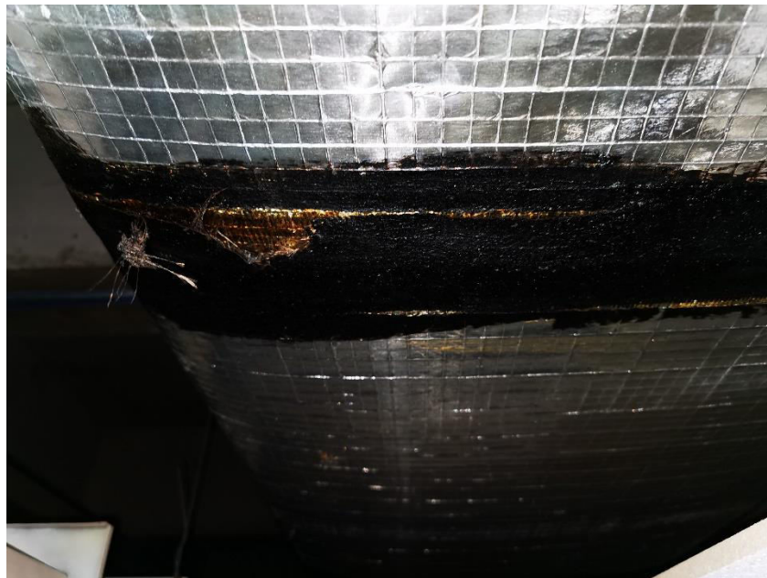
Photo 4: Asbestos containing black mastic found on insulated ducting in the ceiling space, and on mechanical lines within the heater units.
