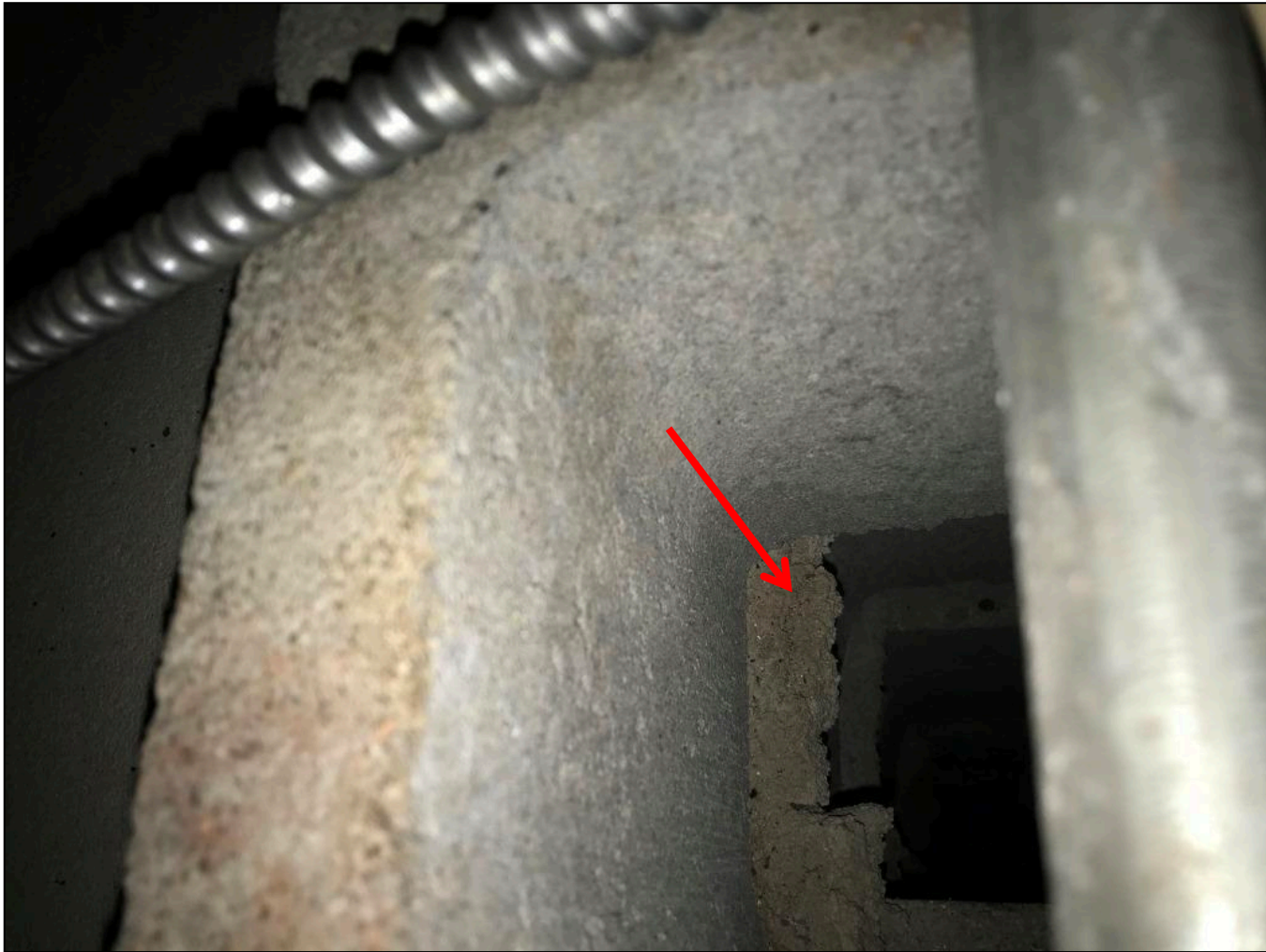
Photo 6 – View of possible vermicrete-like material inside of cinderblocks
