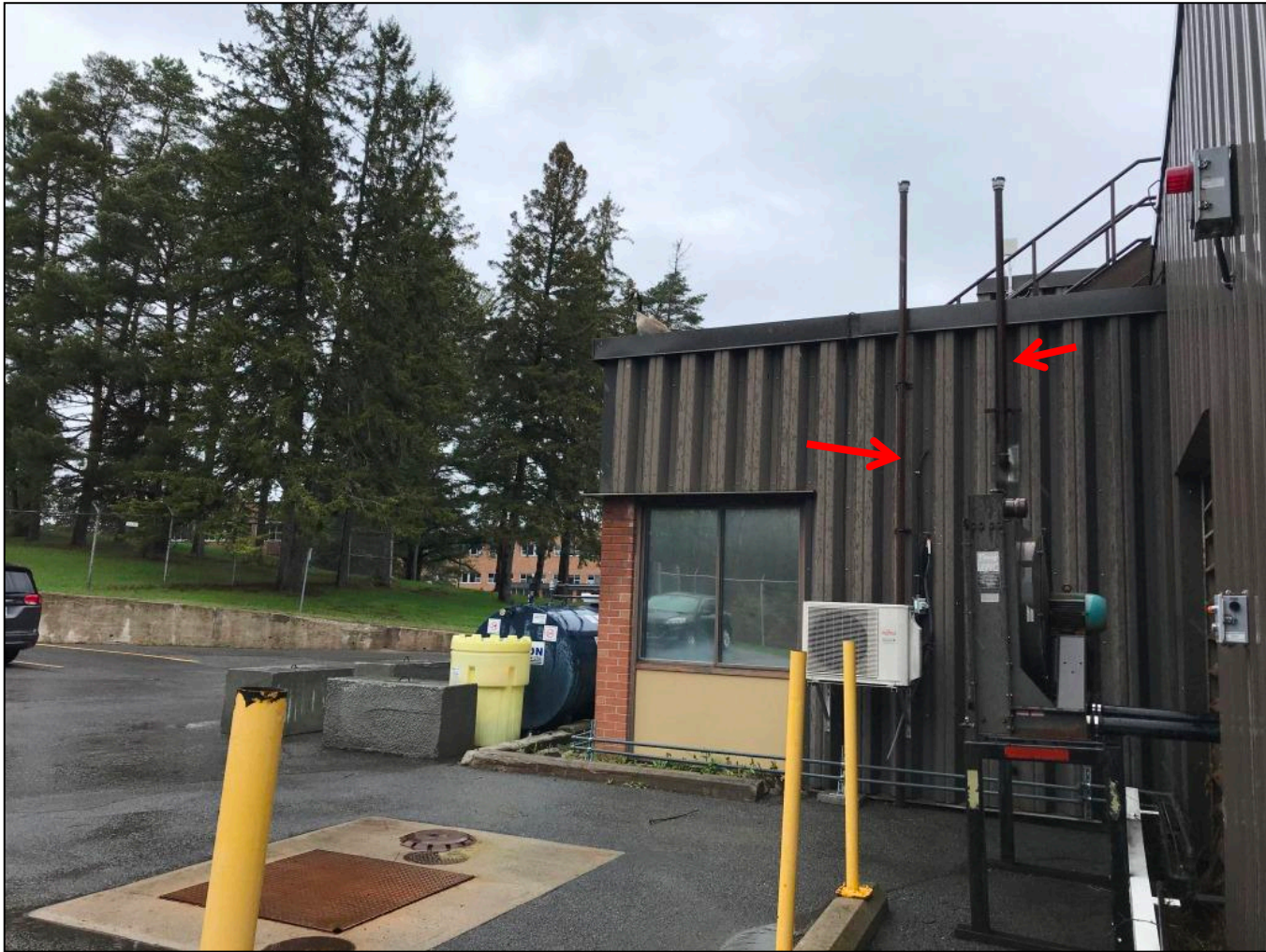
Photo 2: Exterior Piping – Brown. White Paint (Lead Containing)
