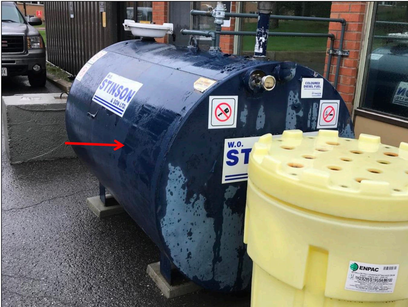
Photo 3: Exterior – Blue Paint (Low Lead Containing)
