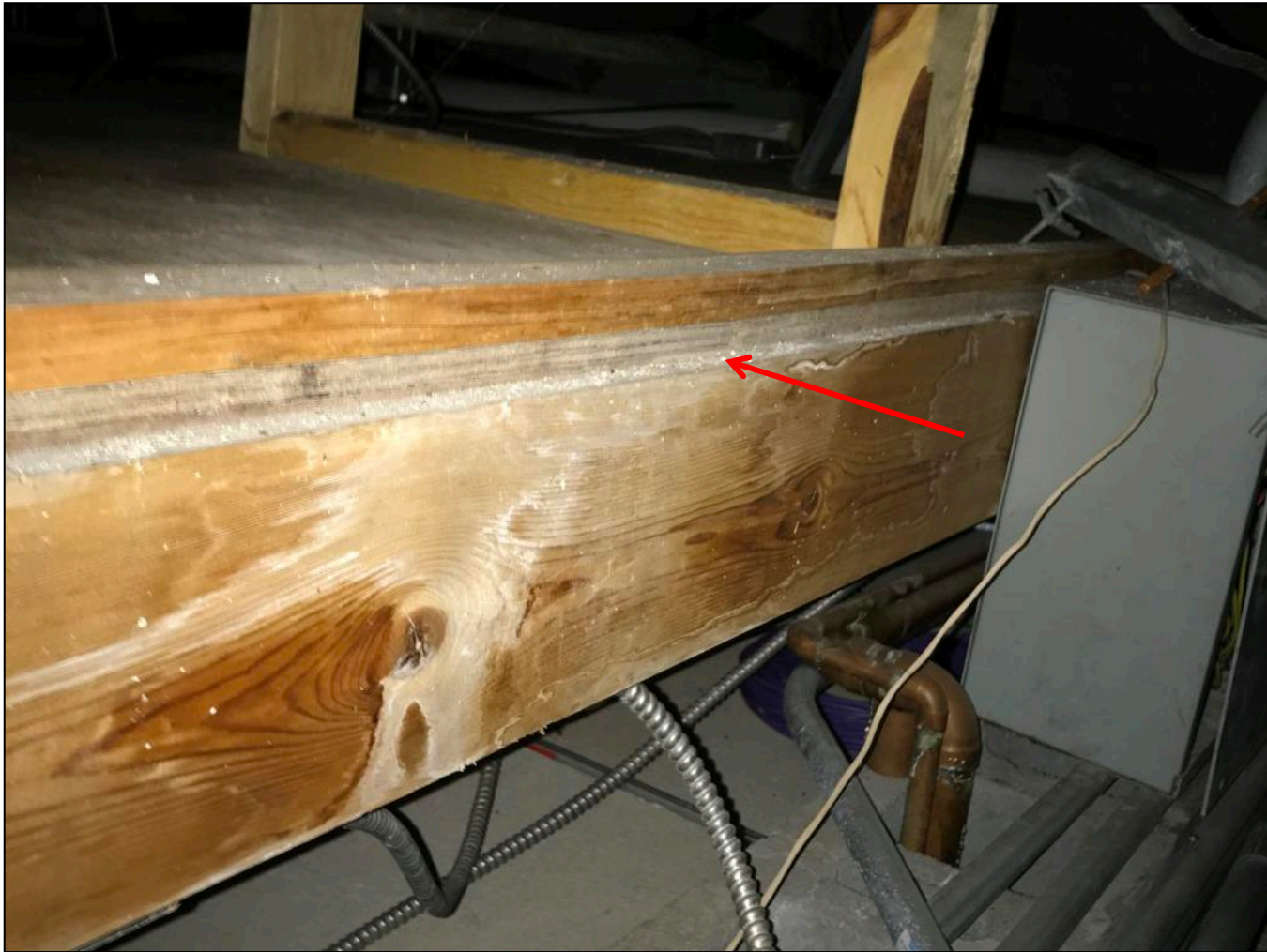
Photo 5 – View of small amounts of mortar and/or vermicrete debris on wooden shelf, above ceiling tiles (room 106)
