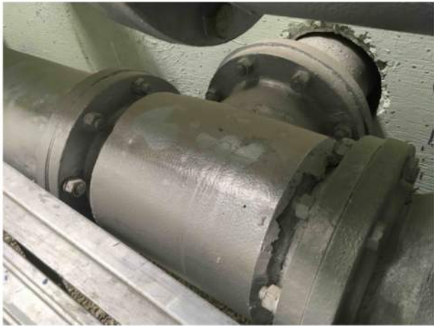
31 Pipe Asbestos sample (MSCA) — Pipe — Beige at flanged connection — Cement paste — At flanged connection — Inaccessible / Not visible — Fair — Current study sample/obs — ACM Daria.Klimenko - 2018-04-06 14:04
