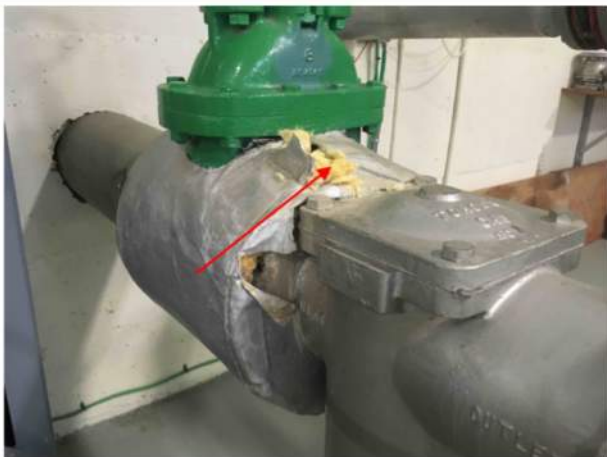
16 Pipe Asbestos sample (MSCA) — Pipe — Pipe insulation — On other pipes — Inaccessible / Not visible — Fair — Current study sample/obs — Sample under regulatory limit Daria.Klimenko - 2018-04-06 12:24
