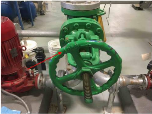
Valve Lead sample (paint) — Mechanical — Bright green paint on metal — Current study sample/obs — Sample under regulatory limit Daria.Klimenko - 2018-04-06 11:39
