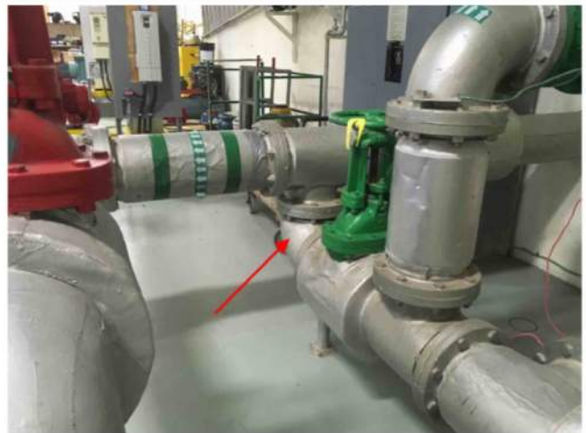
17 Pipe Asbestos sample (MSCA) — Pipe — Pipe insulation — On other pipes — Inaccessible / Not visible — Fair — Current study sample/obs — Observation Daria.Klimenko - 2018-05-18 14:09
