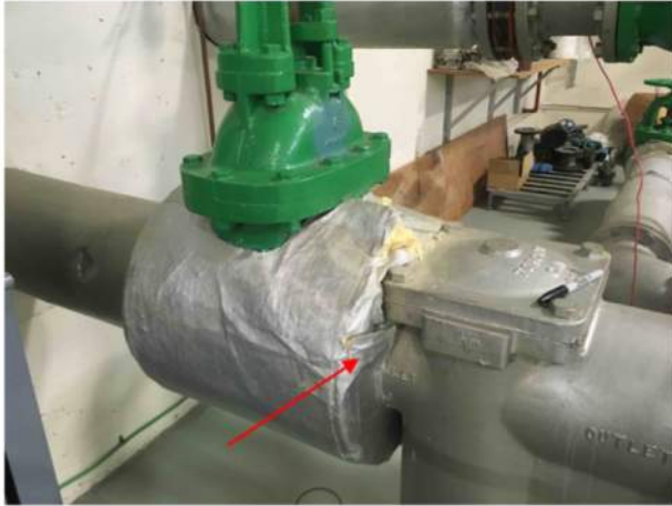
12 Pipe Asbestos sample (MSCA) — Pipe — Joint tape compound — At elbows and flanged connection — Accessible / Visible — Fair — Current study sample/obs — Sample under regulatory limit Daria.Klimenko - 2018-04-06 12:01
