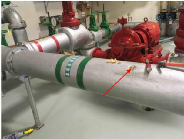
20 Pipe Asbestos sample (MSCA) — Pipe — Pipe insulation — On other pipes — Inaccessible / Not visible — Fair — Current study sample/obs — Sample under regulatory limit Daria.Klimenko - 2018-04-06 12:52
