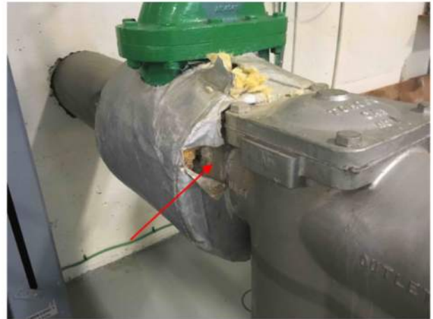
15 Pipe Asbestos sample (MSCA) — Pipe — At flanged connection — Cement paste — Elbows and flanged connection — Inaccessible / Not visible — Poor — Current study sample/obs — ACM presumed Daria.Klimenko - 2018-04-06 12:23
