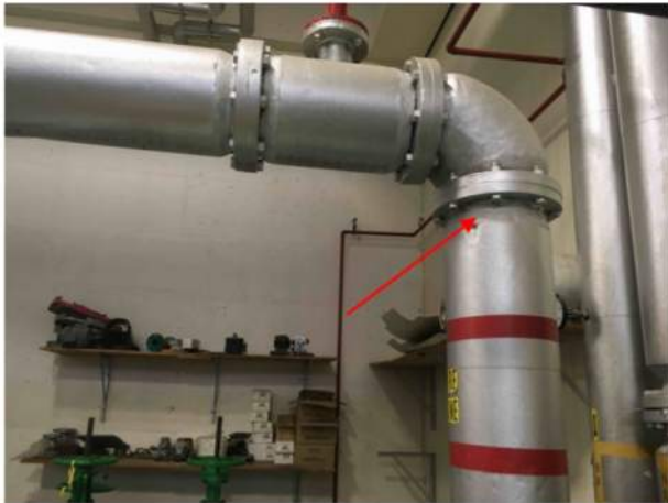
14 Pipe Asbestos sample (MSCA) — Pipe — At flanged connection — Cement paste — At elbows and flanged connection — Accessible / Visible — Fair — Current study sample/obs — ACM Daria.Klimenko - 2018-04-06 12:04
