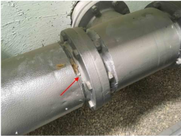
31 Pipe Asbestos sample (MSCA) — Pipe — Beige at flanged connection — Cement paste — At flanged connection — Inaccessible / Not visible — Fair — Current study sample/obs — ACM Daria.Klimenko - 2018-04-06 14:03
