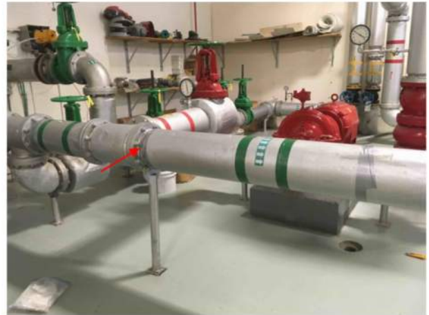
21 Pipe Asbestos sample (MSCA) — Pipe — At flanged connection — Cement paste — Elbows and flanged connection — Inaccessible / Not visible — Poor — Current study sample/obs — ACM presumed Daria.Klimenko - 2018-04-06 12:59
