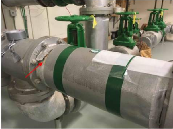
18 Pipe Asbestos sample (MSCA) — Pipe — At flanged connection — Cement paste — Elbows and flanged connection — Inaccessible / Not visible — Poor — Current study sample/obs — ACM presumed Daria.Klimenko - 2018-04-06 12:40
