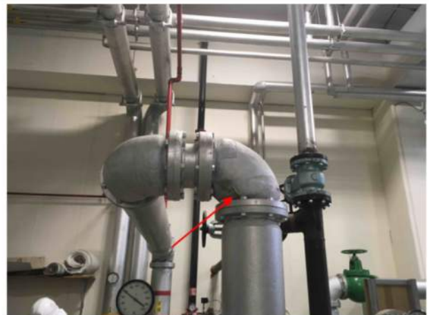
23 Pipe Asbestos sample (MSCA) — Pipe — Elbow — Joint tape compound — At elbows and flanged connection — Accessible / Visible — Fair — Current study sample/obs — Sample under regulatory limit Daria.Klimenko - 2018-04-06 13:05
