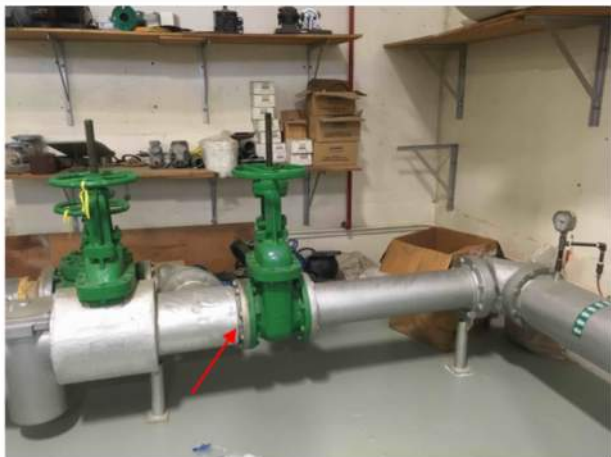
27 Pipe Asbestos sample (MSCA) — Pipe — At flanged connection — Cement paste — Elbows and flanged connection — Inaccessible / Not visible — Poor — Current study sample/obs — ACM presumed Daria.Klimenko - 2018-04-06 13:29
