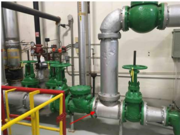
25 Pipe Asbestos sample (MSCA) — Pipe — At flanged connection — Cement paste — Elbows and flanged connection — Inaccessible / Not visible — Fair — Current study sample/obs — ACM Daria.Klimenko - 2018-04-06 13:17
