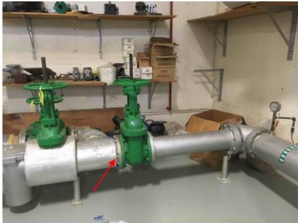
24 Pipe Asbestos sample (MSCA) — Pipe — At flanged connection — Cement paste — Elbows and piping — Inaccessible / Not visible — Fair — Current study sample/obs — ACM presumed Daria.Klimenko - 2018-04-06 13:09
