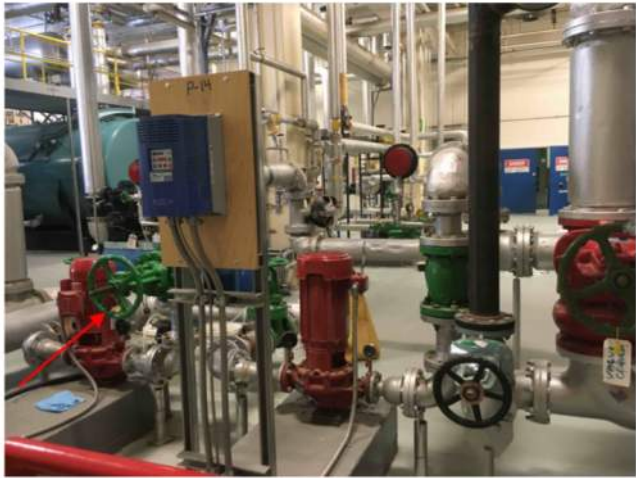
Valve Lead sample (paint) — Mechanical — Bright green paint on metal — Current study sample/obs — Sample under regulatory limit Daria.Klimenko - 2018-04-06 11:39
