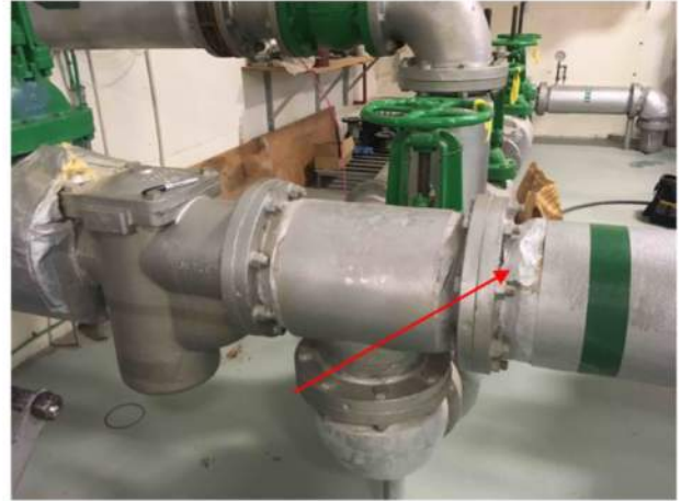
13 Pipe Asbestos sample (MSCA) — Pipe — Joint tape compound — At elbows and flanged connection — Accessible / Visible — Poor — Current study sample/obs — Sample under regulatory limit Daria.Klimenko - 2018-04-06 12:01
