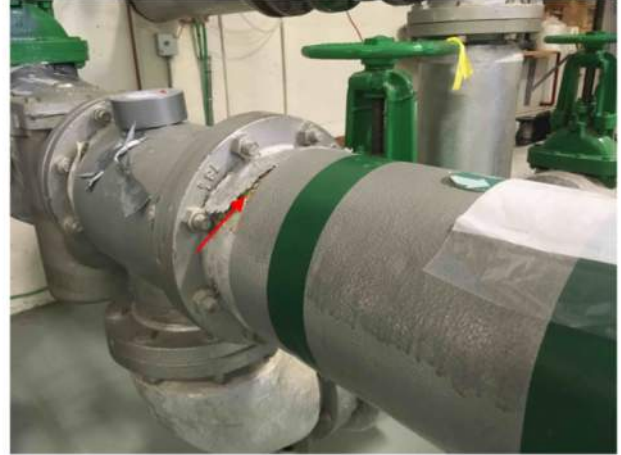
19 Pipe Asbestos sample (MSCA) — Pipe — Pipe insulation — On other pipes — Inaccessible / Not visible — Fair — Current study sample/obs — Sample under regulatory limit Daria.Klimenko - 2018-04-06 12:40
