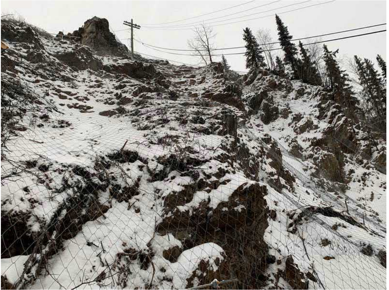
Photograph 6: View looking up slope showing mesh area.
