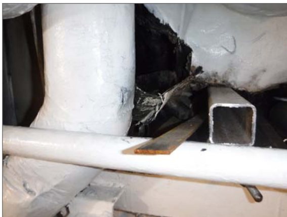
Client identified lagging compound and suspect insulation.
