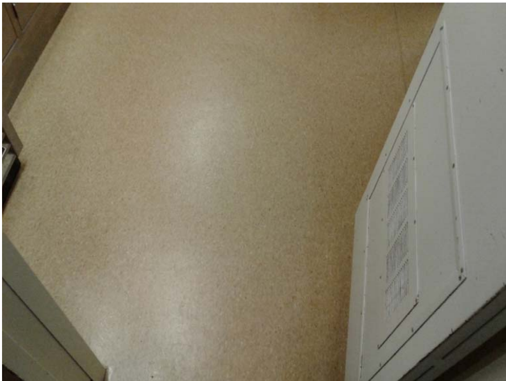
Vinyl Sheet Flooring, New install, , Crew's Mess (Loc. 21)
