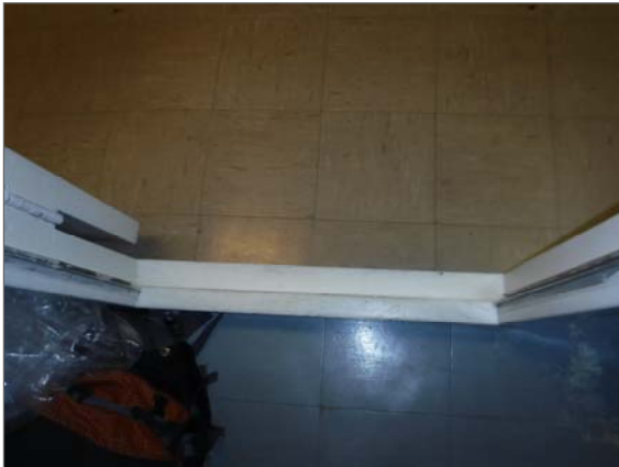
Asbestos-containing 9"x9" beige vinyl floor tiles; depicting painted and not painted conditions.
