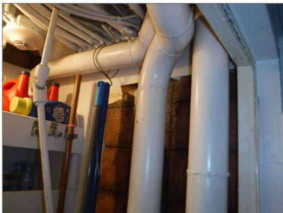
Uninsulated piping Utility and Dry storage Area (Location 16)
