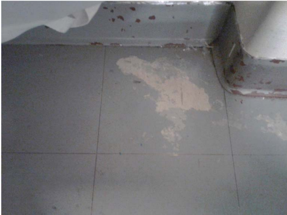
Vinyl Floor Tile and Mastic, In closet 9x9 grey painted brown with brown streak, V9000, Corridor (Loc. 3)
