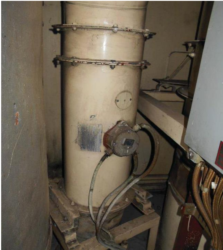
Figure 16.3-10: Photograph of in-situ MCR supply axial fan (SF-4)
