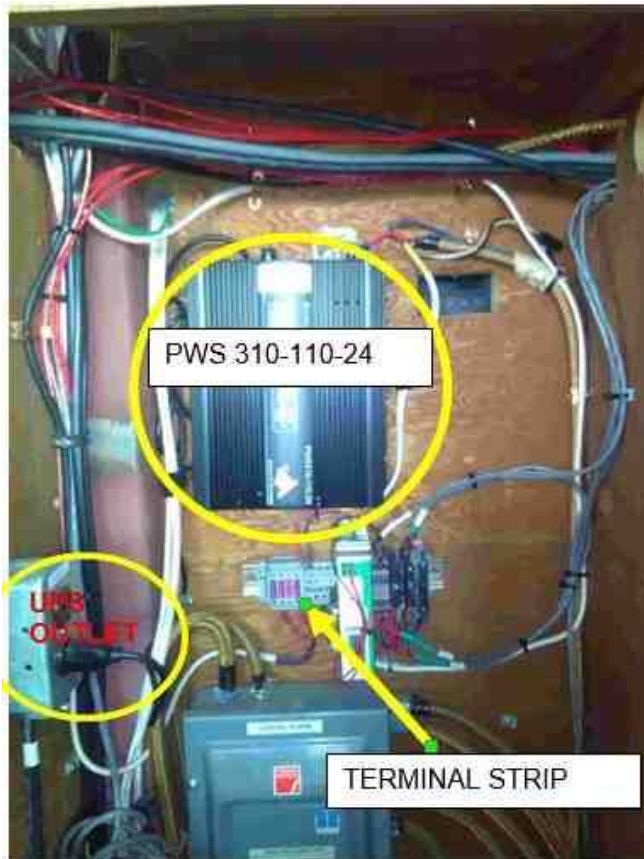
Figure 17.4-4: 24v Power Supply – Chart table
