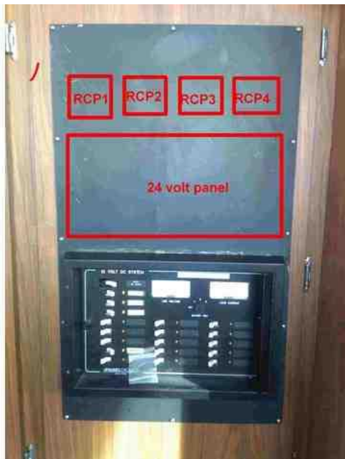
Figure 17.4-21: Proposed 24V Power distribution and RPC location
