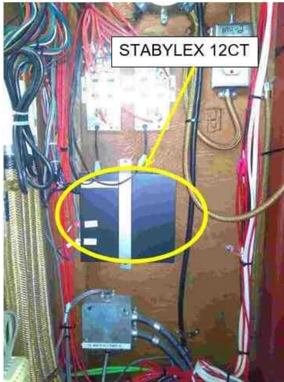
Figure 17.4-1: Stabylex Power Supply Location
