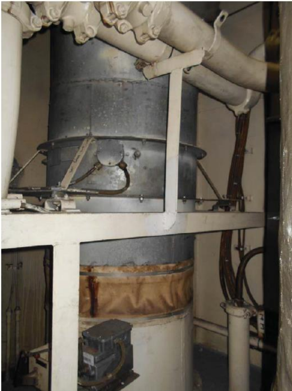
Figure 16.3-2: Photograph of in-situ engine room exhaust axial fan (EF-7 or EF-8)
