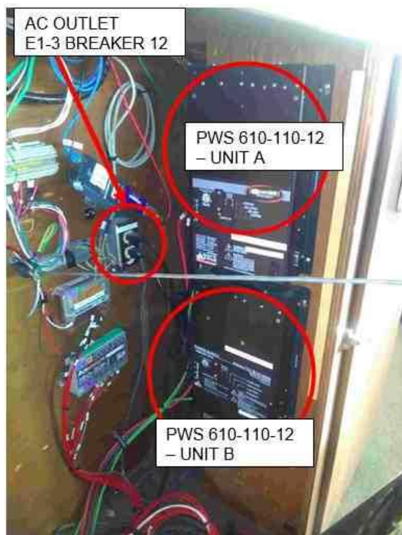
Figure 17.4-16: Current 12V Power supplies location
