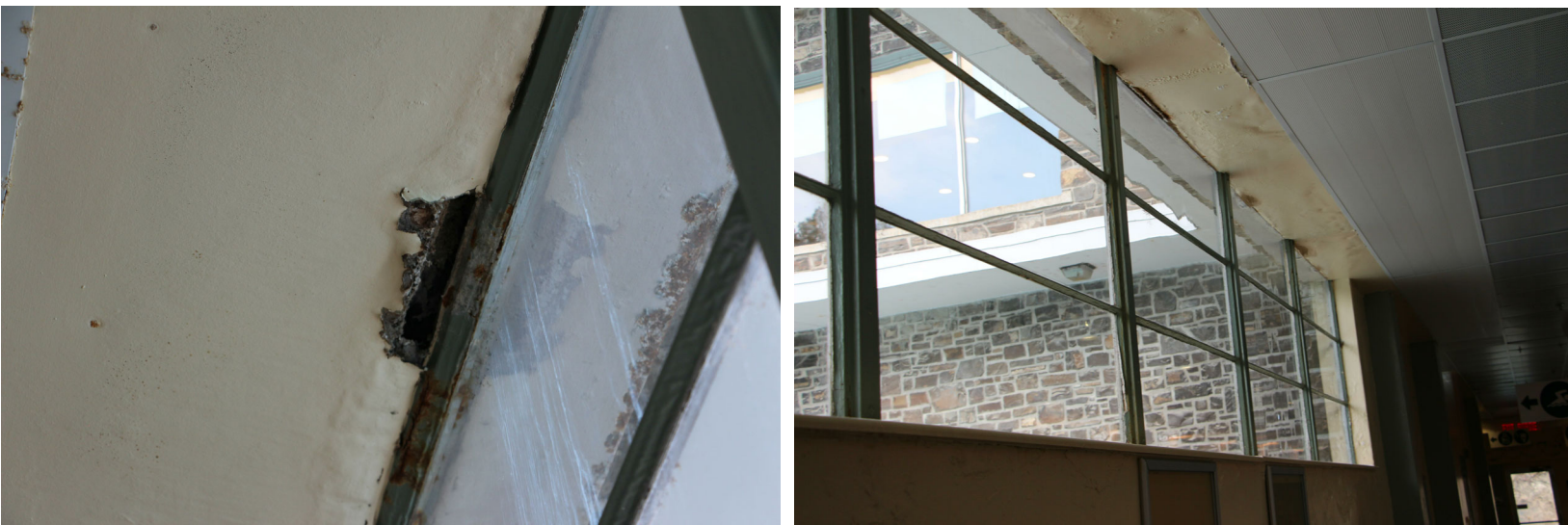
TYP. HEAD CONDITION @ MAIN FLOOR POOL COORIDOR. REMOVE EXISTING DAMAGED DRYWALL
