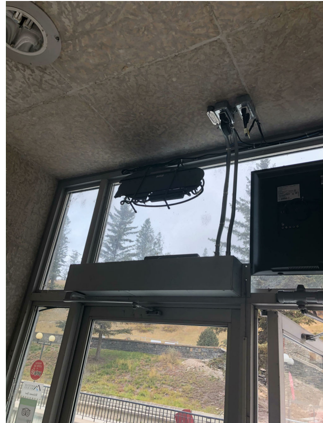
IMG.34. EXISTING AUTOMATIC DOOR OPERATOR AT MAIN ENTRANCE, SECOND FLOOR
