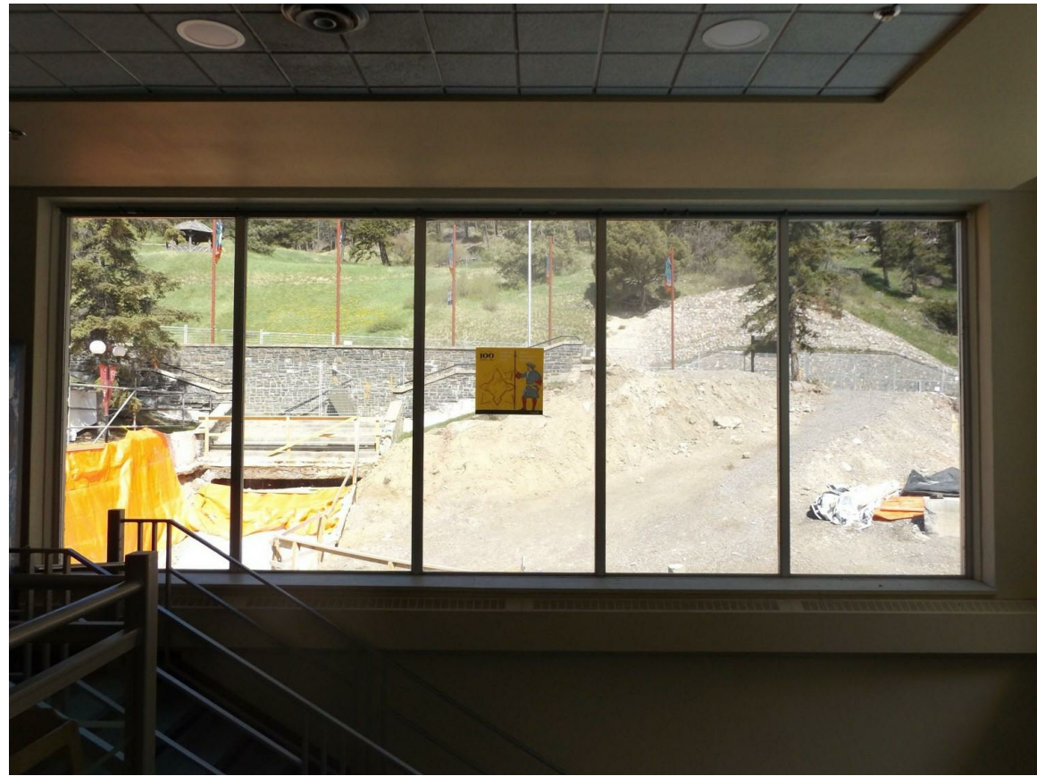
IMG.23. LOBBY CORNER WINDOW. MIDDLE PANEL BEING REPLACED
