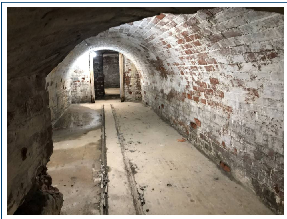
PHOTO 2 — East to West Tunnel, showing white paint in poor condition (note how the condition of the paint varies)
