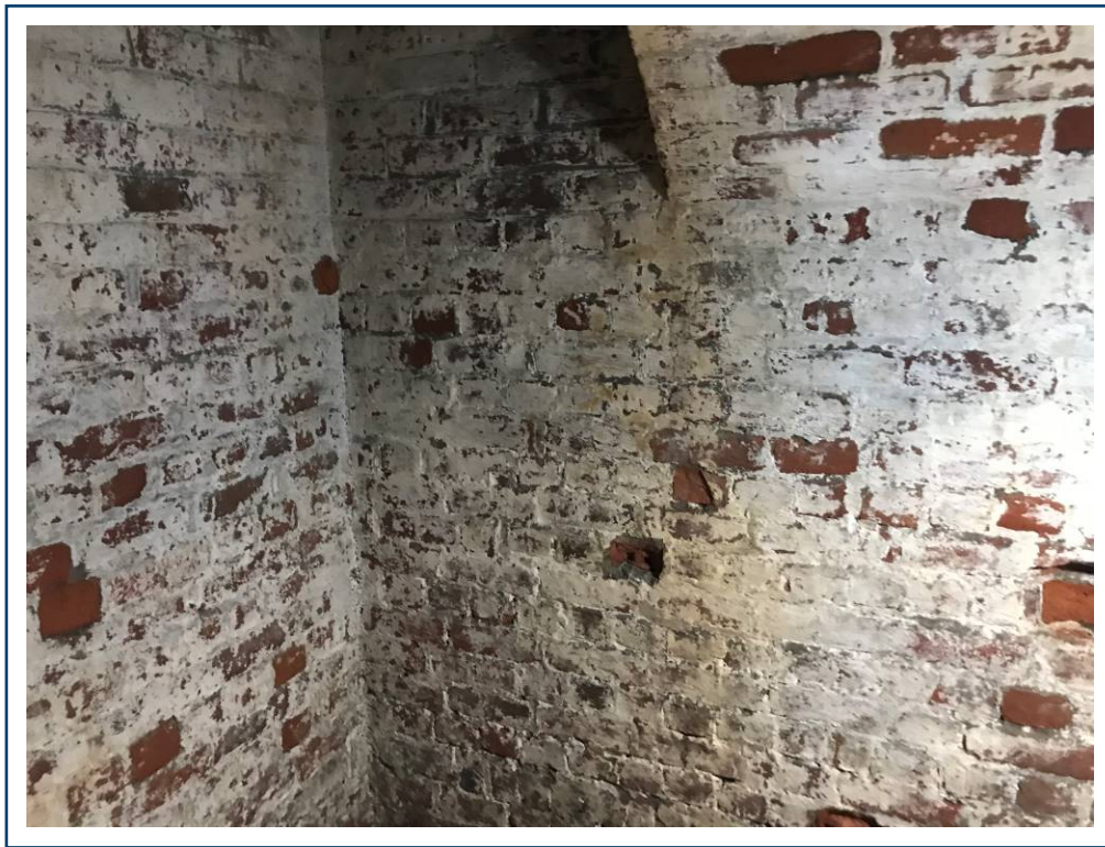
PHOTO 1 — East to West Tunnel, showing white paint in poor condition (note how the condition of the paint varies)
