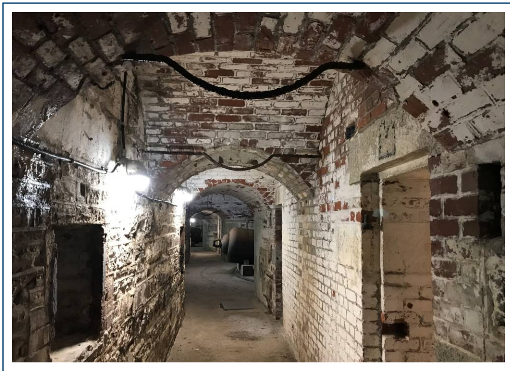
PHOTO 4 — Lower Battery South showing white paint in poor condition (note how the condition of the paint varies)
