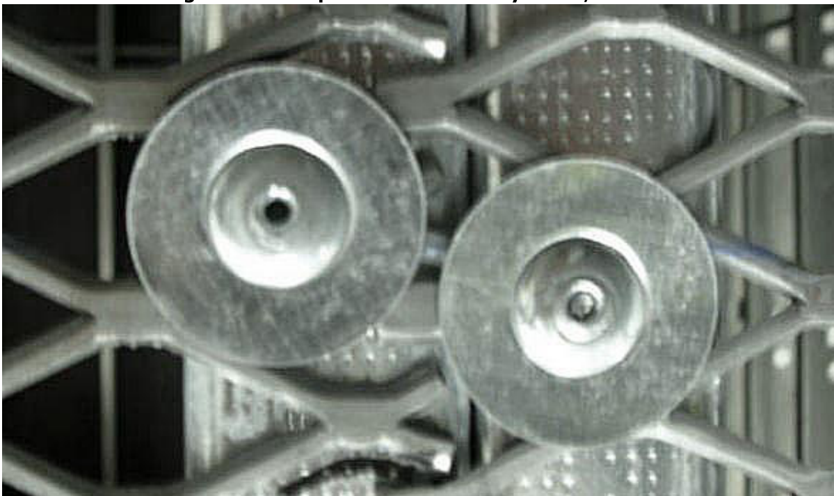
Figure 5: Example of Mesh Interlay Seam, Riveted
