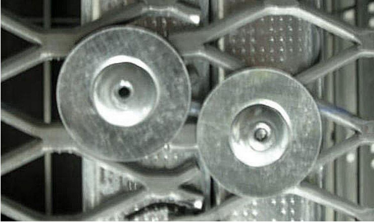
Figure 5: Example of Mesh Interlay Seam, Riveted
