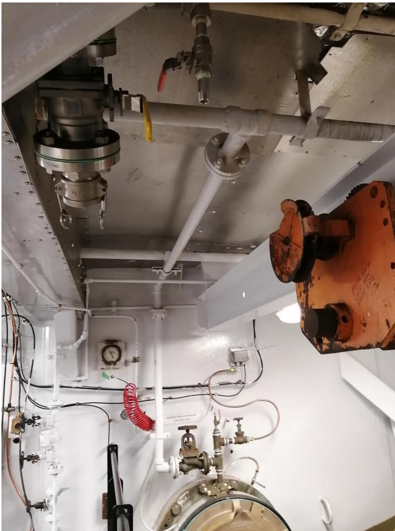
Existing CW line to port stern tube
