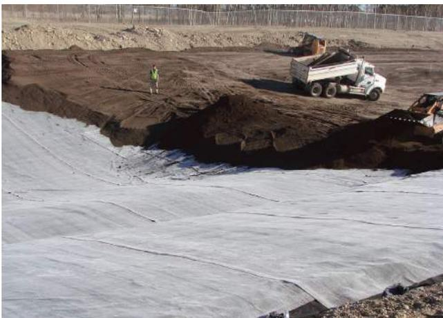
GCL's provide an excellent alternative to conventional compacted clay liners by replacing a thick section of compacted clay with a thin layer of pure sodium bentonite. One truckload of GCL is equivalent to 150 truckloads of compacted clay. Benefits include easy installation, better hydraulic performance, and resistance to varying weather conditions.
