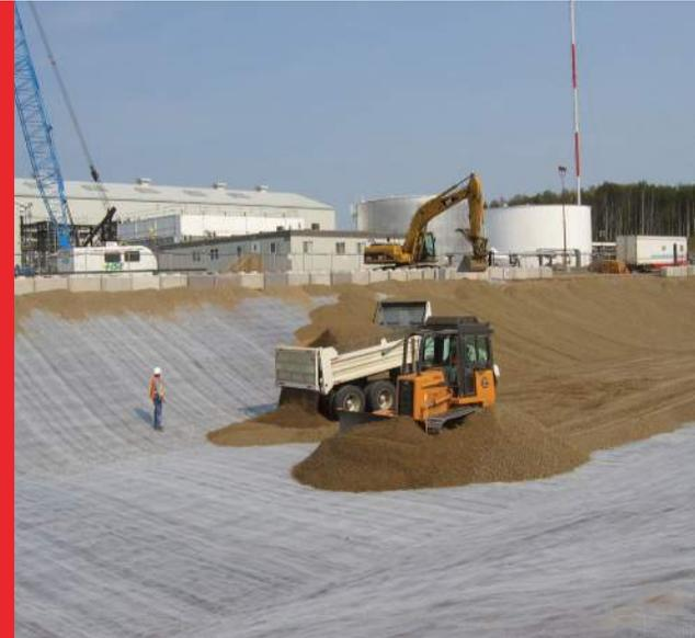
Geosynthetic Clay Liners (GCL's) are high performance environmental liners used in environmental containment applications. GCL's consist of two layers of geotextiles surrounding a layer of low permeability sodium bentonite that are needle punched together to increase internal shear resistance. The geotextiles offer a long lasting resistance to physical or chemical break-down in harsh elements, while the bentonite's high swelling capacity and low permeability provide an effective hydraulic seal.
