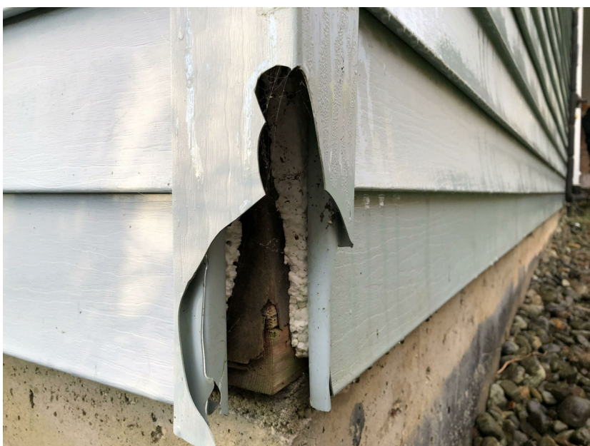
9 TYP. VINYL SIDING / EPS SUBSTRATE A300
