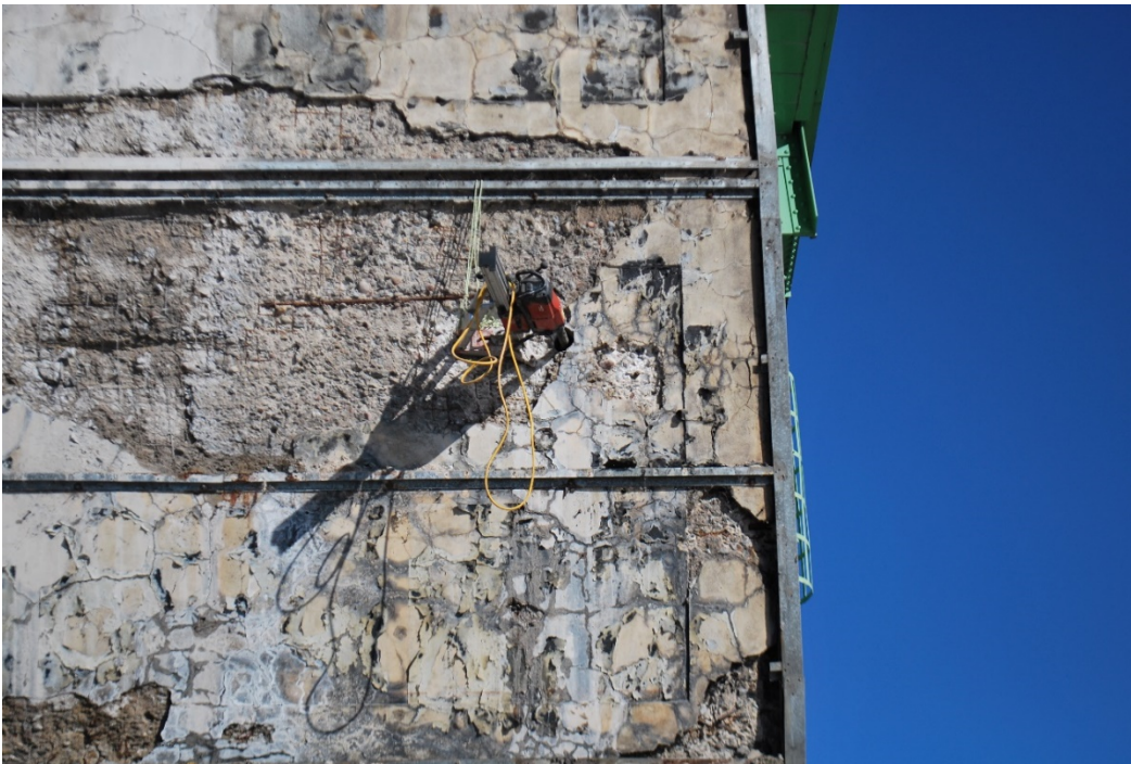
Figure A10 – Concrete core location C2 on West face.
