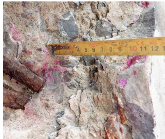
Figure 4-12: Zone indicated by red box in Figure 4-11 (North East bottom corner of East face).
