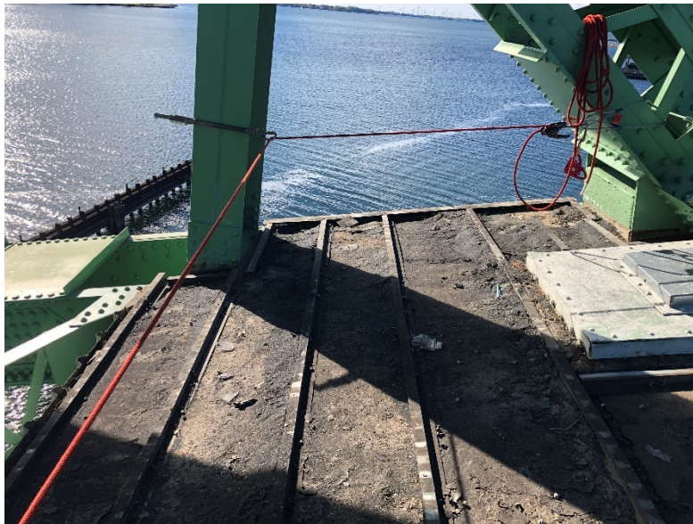
Figure 3-4: Rope access on top of Counterweight
