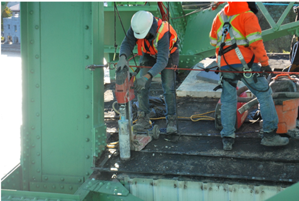
Figure A20 – Coring location C6 (South East corner of top face).
