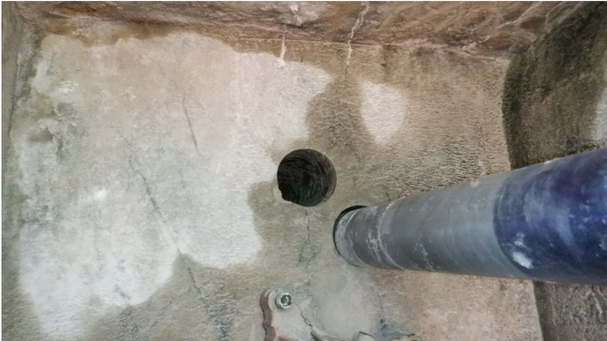
Figure A27 – Core holes C3 (left) and C4 (right) inside North compartment on East face. Please refer to the compartments in Figure A22.
