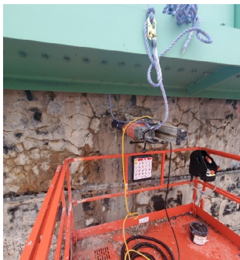
Figure 3-3: Hilti coring machine mounted on Counterweight (core location C1 shown)
