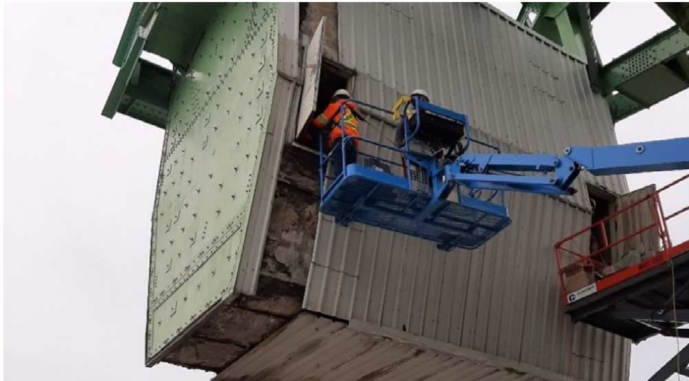
Figure 4-13: Workers inspecting South compartment on East face
