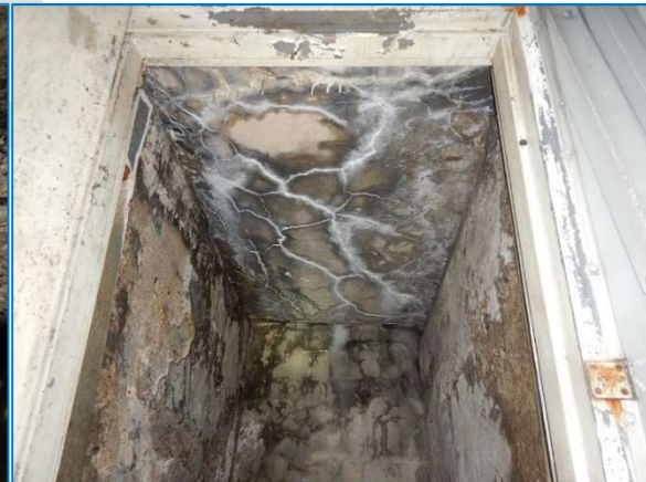
Photo 4 Chamber - South East
