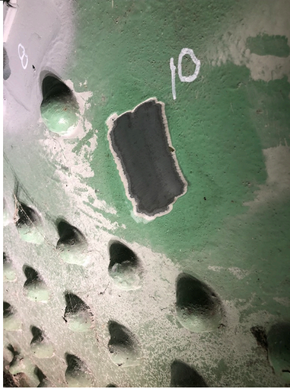
Figure4: Test Location 10 at North Trunnion Plate Exterior Plate (Readings Taken from Inside surface of Plate)
