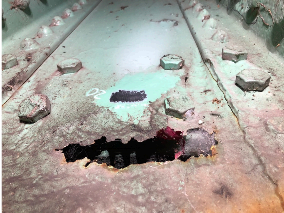
Figure5: Test Location 20 at North Trunnion Location, Batten Plate
