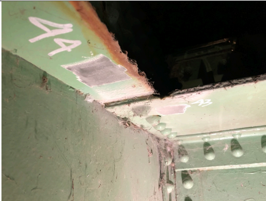
Figure11: Test Locations 43 and 44 at South Trunnion Exterior Plate at Interior Batten Plate and Angle
