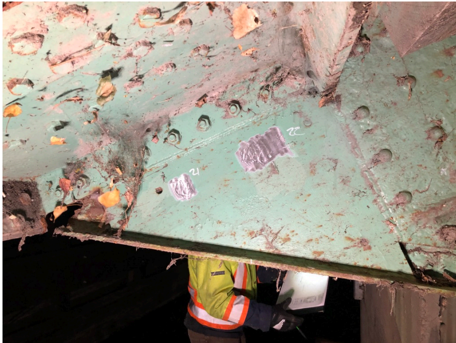
Figure6: Test Locations 21 and 22 at South Trunnion Plate Interior Location (Readings Taken on Exterior Plate Surface)
