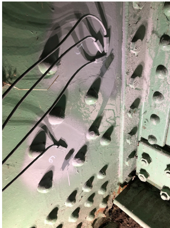
Figure1: Test Locations 5 and 6 at North Trunnion Plate Interior Plate at Strain Gauge Locations (Readings Taken from Inside surface of Plate)
