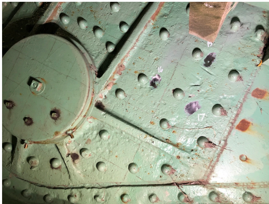
Figure4: Test Locations 15, 16, and 17 at North Trunnion Plate Interior Plate
