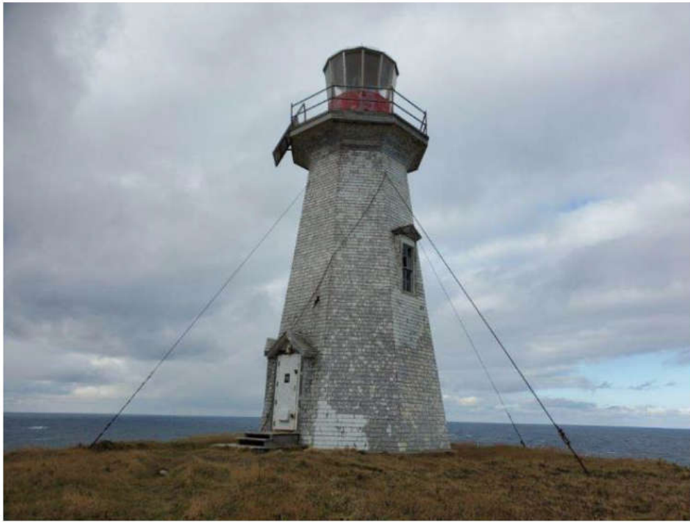
Figure 1: Photo of the Brion Island lighthouse
