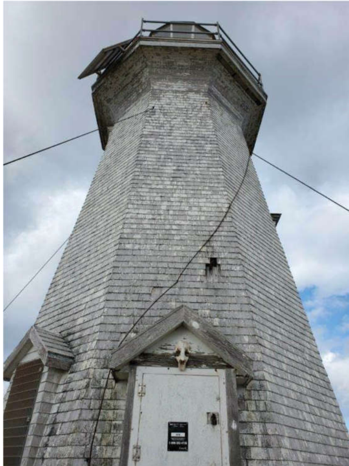
Anchoring of the shrouds on the lighthouse and wooden facing of the lighthouse
