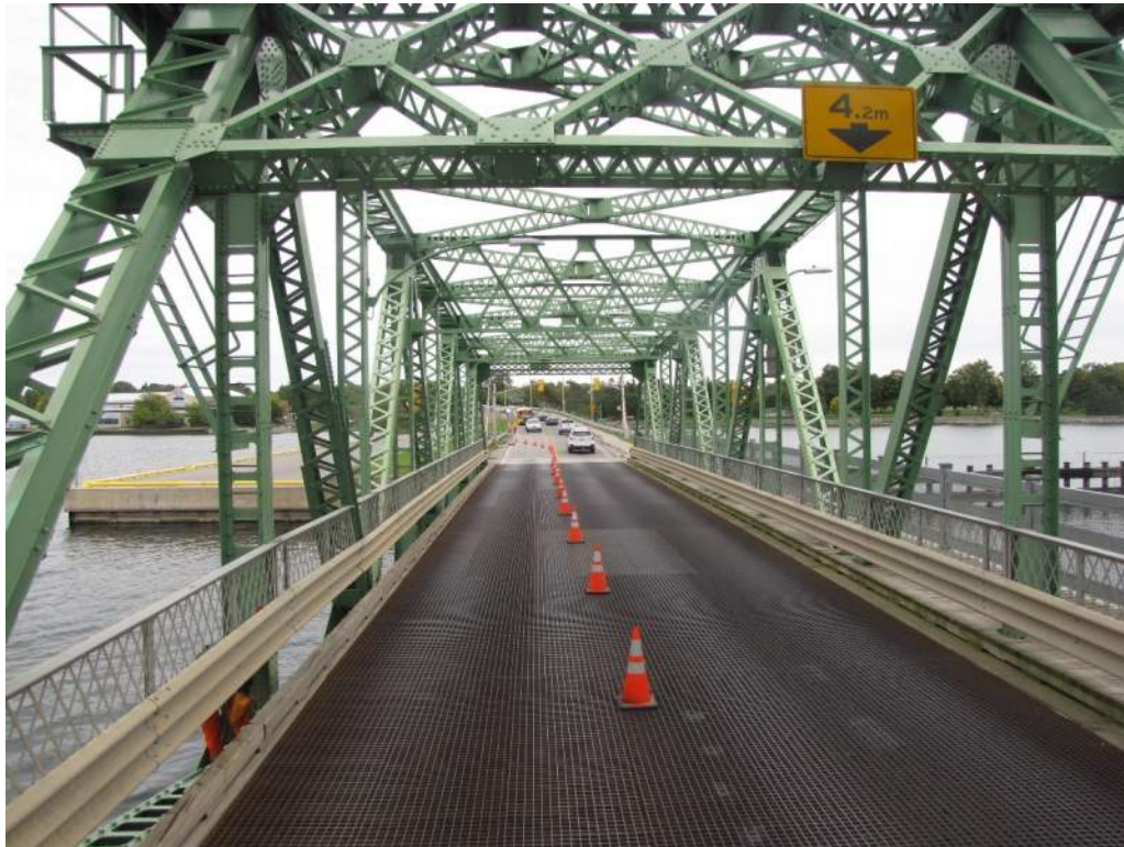
Photo S4: Looking east.
