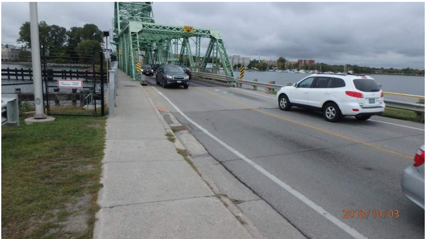
Photo S111: The east end of the east approach slab appears to have settled over time creating an uneven ride for vehicles.
