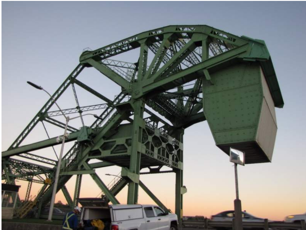
Photo S6: North side of the counterweight truss.
