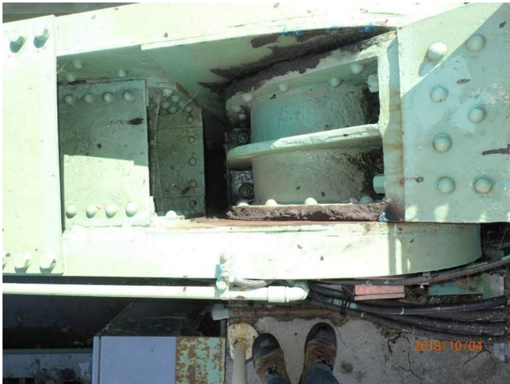
Photo S89: View of the top of the north trunnion.
