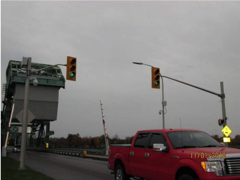
Photo E25: Typical Traffic Signal (West Shown). Each bridge approach is provided with two sets of traffic signal fixtures mounted on cantilevered arms and suspended over the roadway. Additionally, a warning gong and a pedestrian signal light have been provided at each of the south traffic signal poles. The traffic signal equipment was installed as part of a recent rehabilitation project and is in excellent condition.
