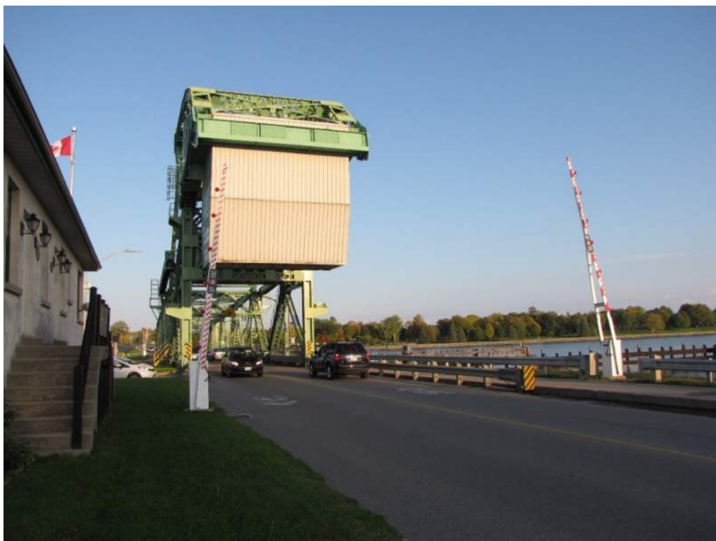
Photo S7: West approach, looking east.
