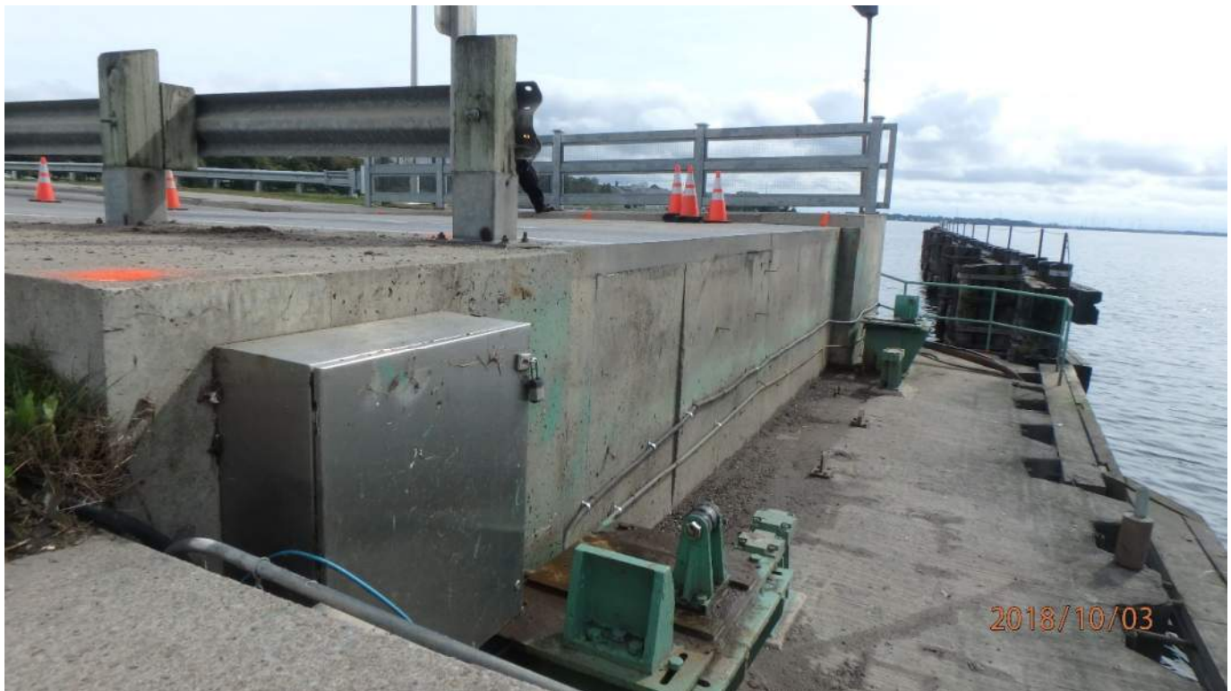
Photo S10: East abutment, looking south.
