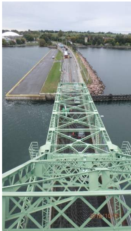
Photo S3: Top of truss, looking east.
