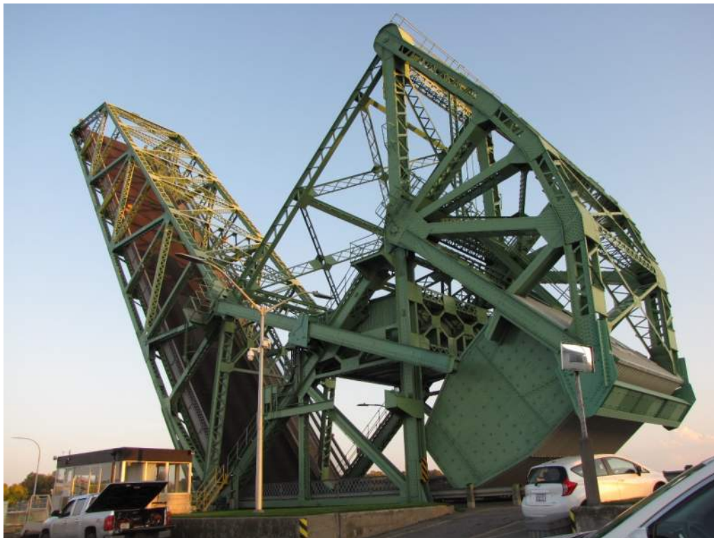
Photo S5: Bridge in open position.
