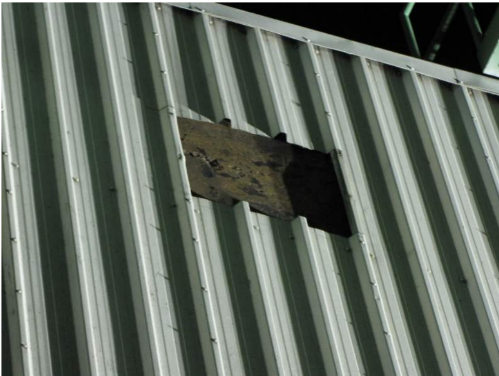
Photo S79: The counterweight concrete in the upper northwest corner exhibits wide cracks.
