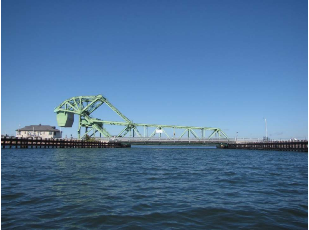
Photo S1: South elevation.
