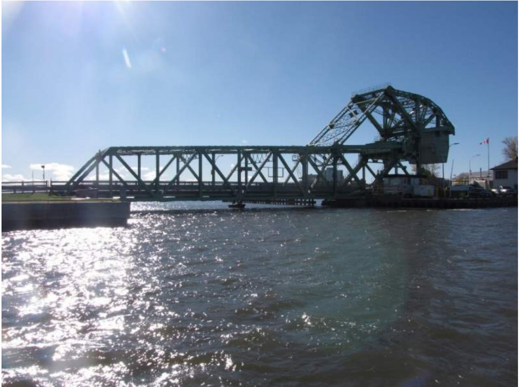
Photo S2: North elevation (photo from 2017 inspection).
