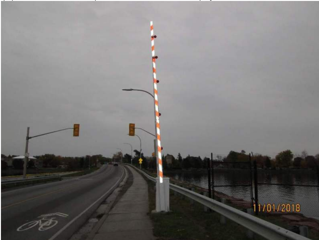
Photo E26: Typical Traffic Gate (Fully Raised). The bridge is provided with four (4) traffic gates, one at each approach to the span. All gates and gate arm lights were in good operational condition at the time of the inspection.
