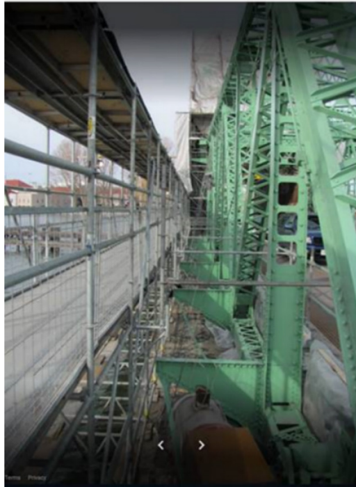
Figure 8 - Temporary removal of the sidewalk (photo from 2010 rehabilitation)
