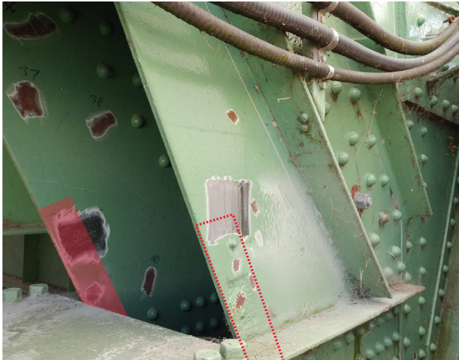
Figure 20 - Gusset Plate Strengthening Type B
