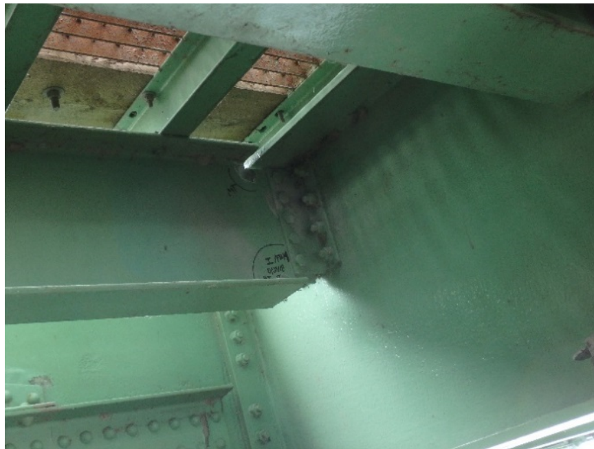
Figure 3: Potential Distortion-Induced Fatigue Detail
