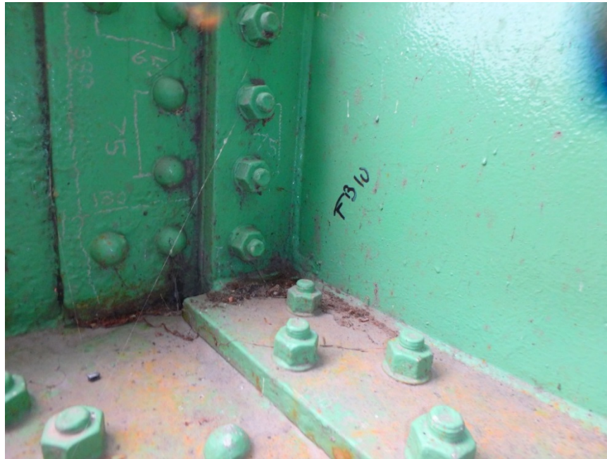
Figure 4: Potential Constraint-Induced Fatigue Detail
