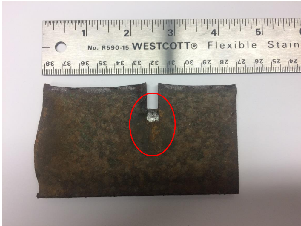
Photo 19: Crack in bearing bar propagating from notch in sample taken from piece that failed.
