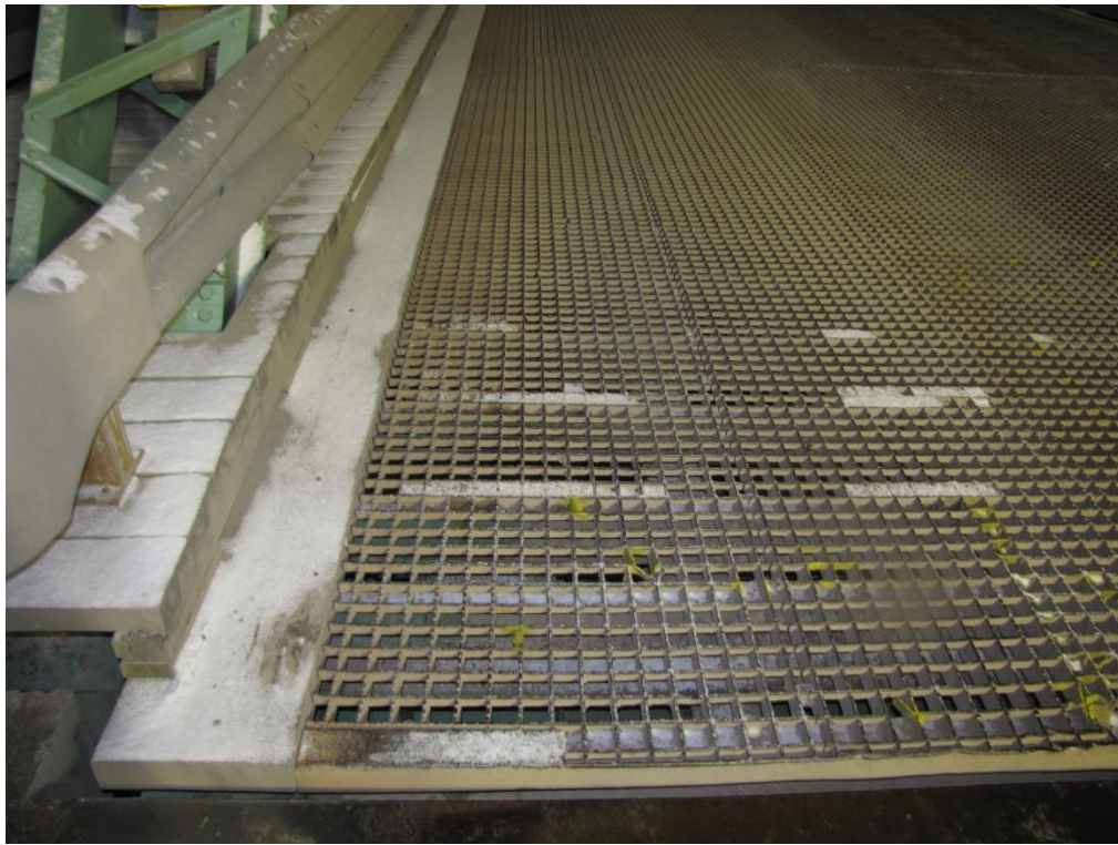
Photo 9: Armouring at south side at east abutment.
