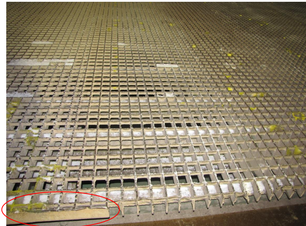
Photo 10: End cross-bar terminates 2.2 metres from the south curb.
