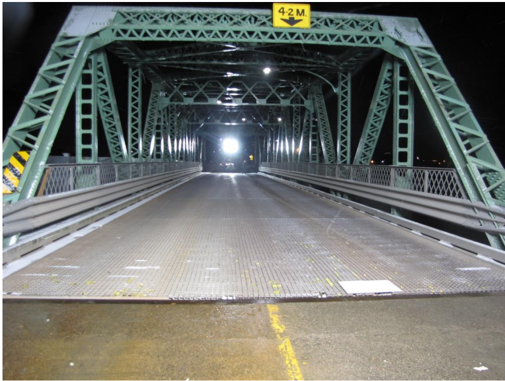
Photo 1: General view of the steel grating on the Bascule bridge looking from the east approach.
