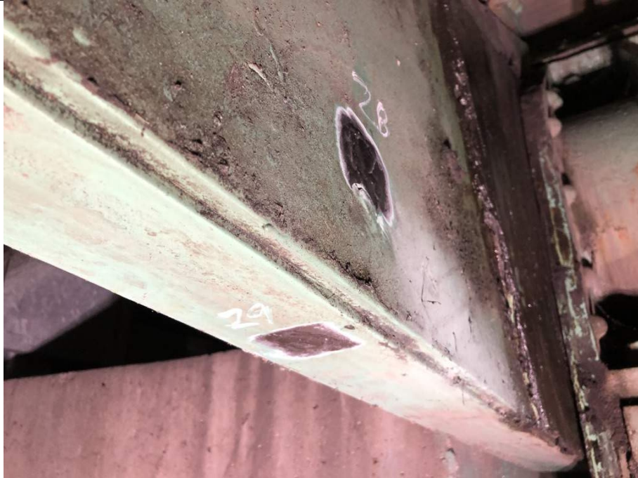
Figure9: Test Locations 28 and 29 at South Trunnion Plate Exterior Location (Readings Taken from Inside Surface and Bottom Surface of Angle)
