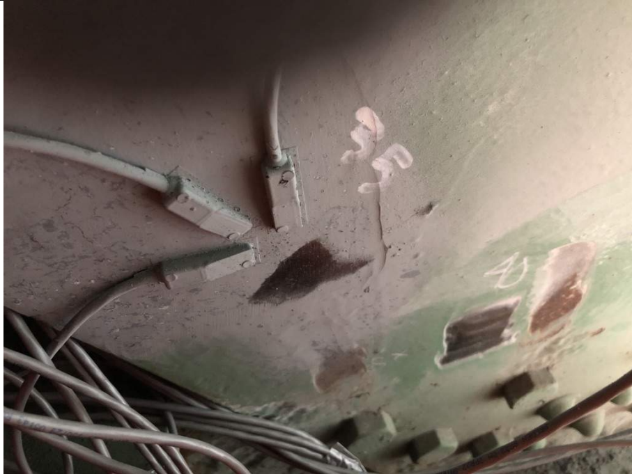
Figure15: Test Locations 35, and 40 at South Trunnion Exterior Plate Location (Readings Taken on Interior Surface of Plate)
