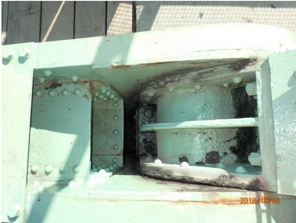
Photo 19: View of the top of the south trunnion (15S).
