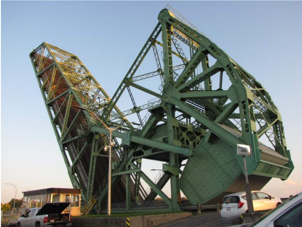
Photo 3: Bridge in open position.
