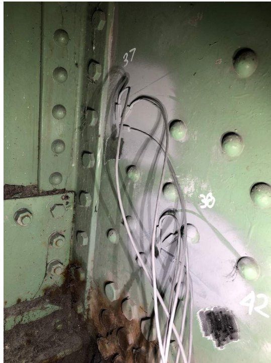
Figure14: Test Locations 37, 38, and 42 at South Trunnion Interior Plate Location (Readings Taken on Interior Surface of Plate)
