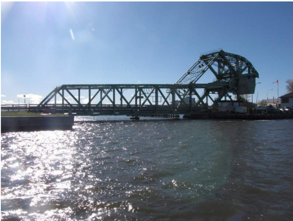
Photo 2: North elevation (2017 photo).
