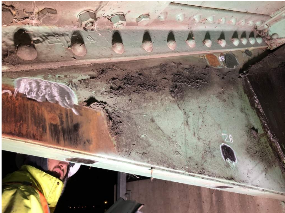
Figure8: Test Locations 25, 26 and 28 at South Trunnion Plate Exterior Location (Readings Taken from Inside Surface)
