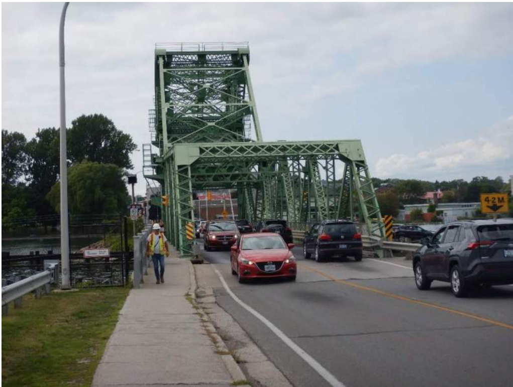
Photo S-6: East approach, looking west.
