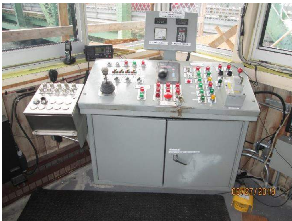
Photo E-18: Control Desk. The location of the control desk provides the operator with a complete view of the channel and vehicular and pedestrian roadway traffic. The control desk is in acceptable condition. Note the foot switch next to the control desk on the floor is in good operational condition.
