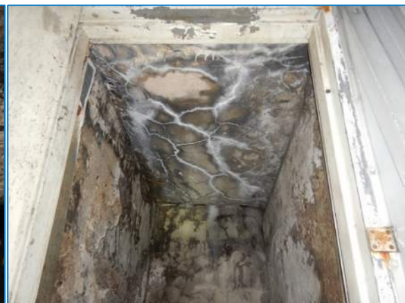
Photo 4 Chamber - South East
