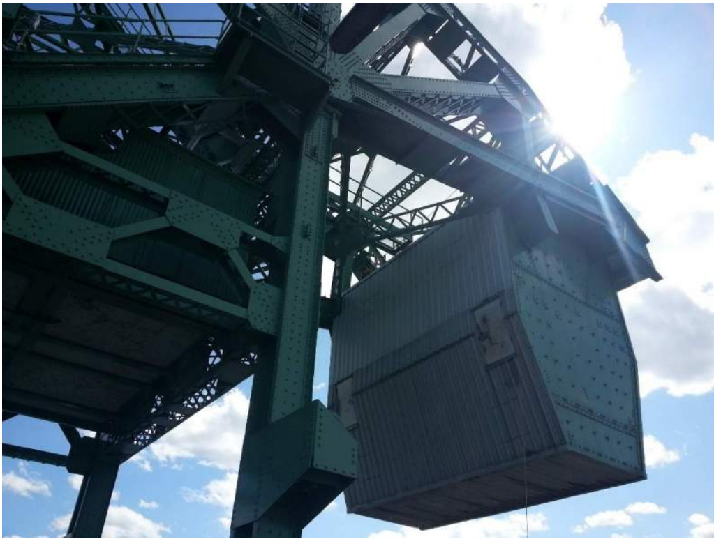
Photo S-8: North side of the counterweight and counterweight truss.
