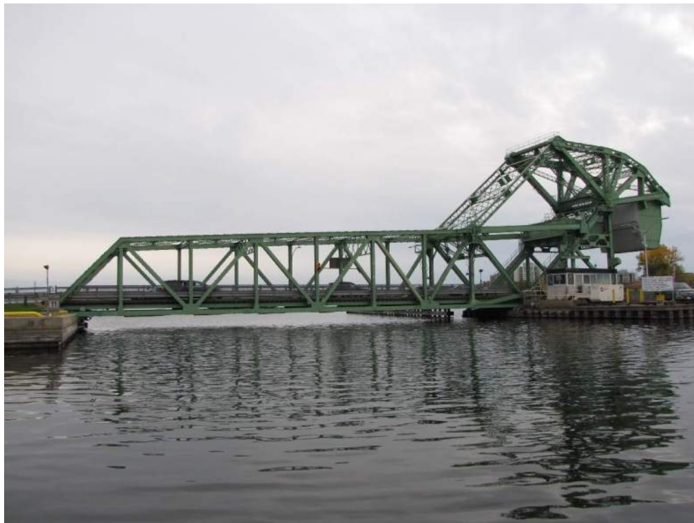
Photo S-2: North elevation.
