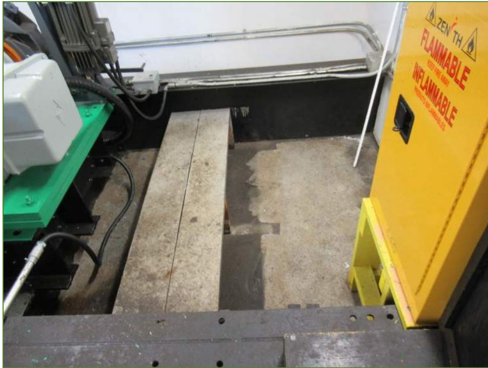
Photo P15 Machinery Room Slab (topside)
