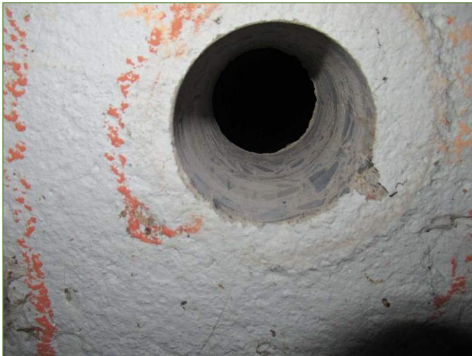
Photo P18 Typical Condition of Inside Core C2
