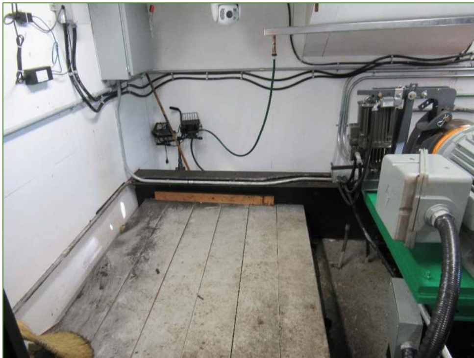
Photo P14 Machinery Room Slab (topside)
