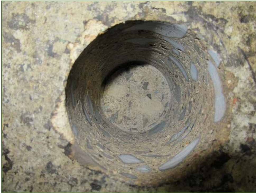
Photo P19 Typical Condition of Inside Core C5
