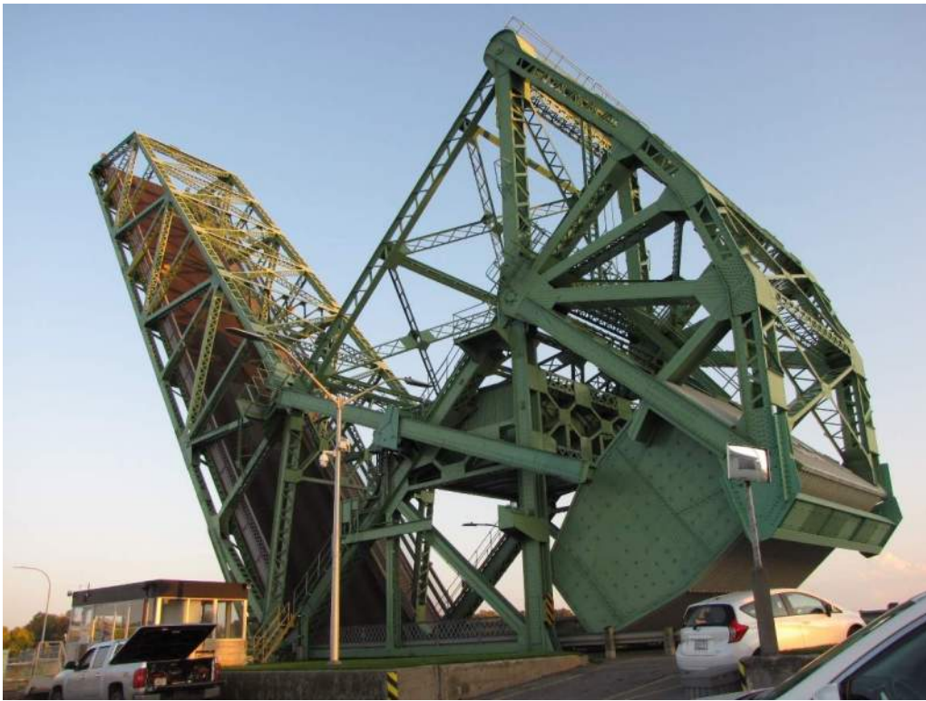
Photo S-4: Bridge in open position (photo from 2018 CDI).
