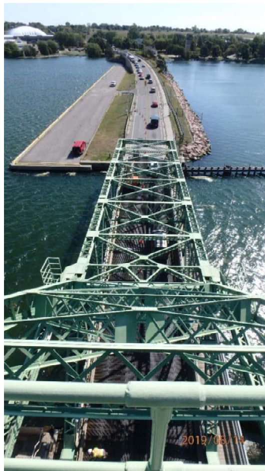
Photo S-3: Top of truss, looking east.
