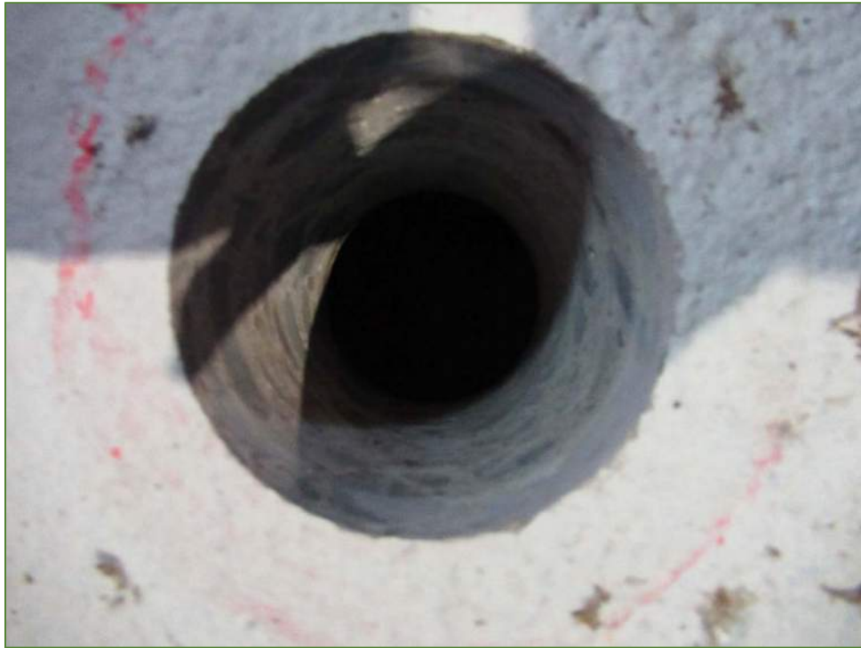
Photo P17 Typical Condition of Inside Core C1
