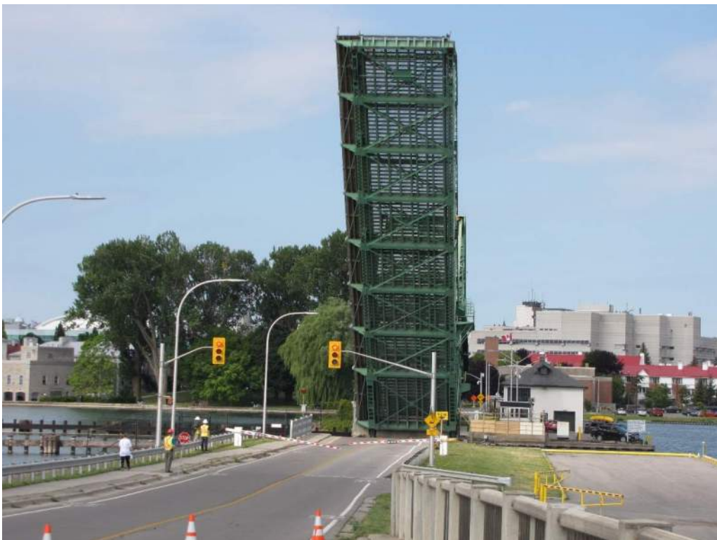
Photo S-5: Bridge in open position, looking east.
