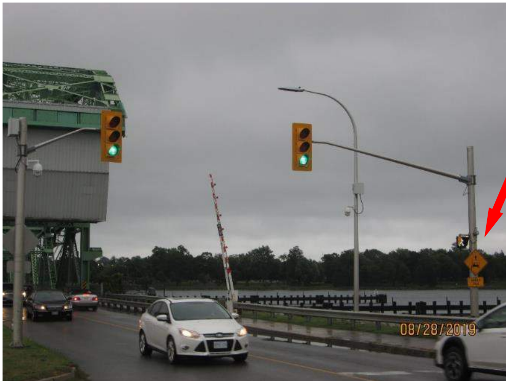
Photo E-25: Typical Traffic Signal (West Shown). Each bridge approach is provided with two sets of traffic signal fixtures mounted on cantilevered arms and suspended over the roadway. Additionally, a warning gong and a pedestrian signal light have been provided at each of the south traffic signal poles. The traffic signal equipment was installed as part of a recent rehabilitation project and is in very good condition. Note the east warning gong was not operational at the time of inspection.
