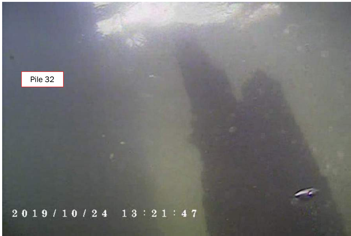
Photo S-115: Old, rotten, and unused pile ending just below the water surface at Pile 32 of the Bascule Bridge west fender wall.
