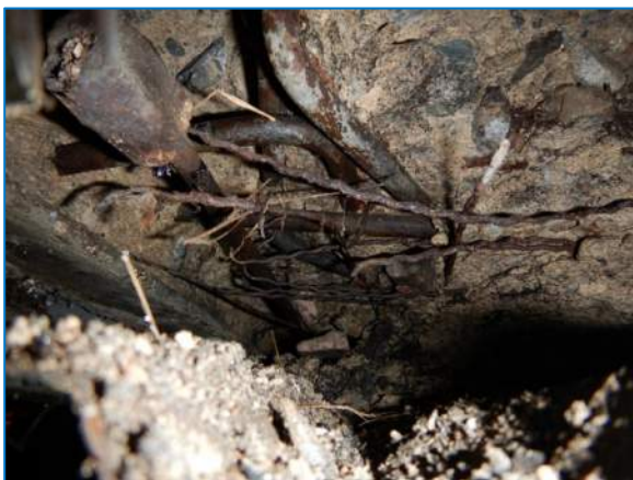
Photo 3 Soffit - South East Region
