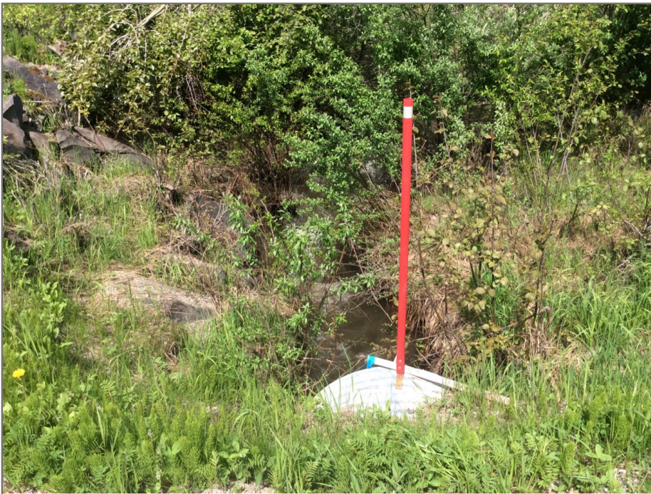
Photo 6: The view upstream of the KM 569.95 culvert.
