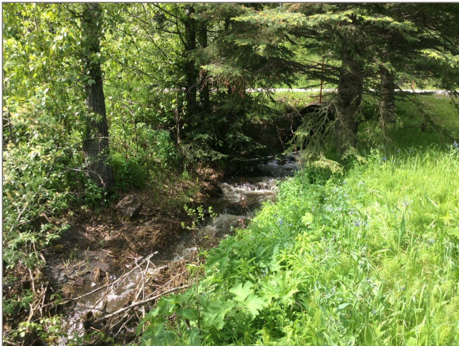
Photo 4: The view of the channel downstream of the KM 568.84 culvert.
