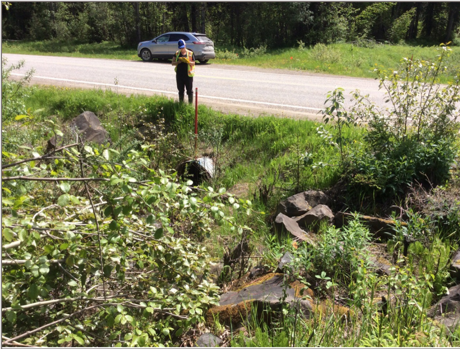
Photo 5: Inlet of the KM 569.95 culvert.
