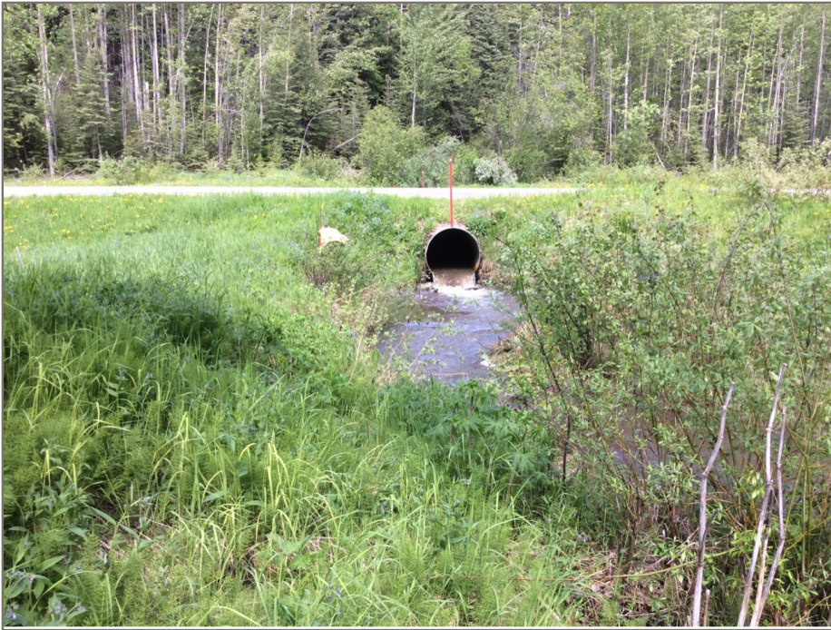
Photo 7: Culvert outlet at KM 569.95.
