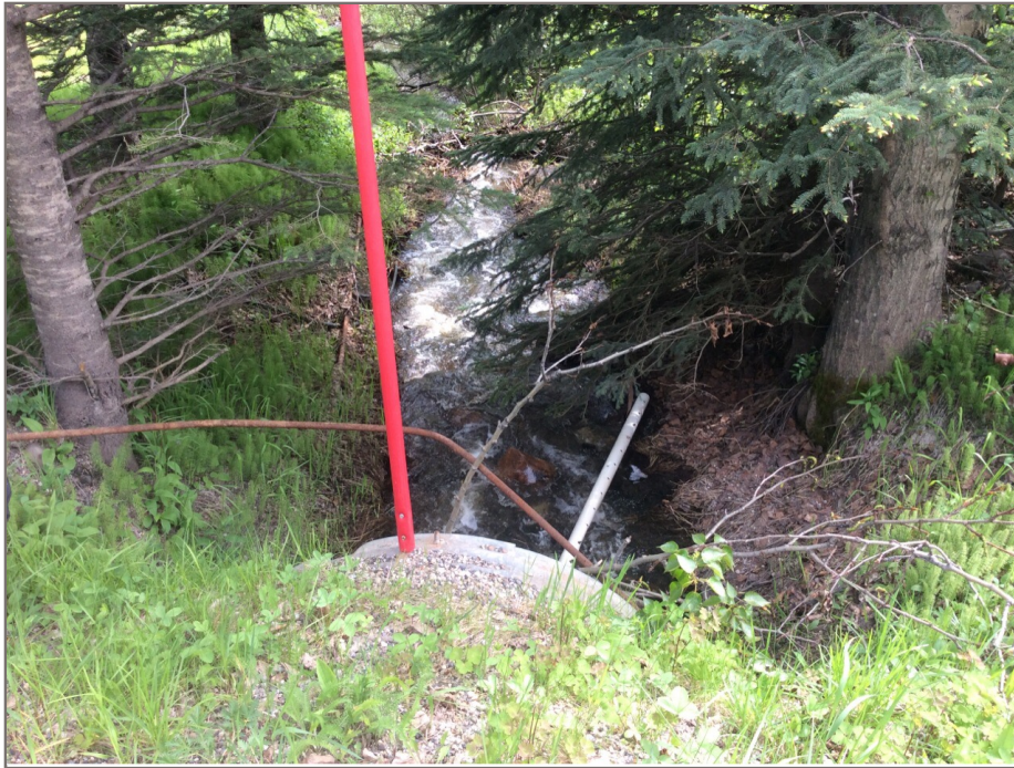
Photo 3: Culvert outlet at KM 568.84.
