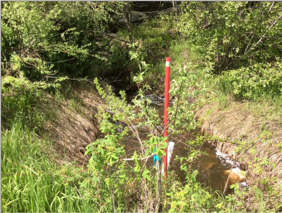
Photo 2: The view of the channel upstream of the KM 568.84 culvert.
