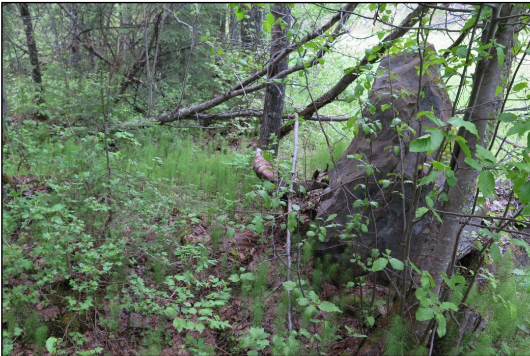
Photo 8: View NW showing rock debris and push along the tree line of the existing right-of-way
