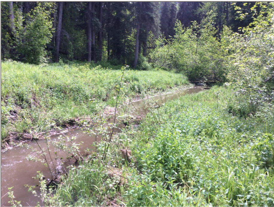
Photo 8: View of the downstream channel at the KM 569.95 culvert.
