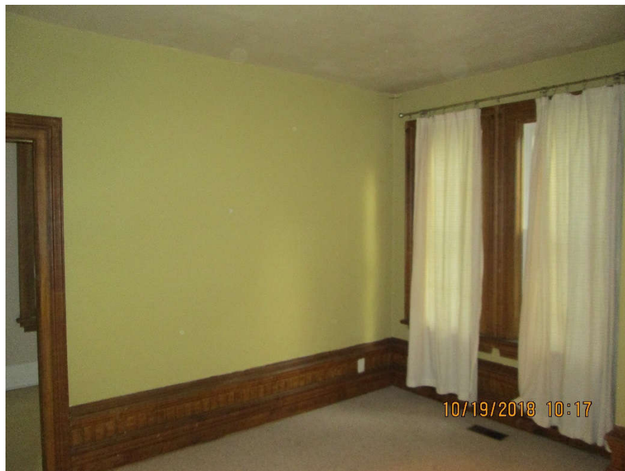
Photo 4: View of green lead-based paint (Sample 673155-P-05) on the wall of the study room of the dwelling.
