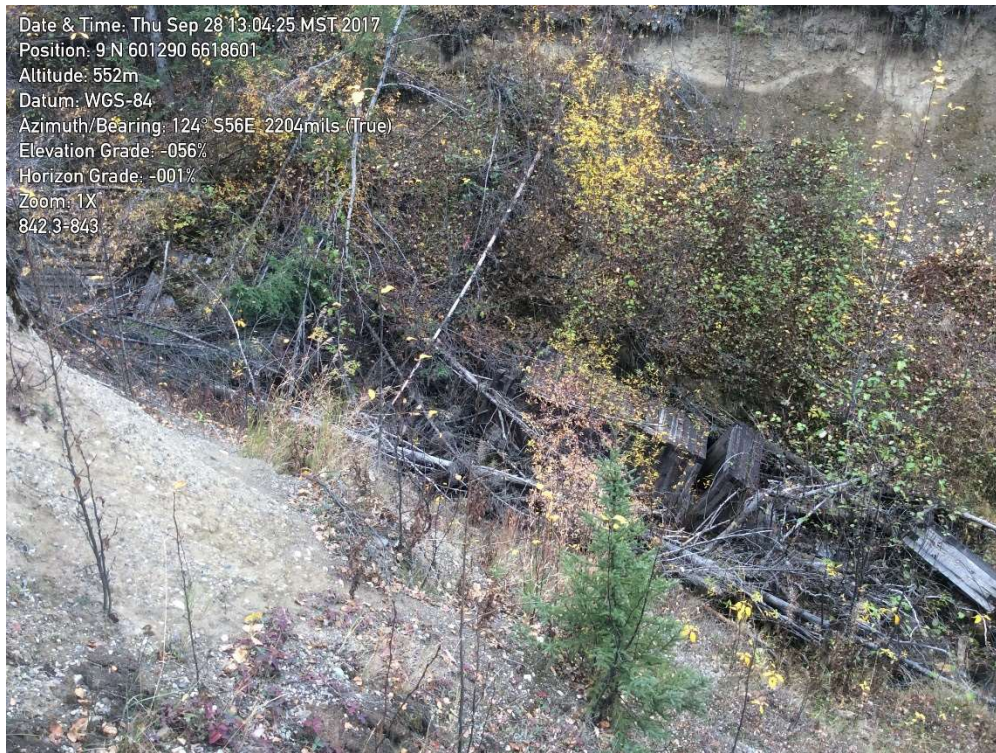
Photo 7: Site 2 (Km 841.95 to 844.40) – Timber Box Culvert - Photo 1 of 3
