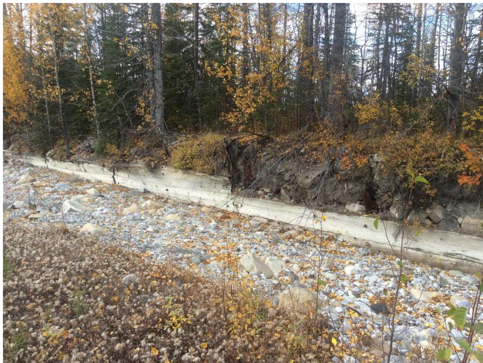
Photo 4: Site 1 (Km 612.70 to Km 481.50) – Timber Training Board - Photo 2 of 3
