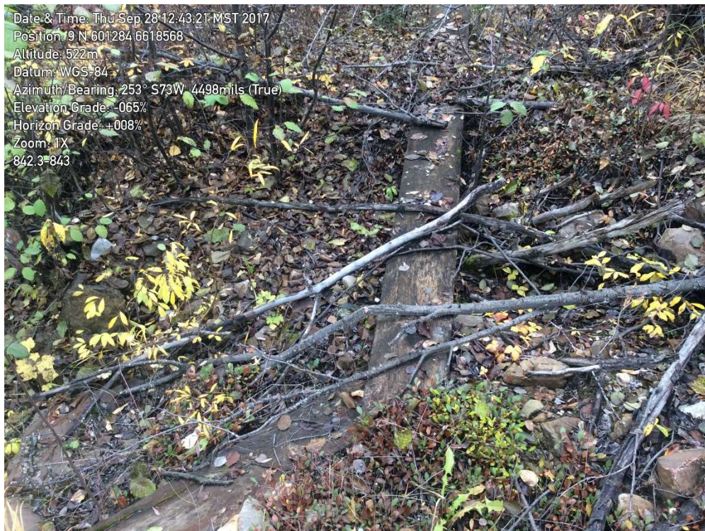
Photo 16: Site 2 (Km 841.95 to 844.40) – Debris downstream of box culvert - Photo 4 of 6
