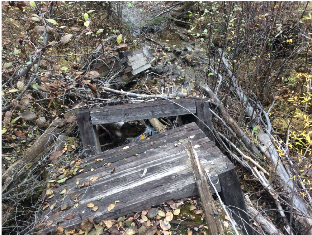
Photo 9: Site 2 (Km 841.95 to 844.40) – Timber Box Culvert - Photo 3 of 3
