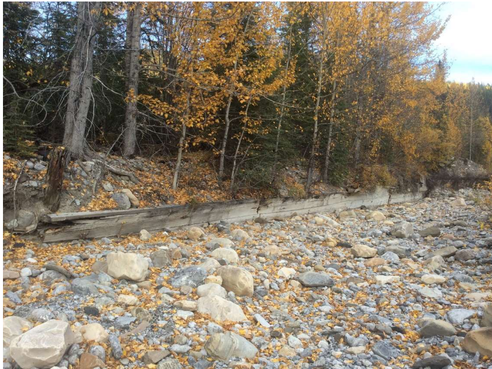
Photo 3: Site 1 (Km 612.70 to Km 481.50) – Timber Training Board - Photo 1 of 3
