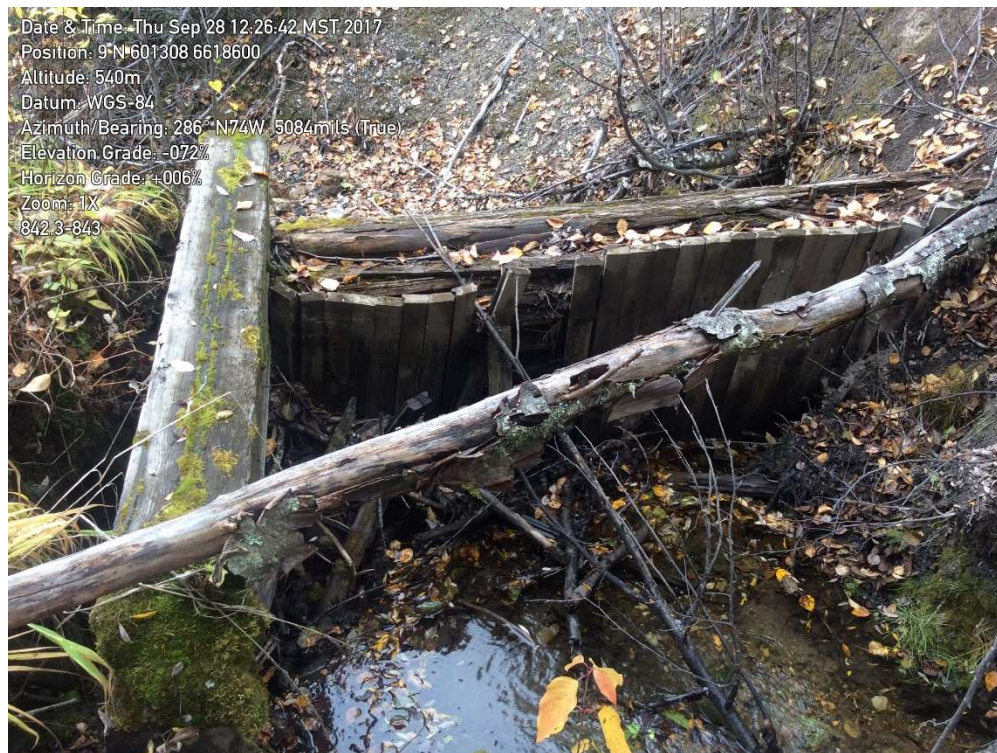
Photo 11: Site 2 (Km 841.95 to 844.40) – Timber Training Wall - Photo 1 of 1
