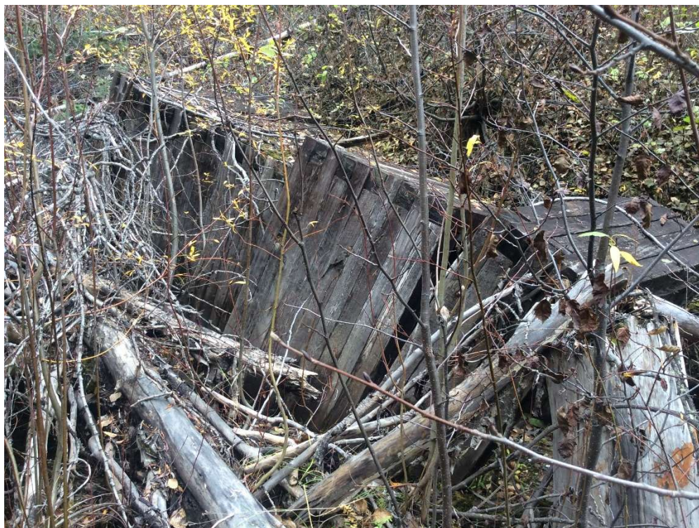
Photo 8: Site 2 (Km 841.95 to 844.40) – Timber Box Culvert - Photo 2 of 3
