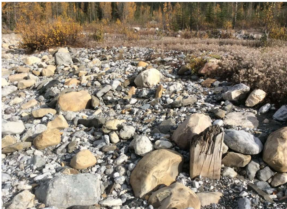
Photo 2: Site 1 (Km 612.70 to Km 481.50) - Timber Bridge Piles - Photo 2 of 2
