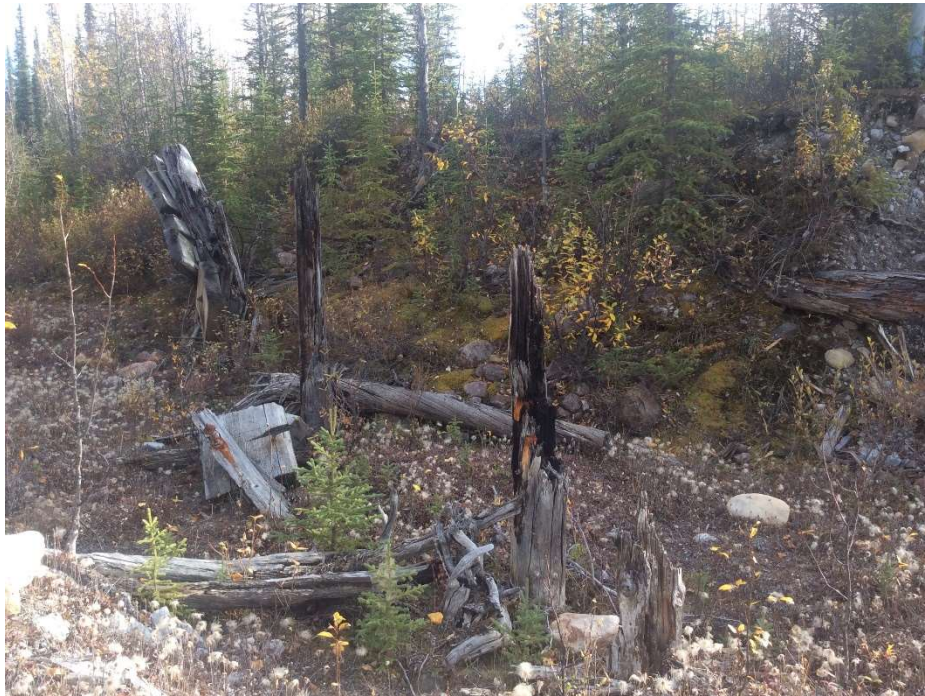
Photo 1: Site 1 (Km 612.70 to Km 481.50) – Timber Bridge Piles - Photo 1 of 2
