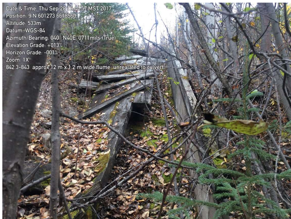
Photo 12: Site 2 (Km 841.95 to 844.40) – Timber Flume - Photo 1 of 1
