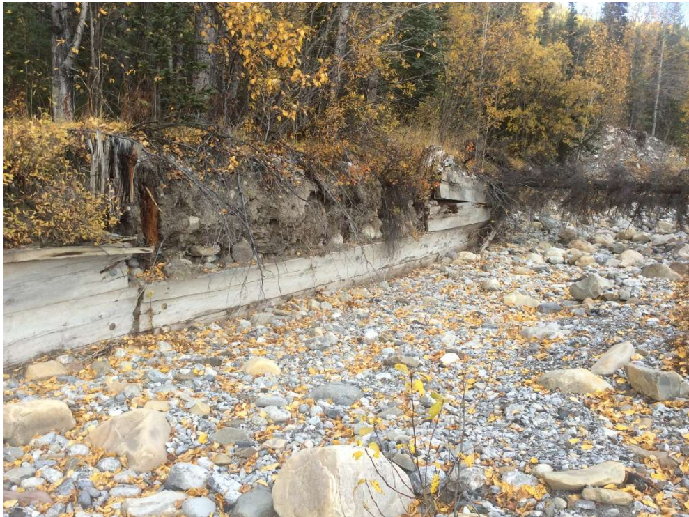
Photo 5: Site 1 (Km 612.70 to Km 481.50) – Timber Training Board - Photo 3 of 3
