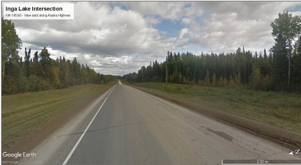
Photo 1: Inga Lake Intersection – View east along the Alaska Highway (Google Earth 2021).
