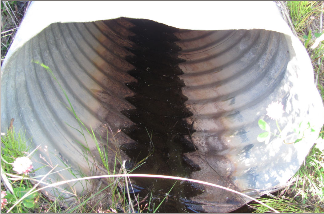
Photo 7: Low flows through the KM 145.30 culvert in 2011.
