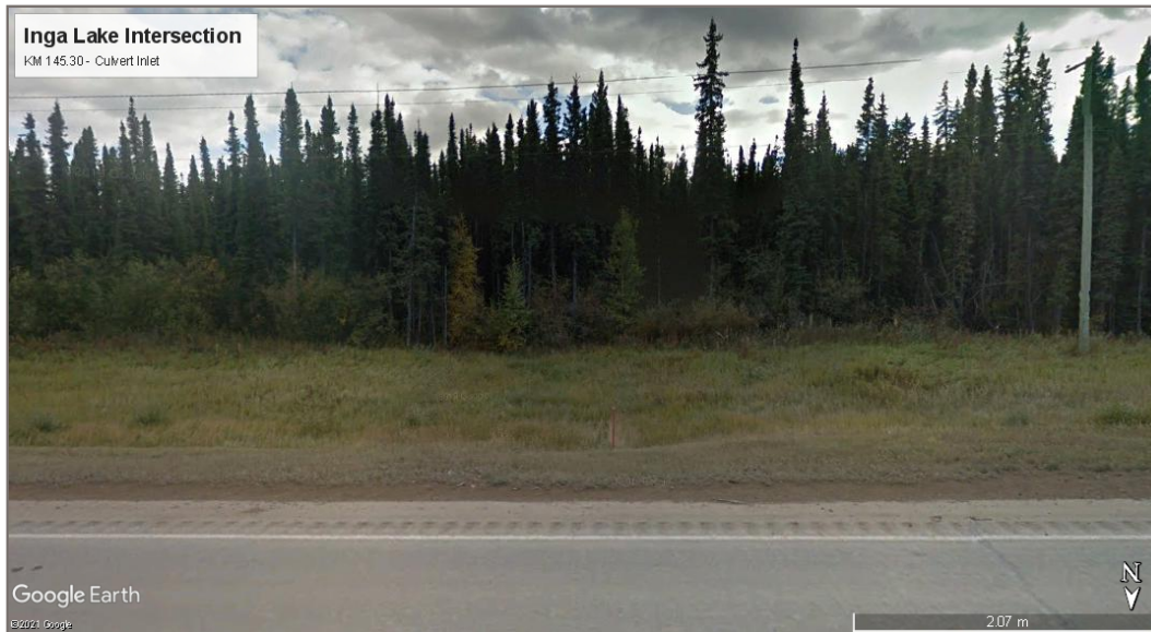
Photo 5: KM 145.30 Culvert Inlet / upstream – This culvert is located at the headwaters of a small 1 st order watercourse and will be undergoing a culvert extension (Google Earth 2021).
