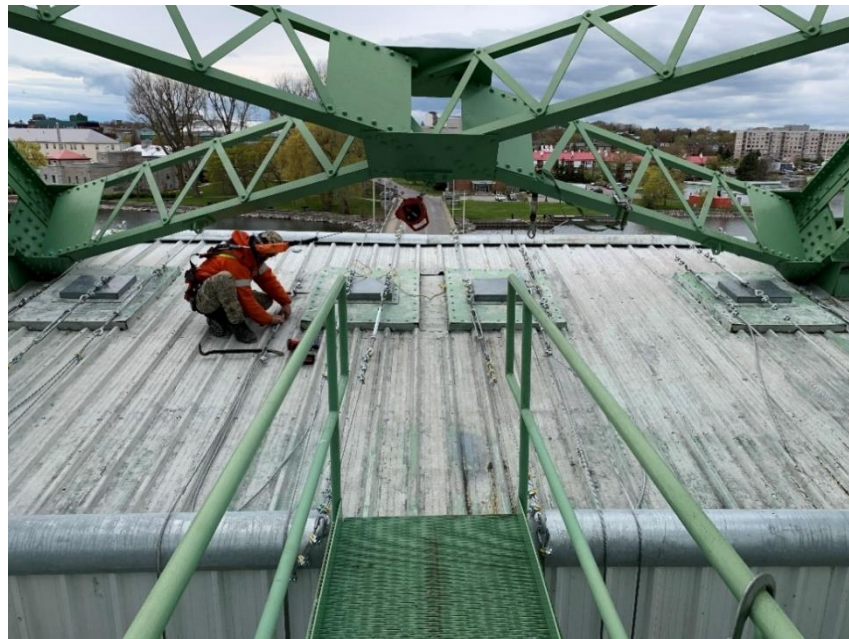
Figure 4: Installation of Wire Rope. Top Face Shown.
