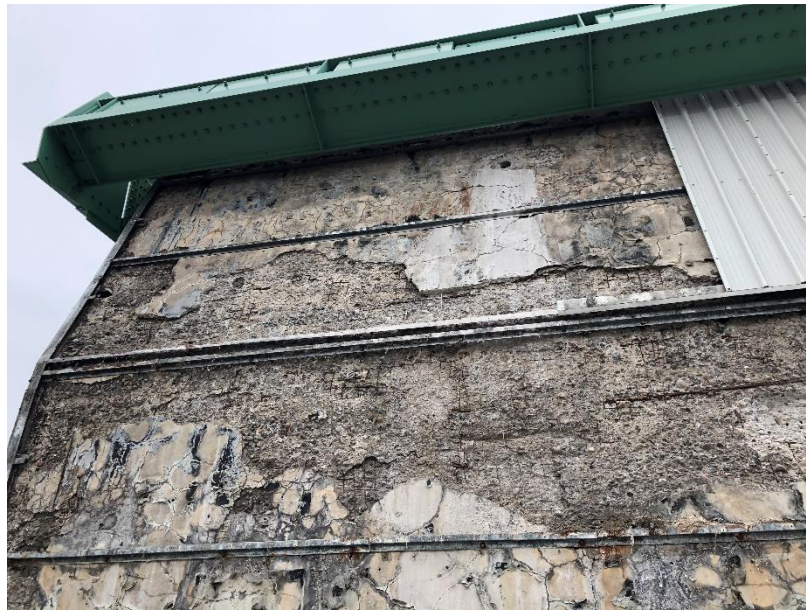
Figure 13: Cladding Support Steel – West Face Shown
