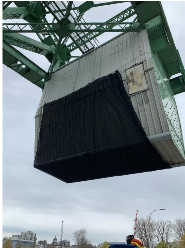
Figure 3: Installation of Debris Netting. East Face shown.
