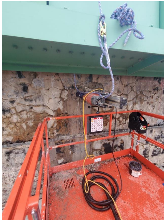
Figure 2: Concrete Core Removal in Progress on West Face.
