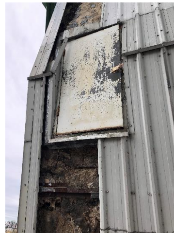
Figure 15: Steel Doors on East Face
