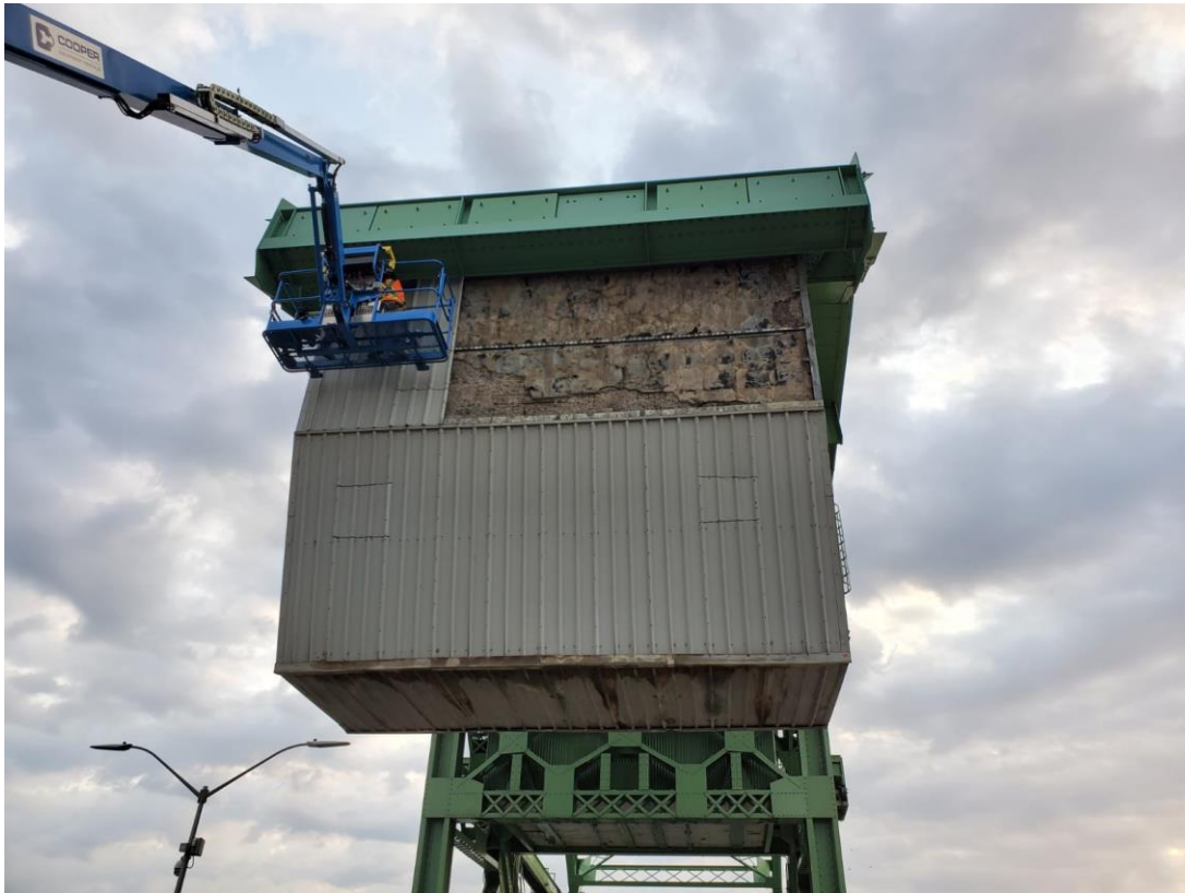
Figure 1: Counterweight Cladding Removal. West Face Shown.
