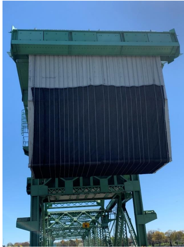
Figure 5: Completed Interim Repair. West Face Shown.
