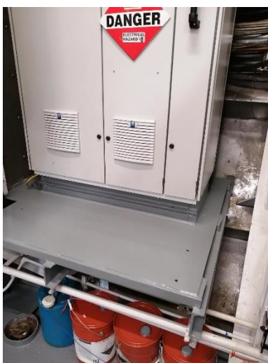
As fitted starboard ABB passive filter unit, seat and baseplate
