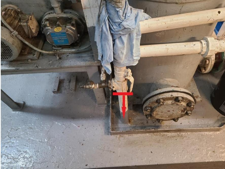
1.5 inch drain line through deck penetration
