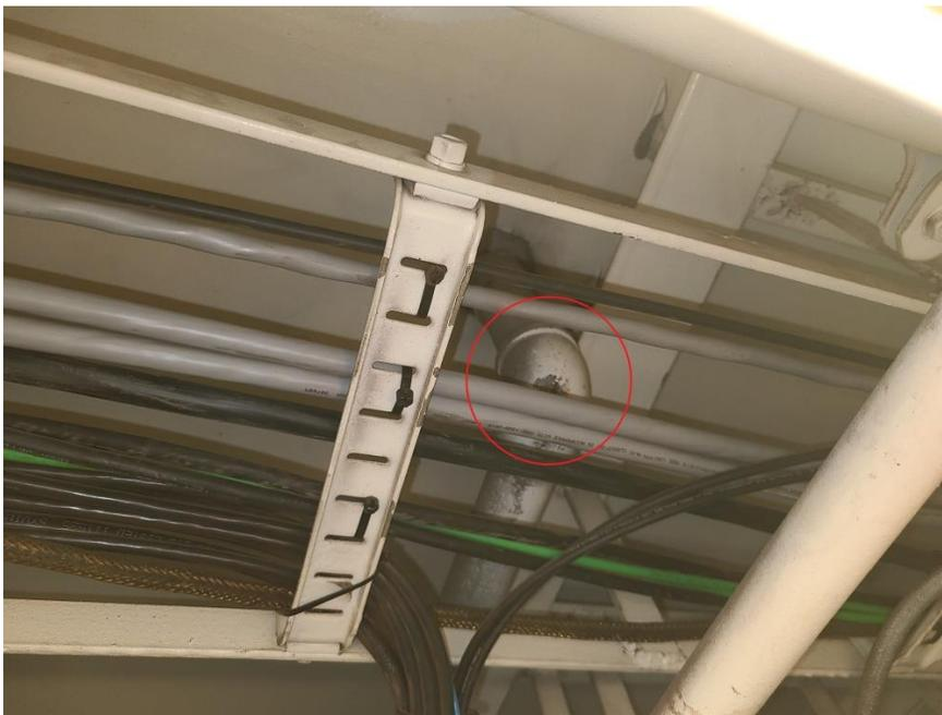
Other side of penetration in deck head. Located fwd of #2 main engine. Blockage is suspected to be in this section of pipe
