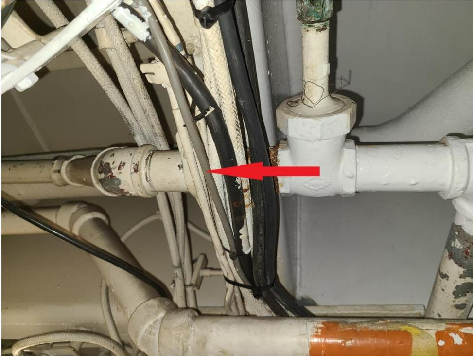
Line terminates above sewage transfer tank at 1.5 inch screw down valve. (arrow pointing to grey water drain line)
