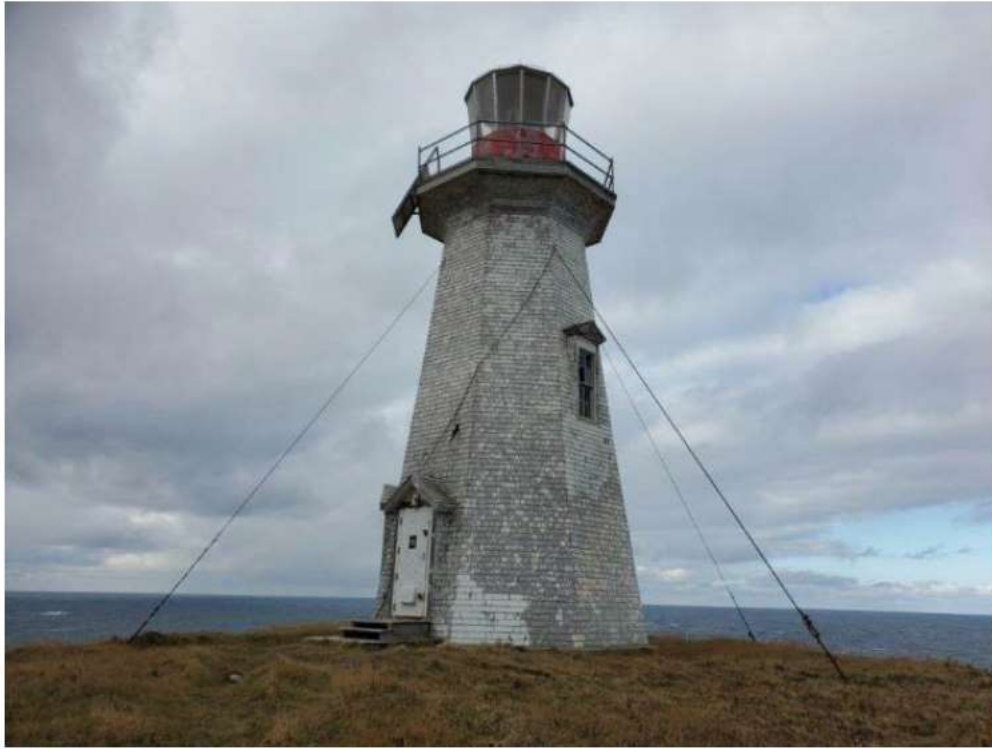
Figure 1: Photo of the Brion Island lighthouse
