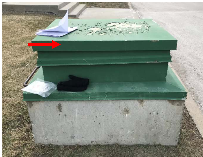
Photo 2. Green paint associated with Type C1 Hatches was confirmed to contain 195 ppm lead (DST Sample ID 1154-LP04).
