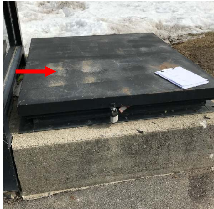
Photo 5. Manufactured black steel observed on Type H Hatch H3 is assumed to be lead-containing until bulk sampling and laboratory analysis prove otherwise. This paint could not be sampled without substrate interference.
