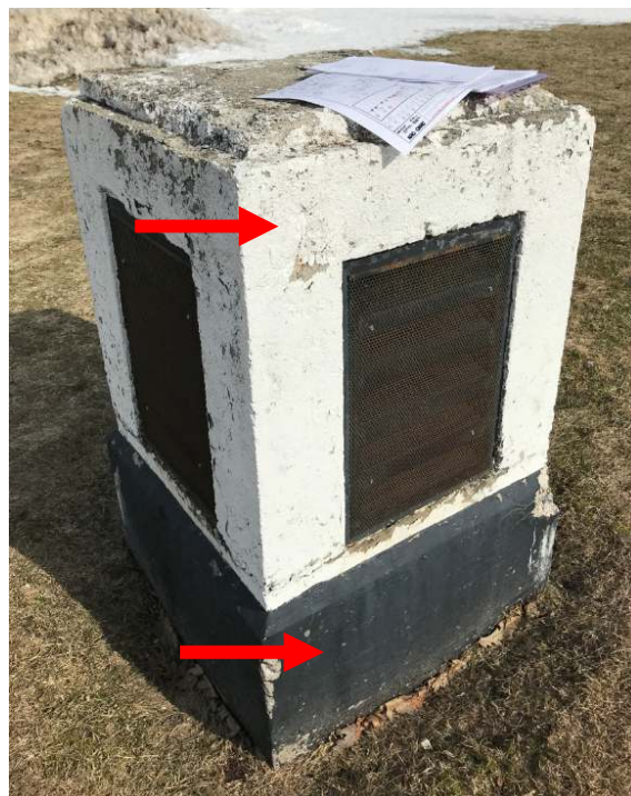
Photo 1. White paint associated with Type D Vents was confirmed to contain 622 ppm lead (DST Sample ID 1154-LP01). Black paint associated with Type D Vents was confirmed to contain 176 ppm lead (DST Sample ID 1154-LP02).
