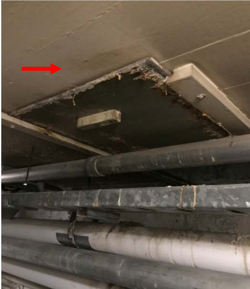
Photo 9. Grey ceiling paint within the tunnel under Type D Vent V2 was confirmed to contain 149 ppm lead (DST Sample ID 3603-LP02).
