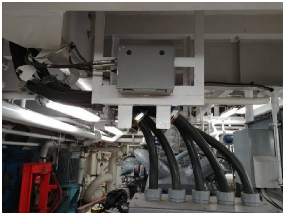
Photo 5 - DA1 – Power cable supports and platform
