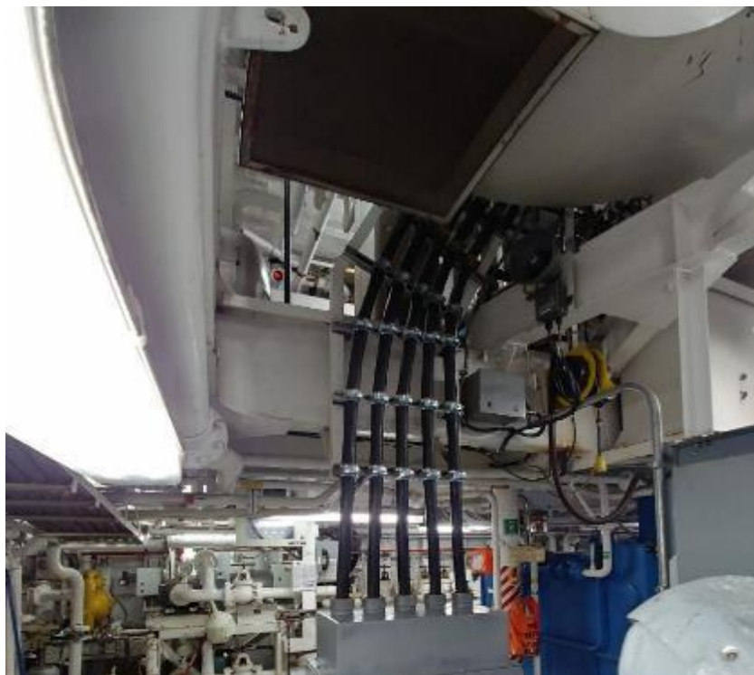
Photo 10 - DA3 – Power cable supports and lighting
