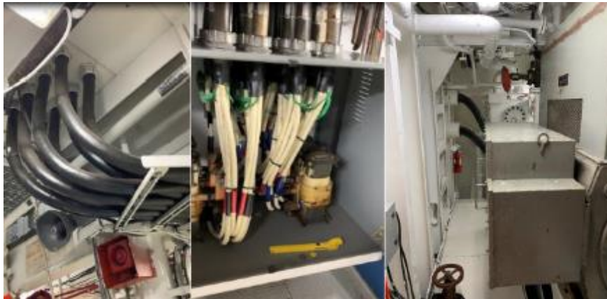
Motor Cabling from VFD, filter box, Forward E-motor
