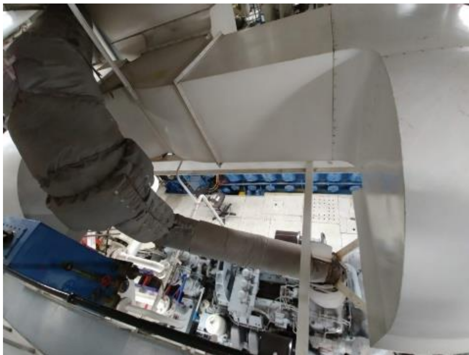
Photo 4 - DA1 – Ventilation ducts and exhaust pipe
