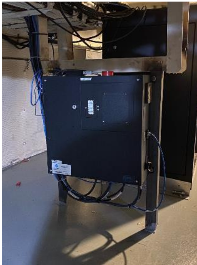
Figure 4 Existing SVDR Data Processing Unit to be removed and replaced with the new Data Acquisition Unit
