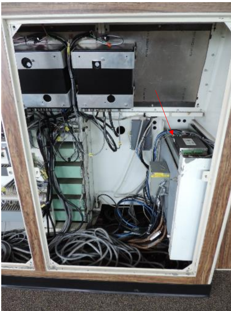
Figure 2 Existing NMEA Interface box to be removed
