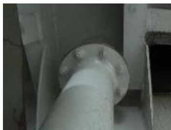
Photo 18 - Bolting to the ceiling
