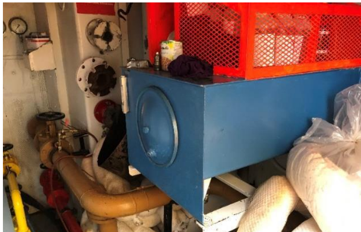
Forward Oil Header Tank (Station de Pompage Avant Valve Control Room)
