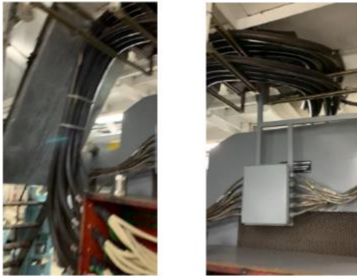
Motor Cabling from bottom of VFD cabinet (Propulsion Control Room) to Aft E- Motor Terminal Box (Propulsion Motor Room)
