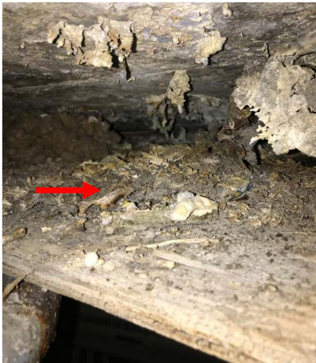
**Photo 7.** Miscellaneous debris observed on plywood within tunnels under the vents noted in Section 5.1.2 was confirmed non-asbestos containing (DST Sample ID 3603-01A-C to 08A-C).
