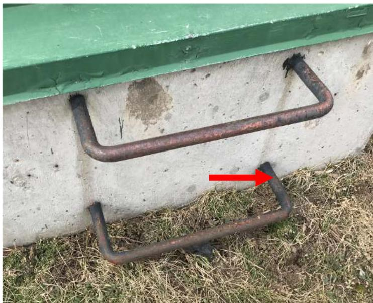
**Photo 3.** Black paint associated with the rebar on Type C1 Hatches was confirmed to contain 316 ppm lead (DST Sample ID 1154-LP05).
