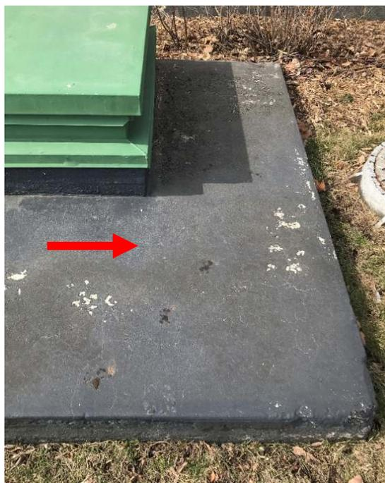
**Photo 6.** Black tar observed on the base of Type Q Hatch H11 was confirmed to contain 4.17% Chrysotile (DST Sample ID 1154-12A-C).
