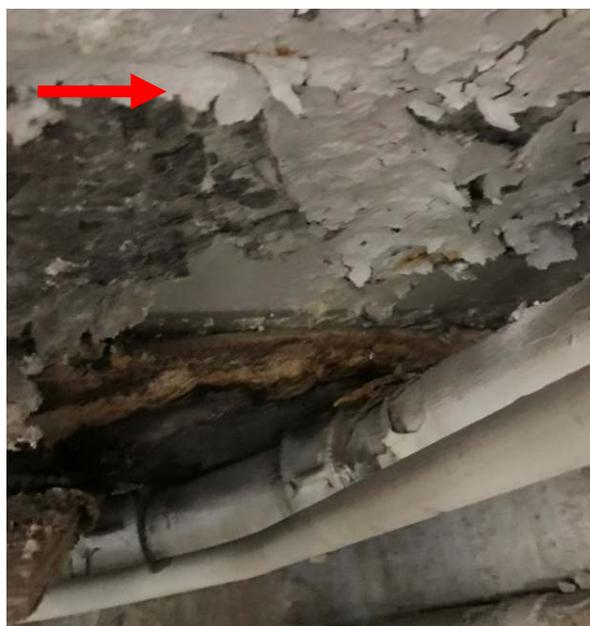
**Photo 8.** White ceiling paint within the tunnel under Type D Vent V1 was confirmed to contain 918 ppm lead (DST Sample ID 3603-LP01).
