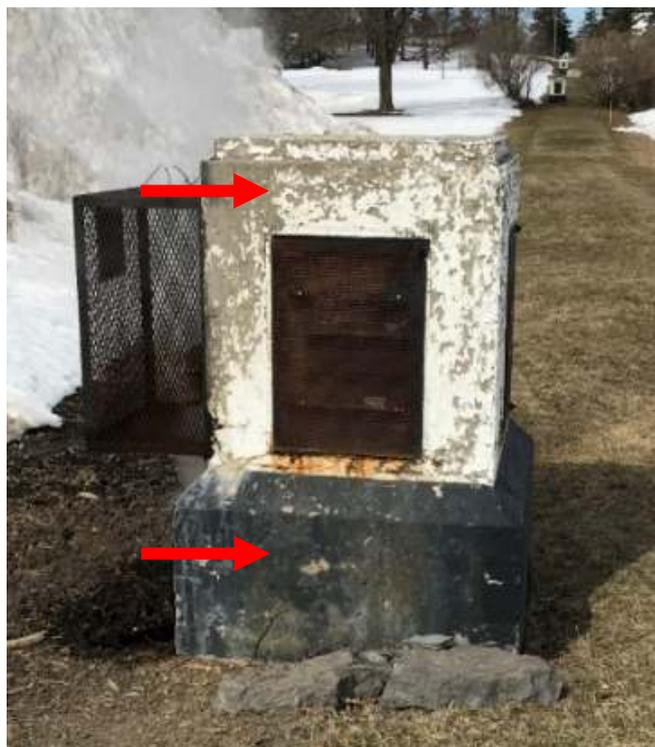
**Photo 4.** White paint associated with Type M Vents was confirmed to contain 5,710 ppm lead (DST Sample ID 1154-LP18). Black paint associated with Type M Vents was confirmed to contain 294 ppm lead (DST Sample ID 1154-LP19).
