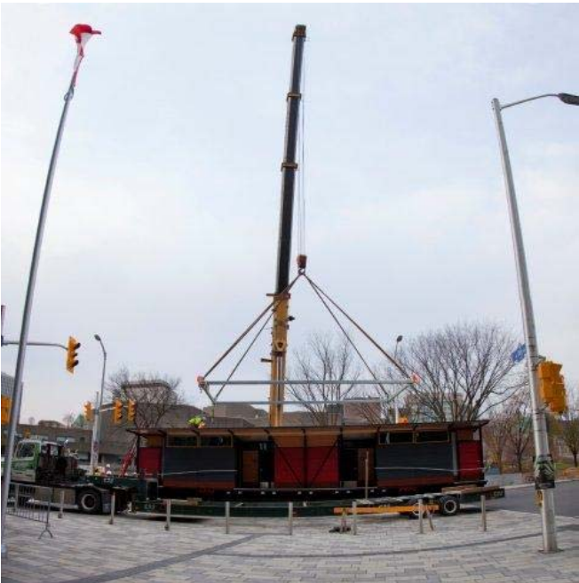
Picture illustration the lifting operation at Rideau Rest Area
