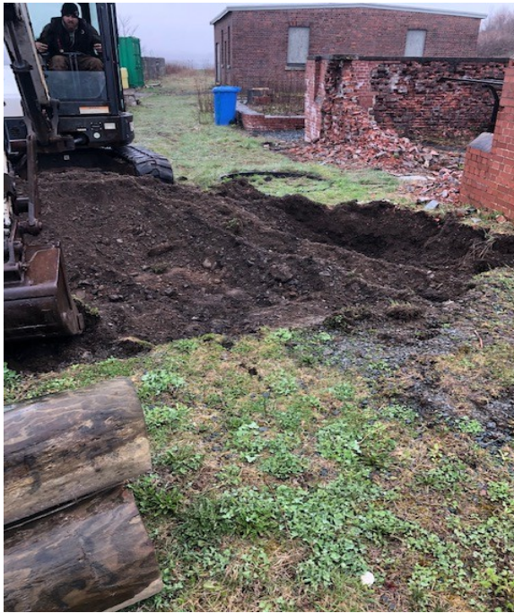
Photo 59 - Excavation from existing catch basin investigation on May 4, 2020. Excavator dug ~1m with no findings.
