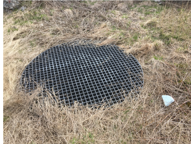
Photo 6 - Catch basin/well structure with steel grate between ruins.
