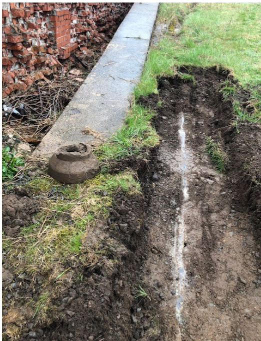
Photo 61 - Bottom of burried concrete swale was discovered during the excavation.
