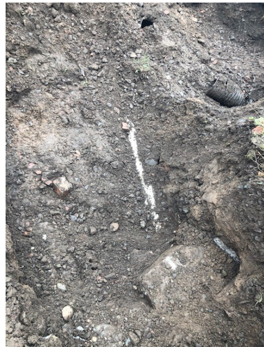
Photo 62 - Small PVC pipe (white) with wye connection as well as small corrugated pipe (black) discovered during the excavation.
